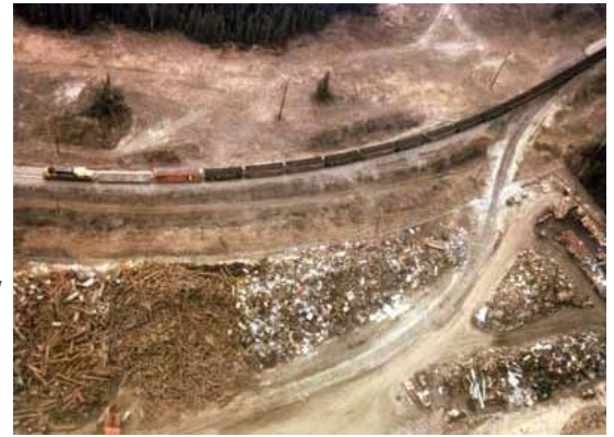
At the end of construction of the pipeline, scrap pipe, other metal and drums were stockpiled on Tax lot 201 for hauling south. Shown above the scrap piles is an Alaska Railroad train. The railroad tracks are at the southern boundary of the property. (DEC photo, late 1970s.)
