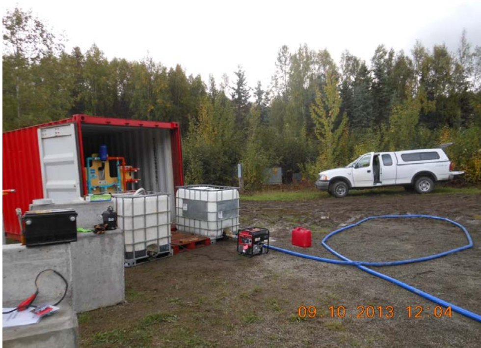
Photograph A-21: Injection system set up on site (September 2013)
