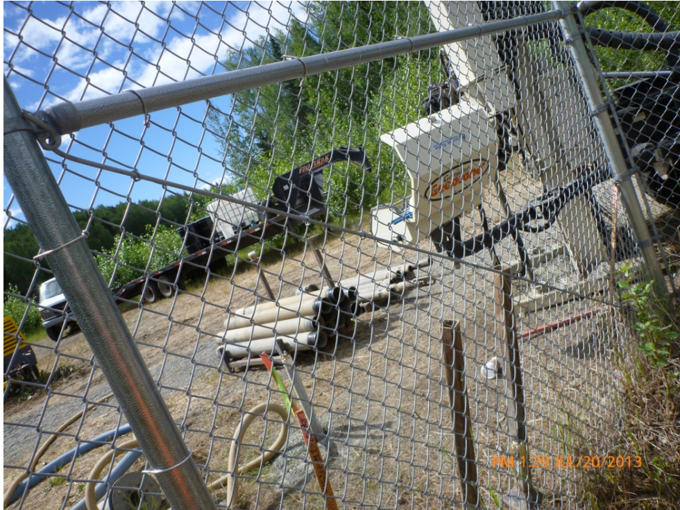
Photograph A-12: Air rotary equipped direct-push rig (July 2013)
