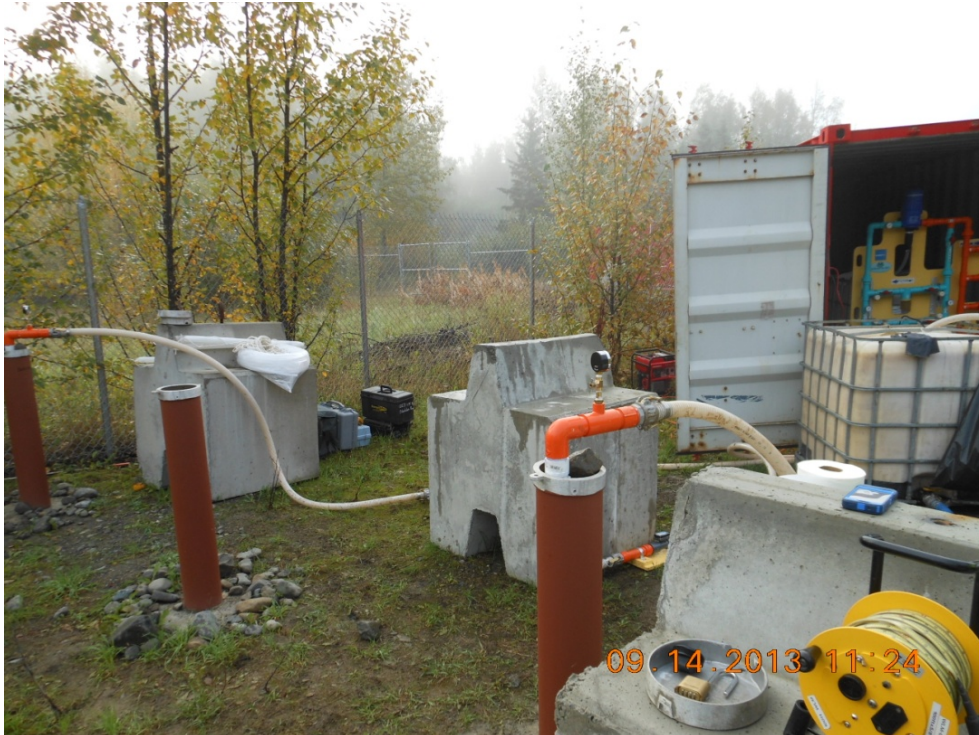
Photograph A-27: Injection at AP-3983 Target Treatment Zone (September 2013)
