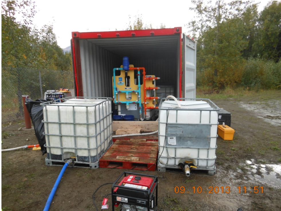
Photograph A-15: Injection at AP-4550 and AP-4551 Target Treatment Zones (September 2013)
