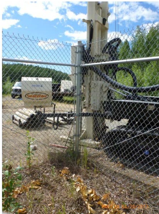
Photograph A-10: Air rotary equipped direct-push rig (July 2013)
