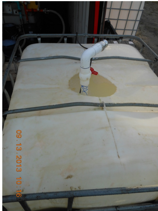
Photograph A-24: Injection batch mixing tank (September 2013)
