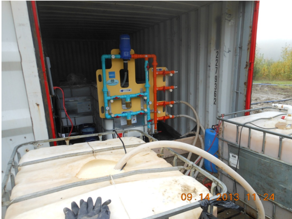
Photograph A-29: Batch injection at AP-3983 Target Treatment Zone (September 2013)
