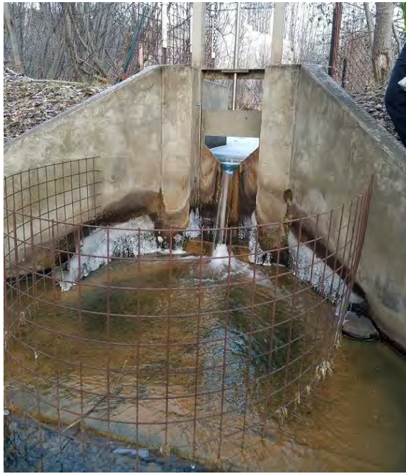
Photo A4-27 (SW): Site walk ST037-; Downstream of concrete weir (11/18/16)
