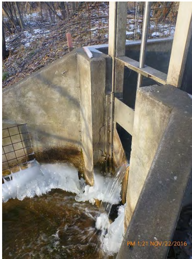
Photo A4-33 (NW): Sampling ST037-WCSW02; Concrete weir (11/22/16)
