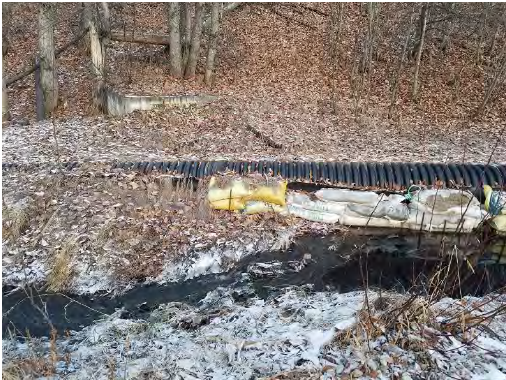
Photo A4-20 (NW): Site walk ST037-OU5SP-10; Stream to wetland (11/18/16)
