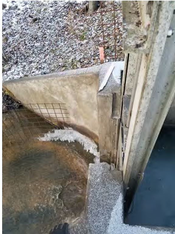
Photo A4-24 (W): Site walk ST037-WCSW02; Concrete weir (11/18/16)
