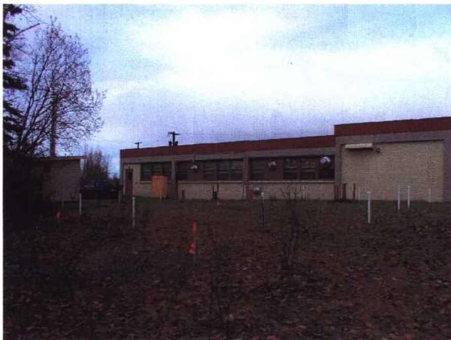
10/08/2003 – Backfilled and Cap of CB-12, CB-13, CB-14, and CB-15 on Southside of Building 986
