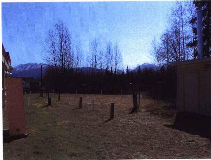
04/29/2003 – Gas Monitoring Points MP-1, MP-2, MP-3 South of Side Building 986
