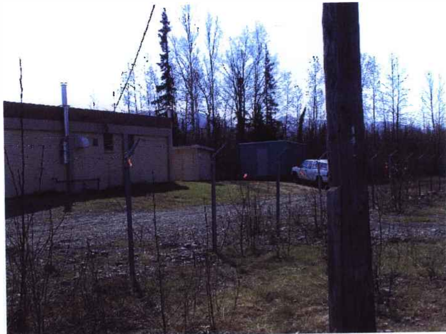
04/29/2003 – West View of Building 986, Power Pole and Blower House
