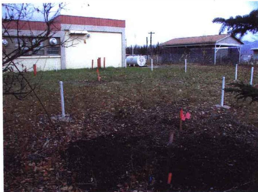
10/08/2003 – Backfilled and Cap of CB-12, CB-13, CB-14, and Building Heating Oil Storage on Southside of Building 986
