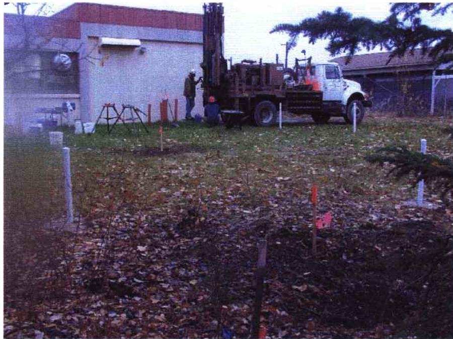
10/07/2003 – Soil Boring of CB-14 South- Southeast Corner of Building 986
