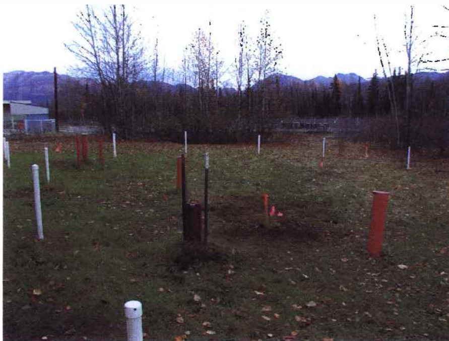
10/08/2003 – Backfilled and Cap of CB-15 on Southside of Building 986
