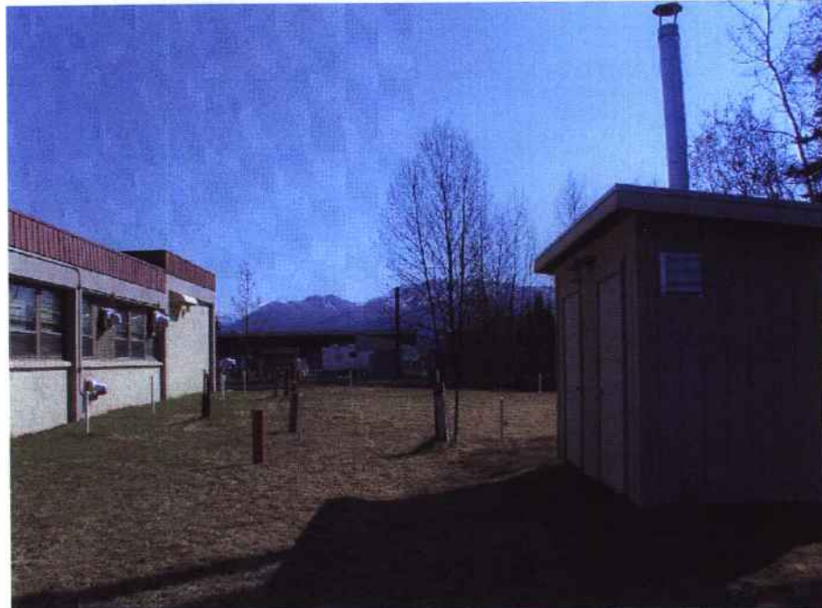
04/29/2003 – Blower Building and Vapor Extraction Piping South of Building 986
