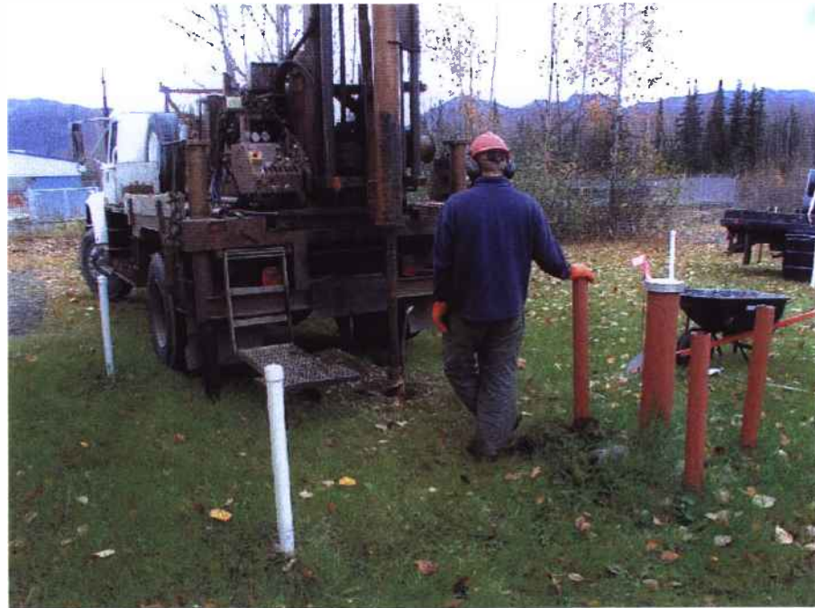
10/07/2003 – Boring of CB-14 on South-Southeast Corner of Building 986
