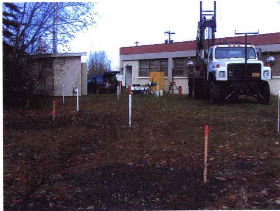
10/08/2003 - Boring of CB-15 on Southside of Building 986
