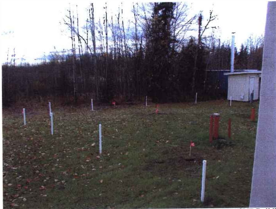
10/08/2003 – Backfilled and Cap of CB-12, CB-13, CB-14, CB-15, and BV/SVE Building for Vapor Extraction System on Southside of Building 986
