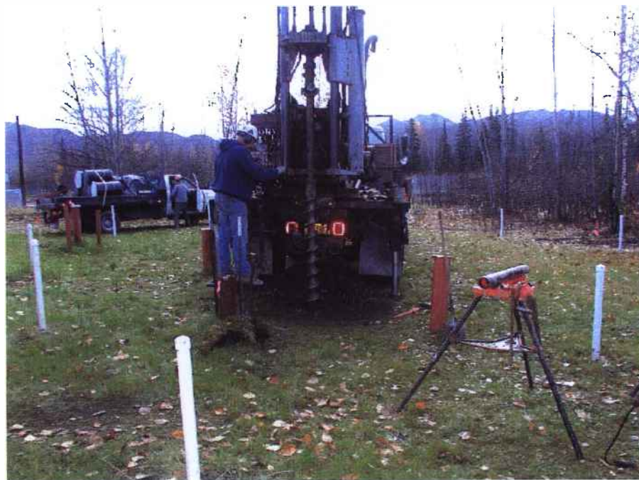
10/08/2003 - Boring of CB-15 on Southside of Building 986
