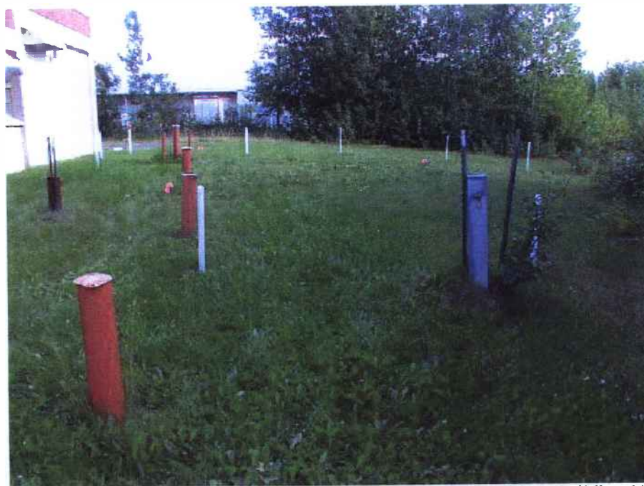
08/22/2003 – Gas Monitoring Points MP-1, MP-2, MP-3 South of Side Building 986
