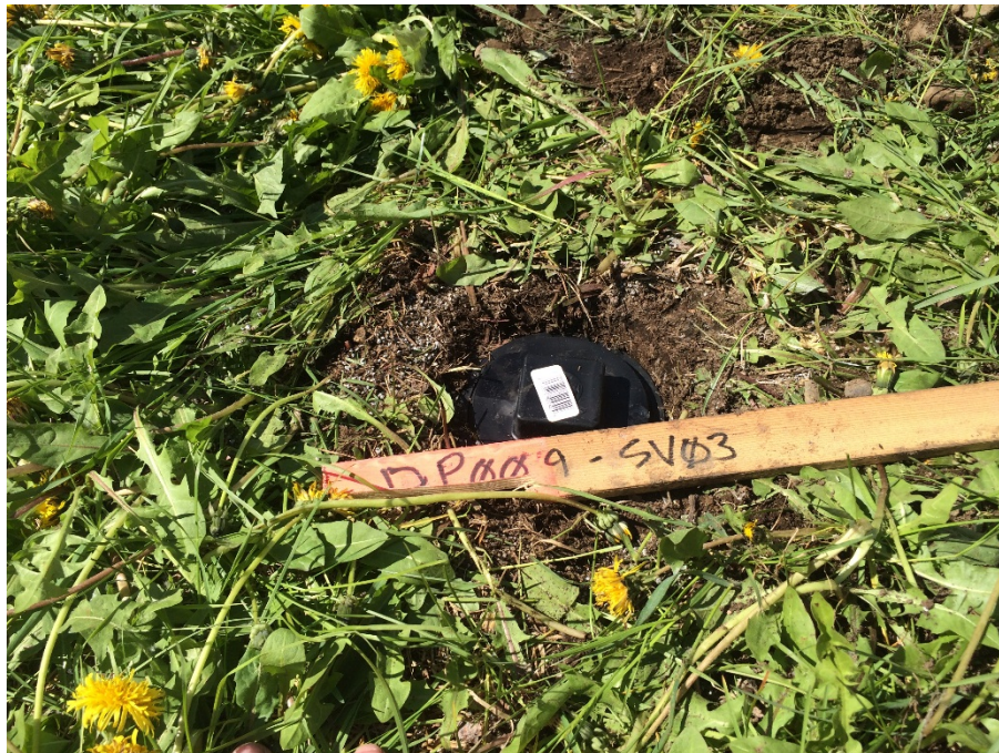
Photo A6-6: DP009-SV03, soil vapor probe monument after installation
