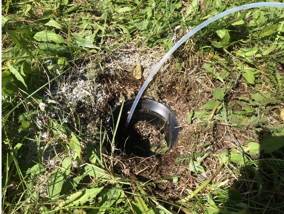
Photo A6-5: DP009-SV03, soil vapor probe after installation
