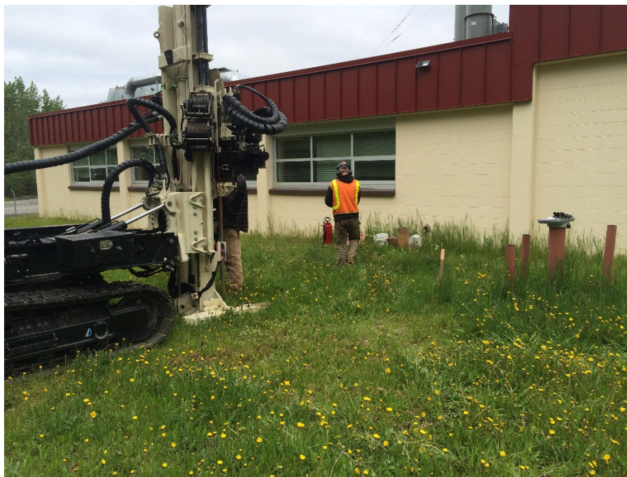
Photo A6-2: Installation of soil gas probe at DP009-SV03, NW view
