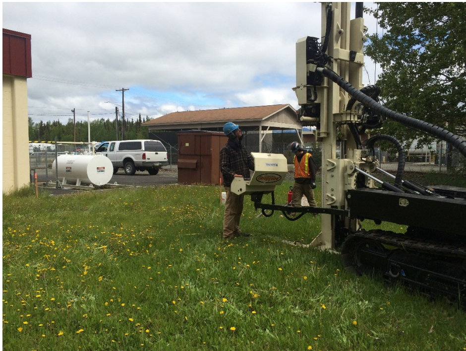
Photo A6-4: Installation of soil gas probe at DP009-SV05, E view
