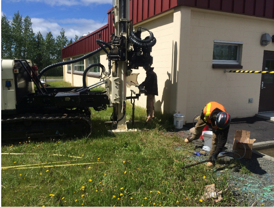
Photo A6-3: Installation of soil gas probe at DP009-SV04, W view
