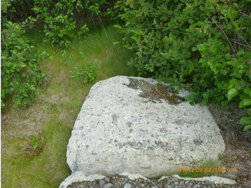
Photograph A5-17: Exposed transmitter annex concrete pad (July 2014).
