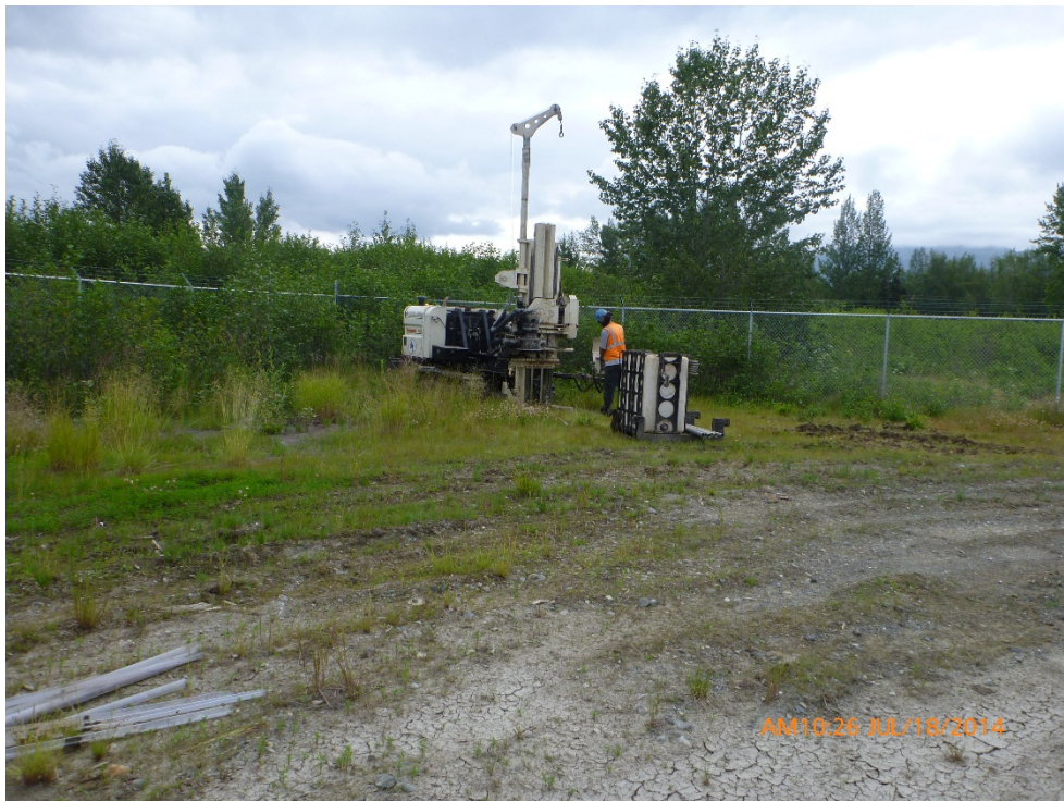
Photograph A5-6: SS041-SB02, 8040DT rig setup at SS041-SB02 facing North (July 2014).
