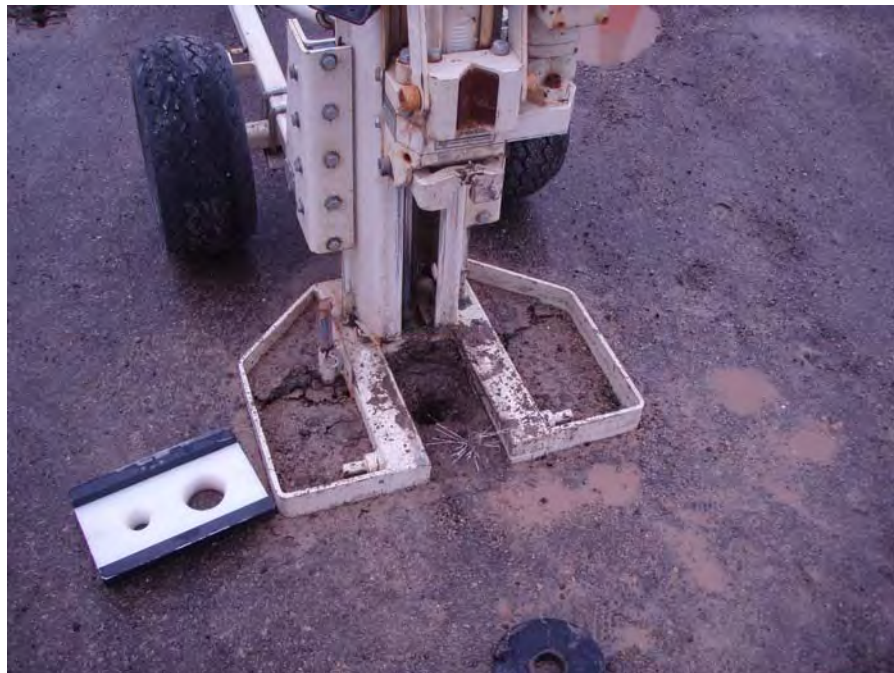
Photo No. 19 – 110924 Geoprobe® Operation
