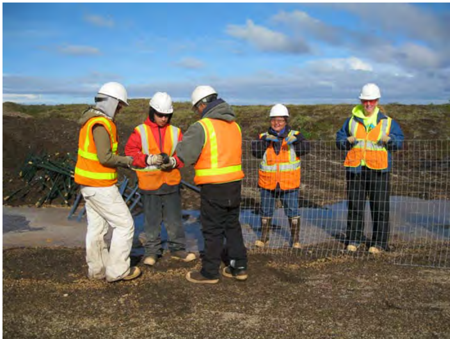
Photo No. 6 – 110827 Aniachak Workers Putting Up Fence in Storage Area 2, View North
