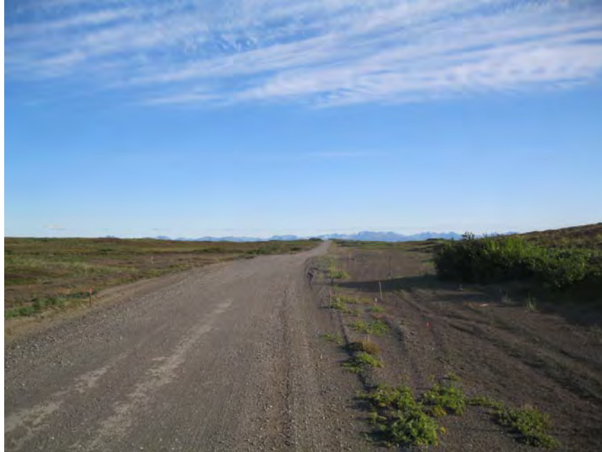
Photo No. 1 – 110816 View of Site Road to Southeast
