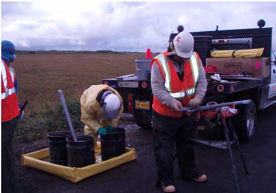
Photo No. 21 – 110924 Geoprobe® Decontamination and Operation, View East
