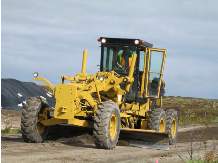
Photo No. 5 – 110827 Grading Site Road near Storage Area 1, View North
