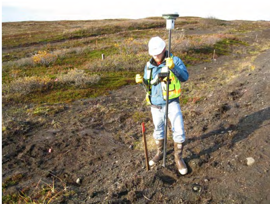
Photo No. 15 – 110915 Surveying Shoulder Profile, View Southwest
