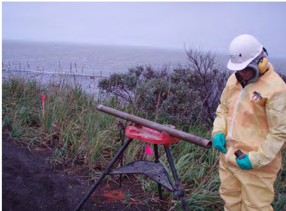
Photo No. 17 – 110924 Geoprobe® Tools, View West
