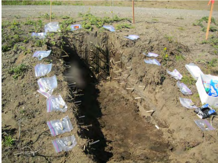
Photo No. 3 – 110817 Shoulder Profile Sampling Effort, View West
