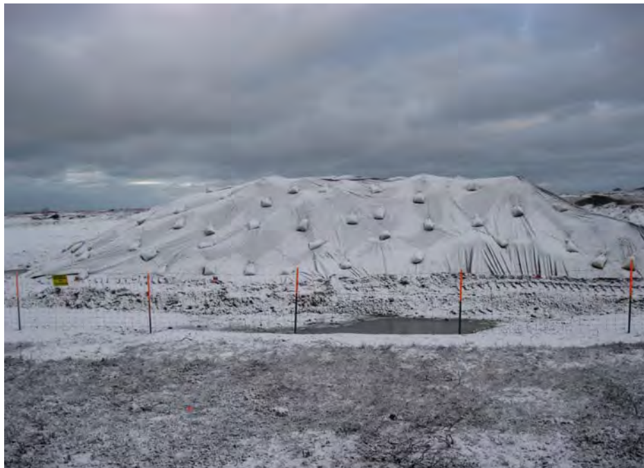
Photo No. 27 – 111031 Stockpile in Storage Area 1, View North
