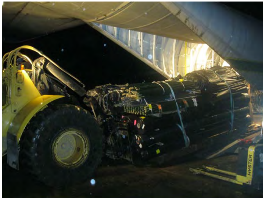
Photo No. 4 – 110818 Loader Unloading Liner from Hercules C130, View East.
