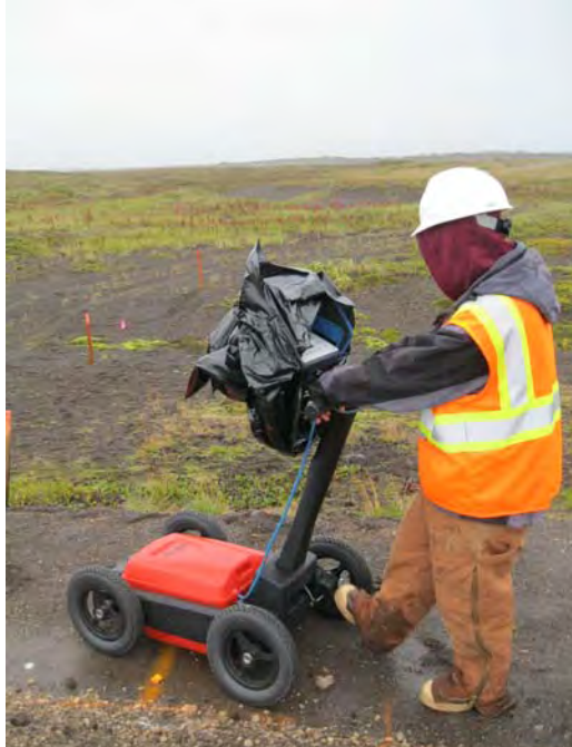
Photo No. 13 – 110913 Operating GPR, View East
