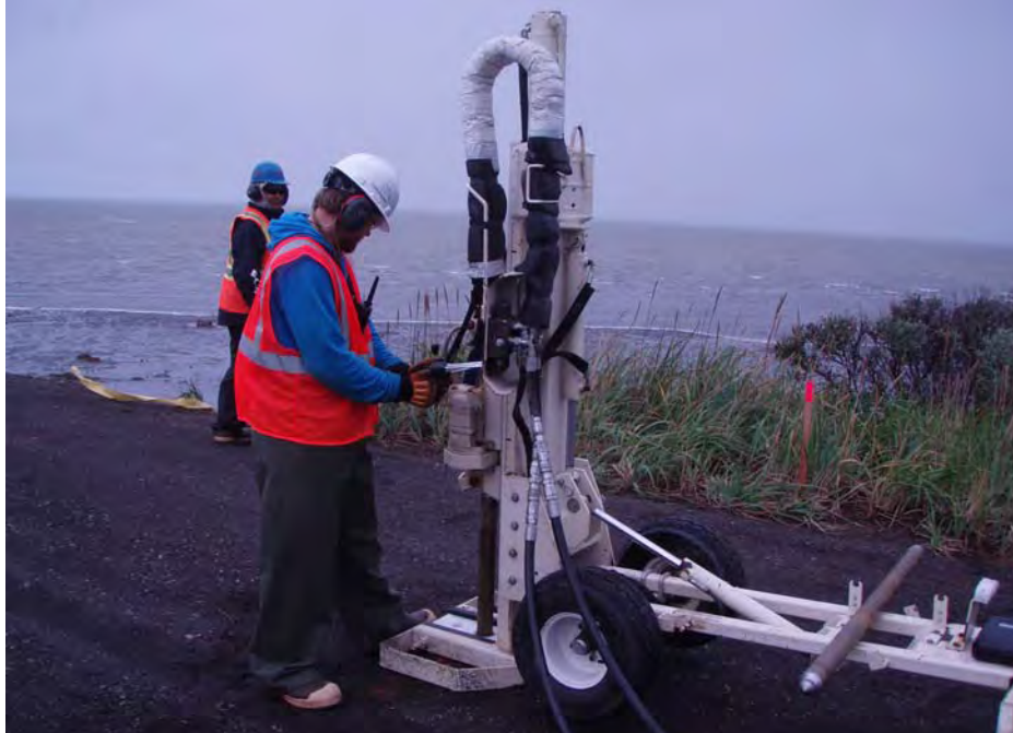
Photo No. 16 – 110924 Geoprobe® Investigation, View West
