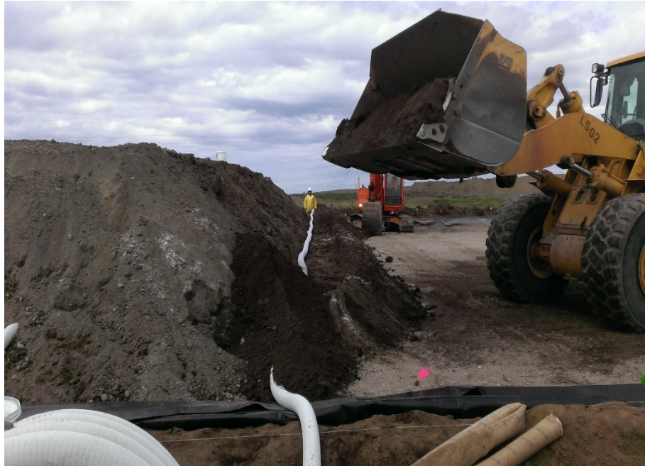
Photo No. 7 – 08 July 2014 Covering the second tier of ventilation piping in biopile. Facing north.
