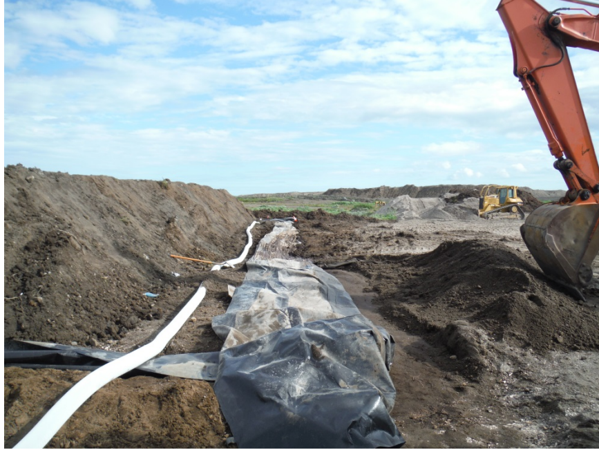
Photo No. 11 – 15 July 2014 Filling Biopile BSA. Facing east.
