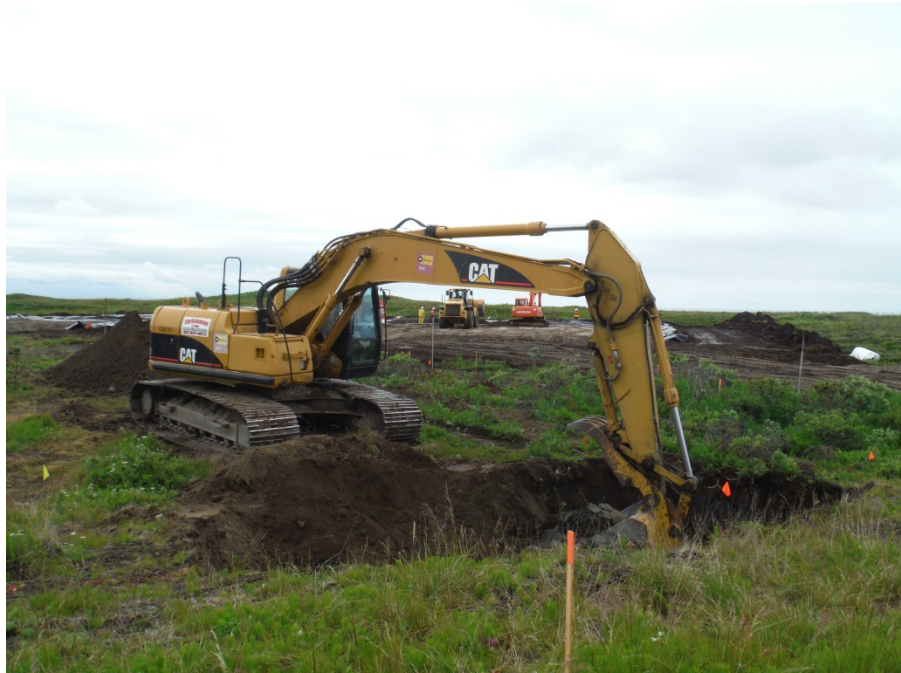
Photo No. 5 – 07 July 2014 Excavating the PCE-contaminated soil for the biopiles. Facing west.
