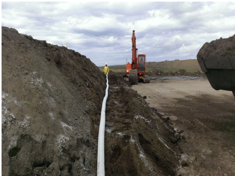
Photo No. 6 – 08 July 2014 Installing the second tier of ventilation piping in biopile. Facing north.
