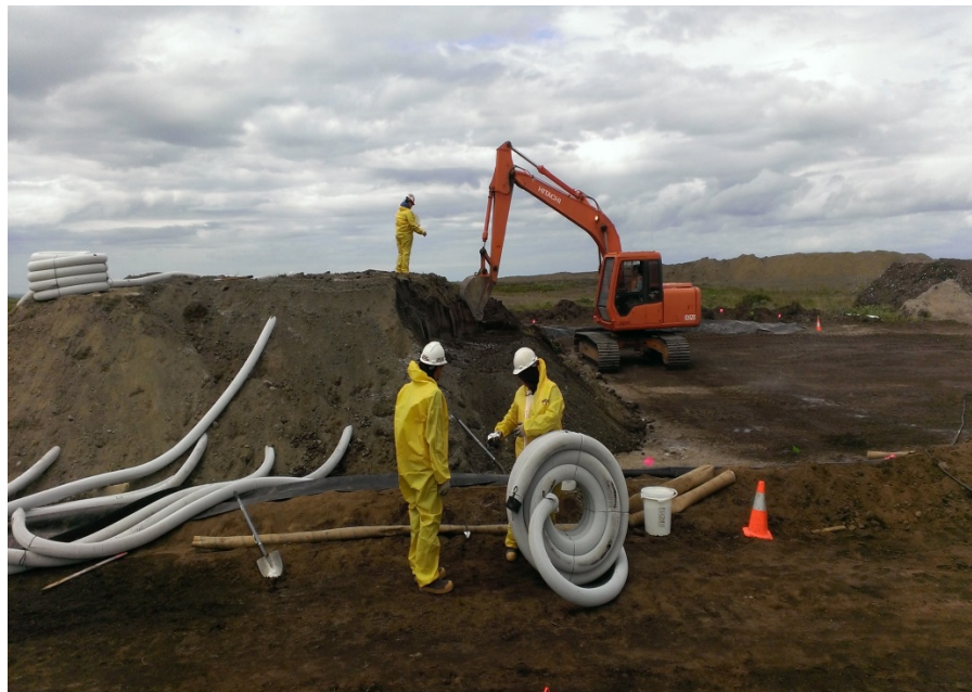
Photo No. 8 – 08 July 2014 Prepping biopile for third tier of piping. Facing north.
