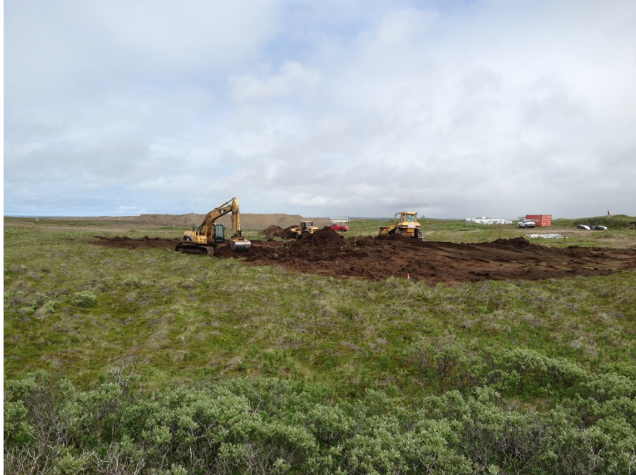
Photo No. 1 – 30 June 2014 Clearing the pads for the biopiles. Facing west.
