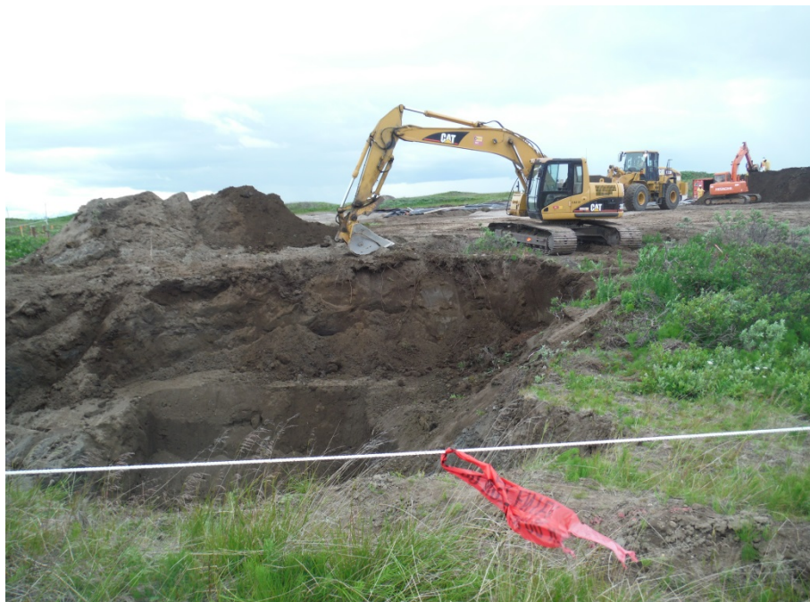
Photo No. 10 – 12 July 2014 PCE-contaminated soil excavation. Facing west.
