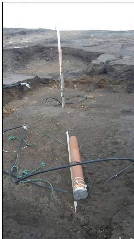
Photograph 5. Monitoring well PG-1 at the former RRS. October 14, 2016; view to the north.
