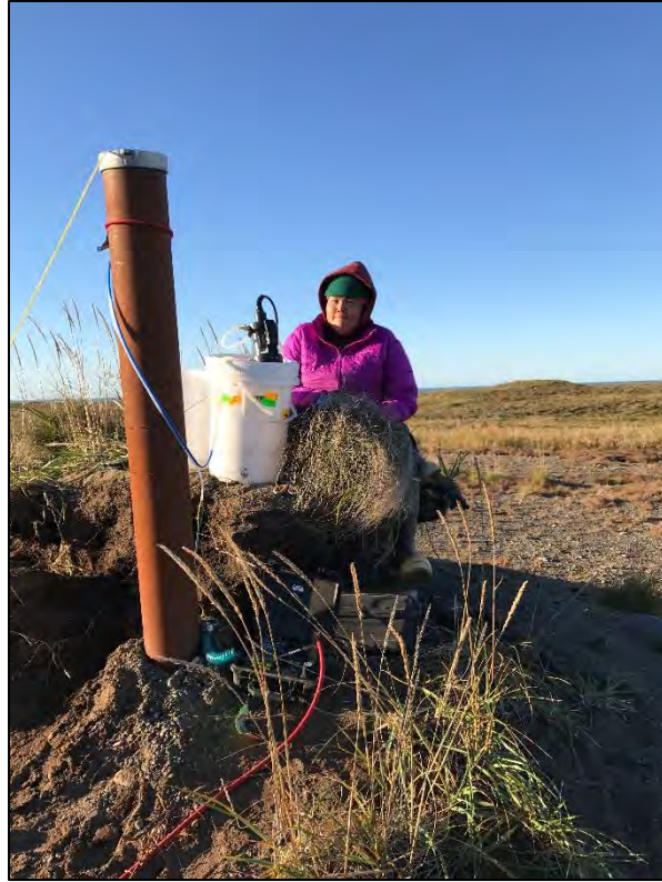
Photograph 3. GLO-MW-03. The well is in good condition, however, the ground around the well is eroding away. View to the north-northeast. September 30, 2017.
