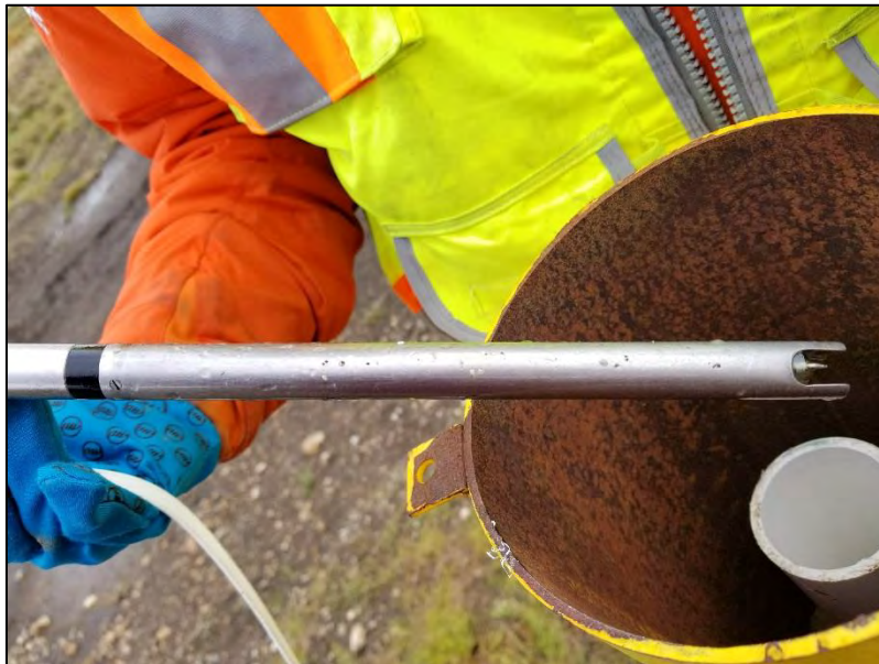
Photograph 4. BLO-MW-01, top of well. Petroleum residue on probe. This well had been damaged and repaired by another contractor in the summer of 2017. September 27, 2017.
