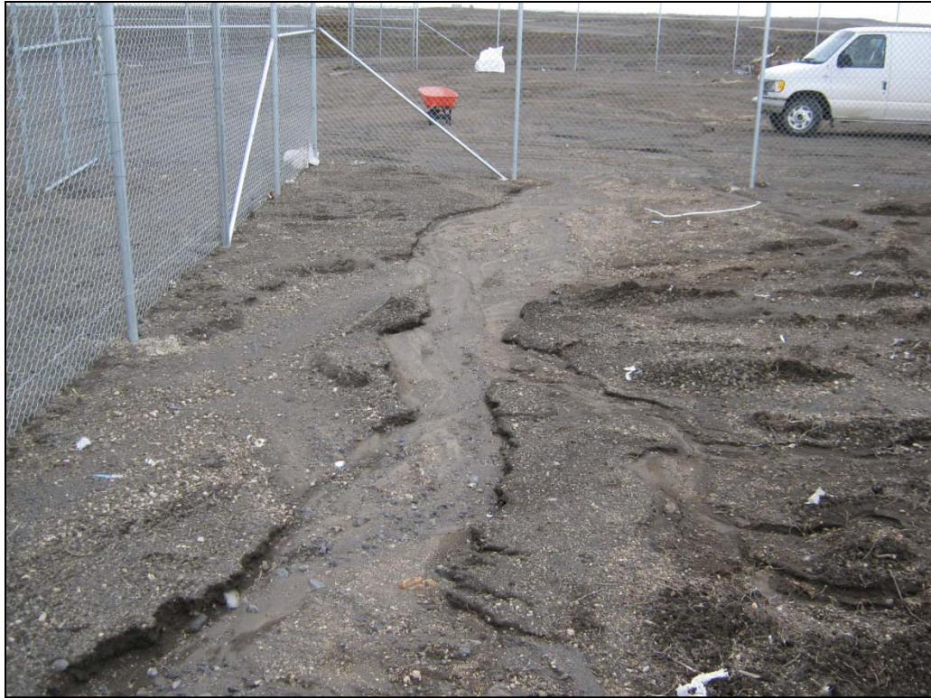
Photo 13. Landfill Erosion
