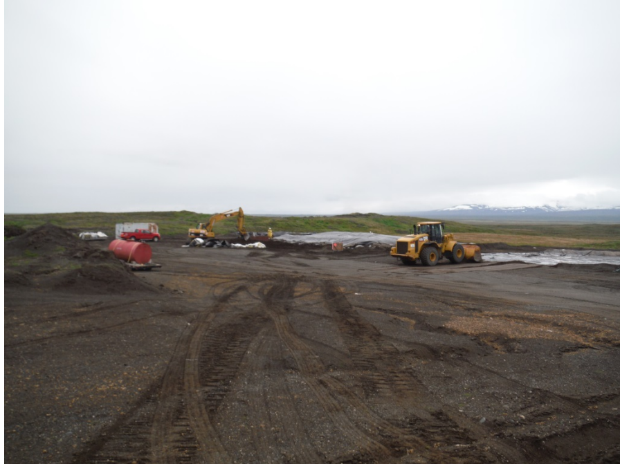
Photo No. 17 – 12 June 2014
