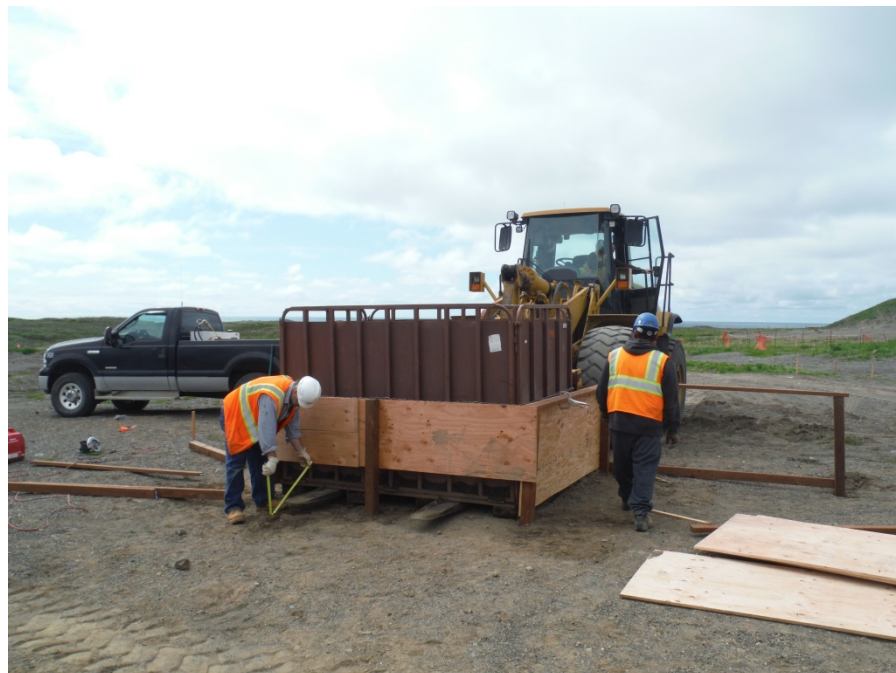
Photo No. 20 – 16 June 2014
