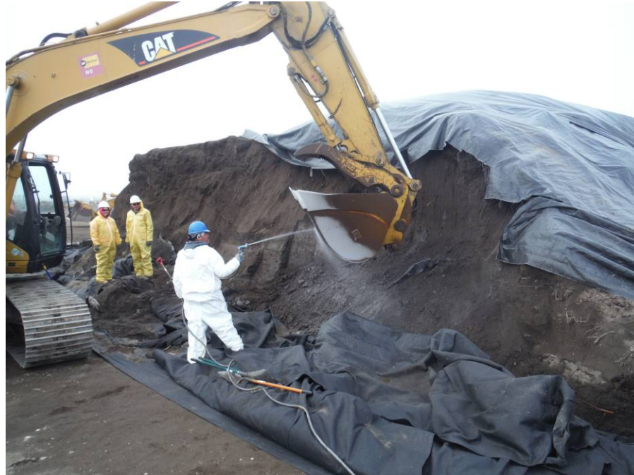
Photo No. 5 – 13 May 2014
