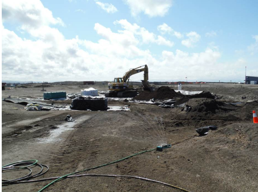
Photo No. 8 – 19 May 2014 Dust control measures around hoppers. View facing south.
