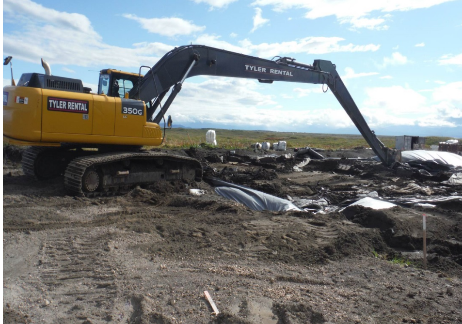
Photo No. 40 – 16 September 2014 Excavating non-TSCA PCB soil from stockpile CA 4. View facing south.
