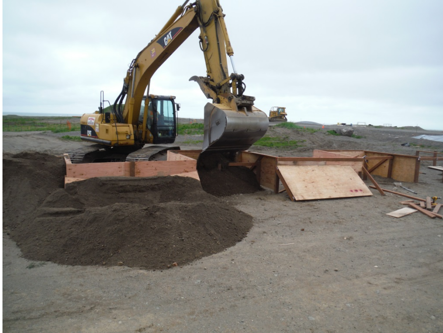
Photo No. 21 – 17 June 2014 Backfilling Super Sack workstation. View facing northwest.
