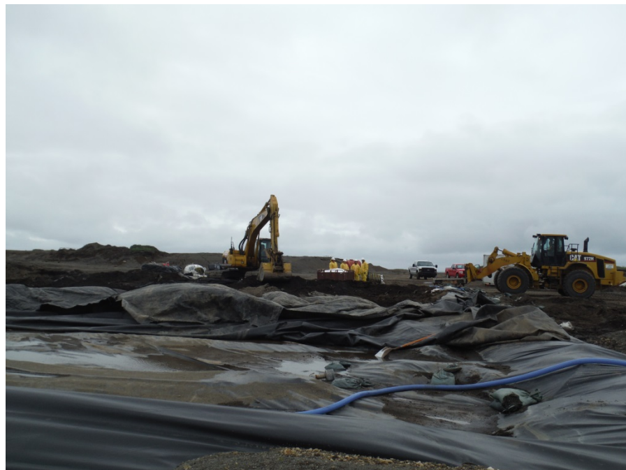
Photo No. 18 – 13 June 2014
