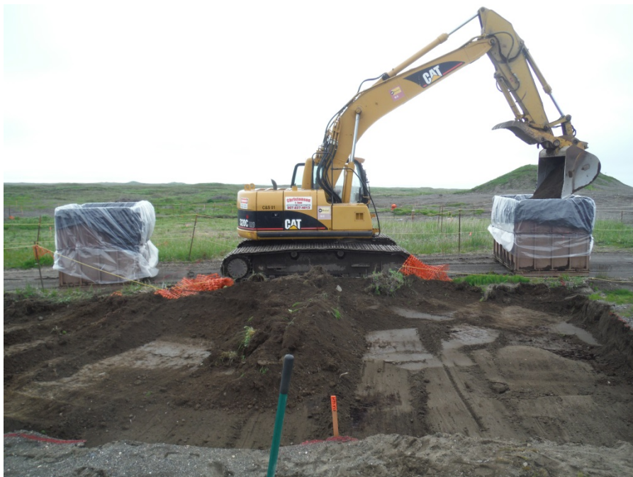
Photo No. 22 – 19 June 2014 Excavating into two hoppers at Soil Removal Area 2. View facing west.
