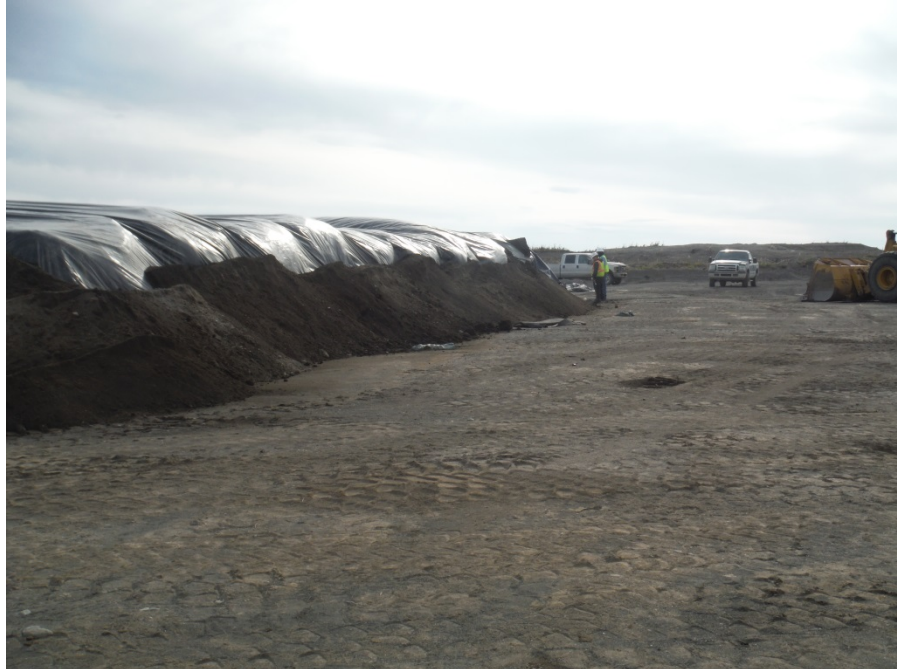
Photo No. 46 – 01 October 2014 Covered Super Sacks with berm at the former Port Heiden RRS. View facing east.
