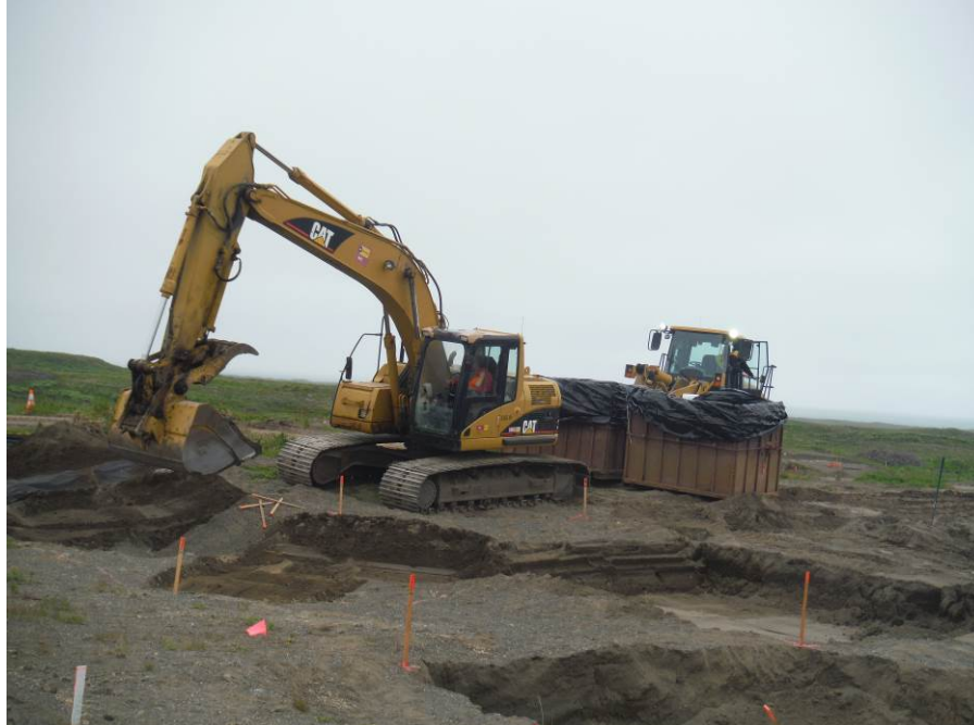
Photo No. 28 – 28 June 2014
