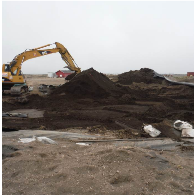
Photo No. 7 – 17 May 2014 Stockpile J 1.3 at 90-percent decommissioned. View facing east.
