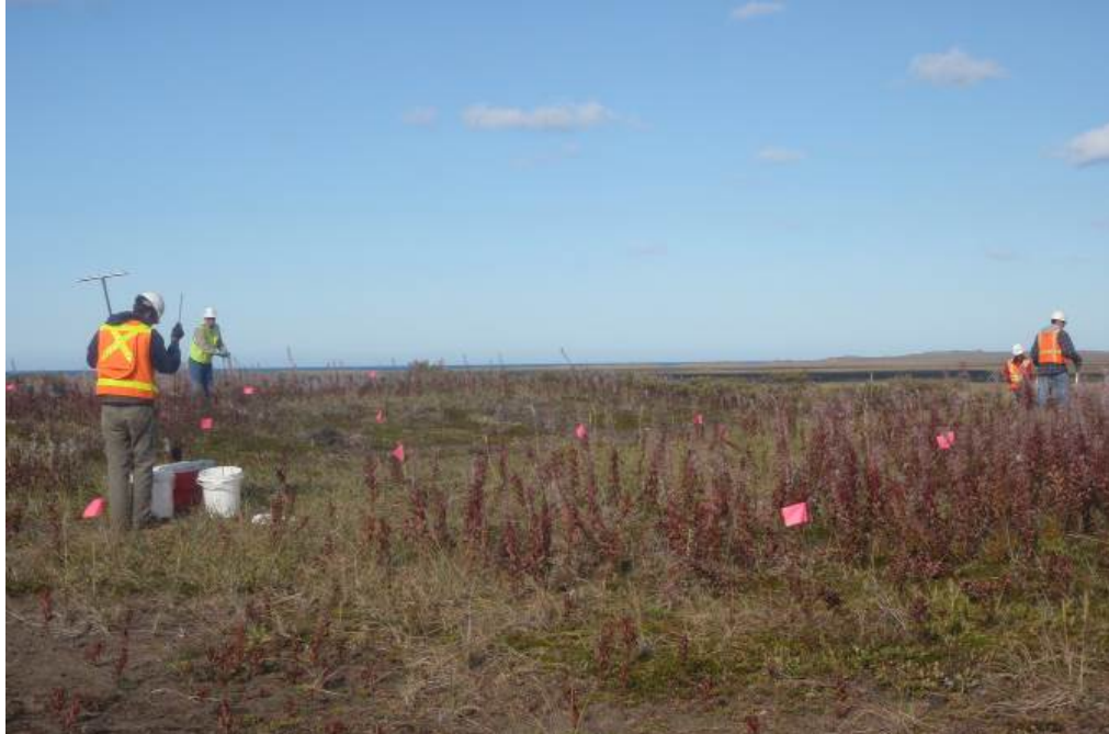
Photo No. 44 – 25 September 2014 Collecting characterization samples from the cap of the North Landfill. View facing west.
