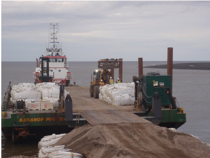
Photo No. 39 – 09 September 2014 ELM Solutions loading the lighterage barge. View facing west.
