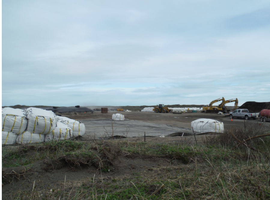
Photo No. 10 – 26 May 2014 Storage Area J 1 near the airport. View facing north.
