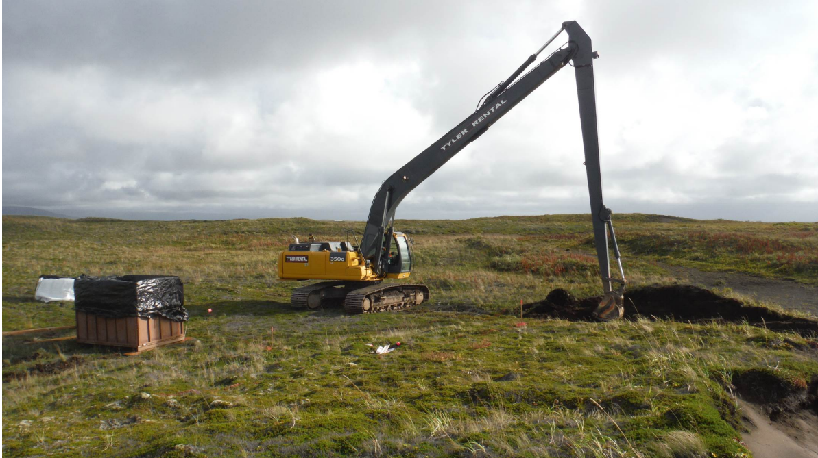
Photo No. 42 – 18 September 2014 Excavation of non-TSCA soil from Soil Removal Area 2. View facing south.
