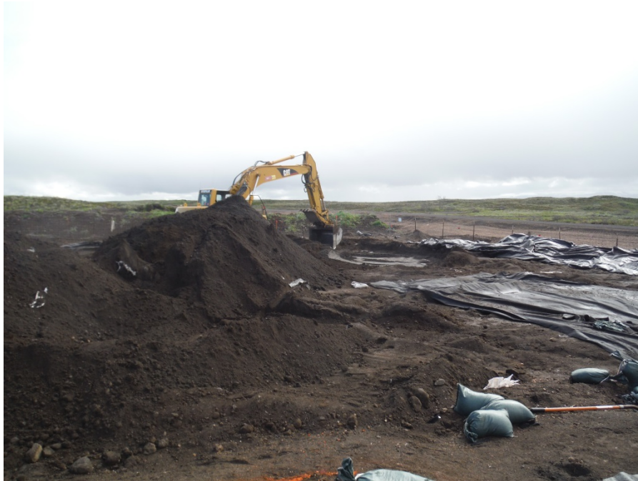
Photo No. 15 – 10 June 2014 Repositioning soil in Stockpile J 1.1. View facing east.
