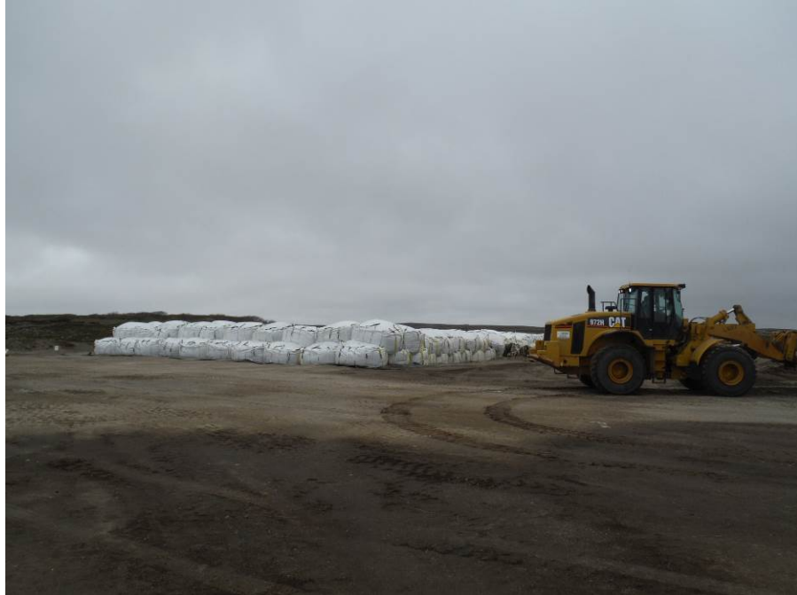
Photo No. 9 – 21 May 2014 Super Sacks staged in Storage area J 1. View facing northwest.
