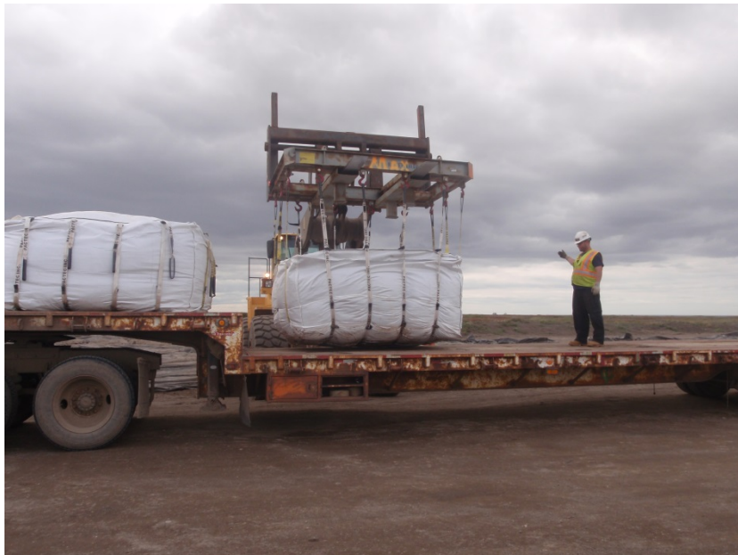
Photo No. 38 – 08 September 2014 Loading the final Super Sacks from Storage Area J 1 onto the trailer. View facing southwest.
