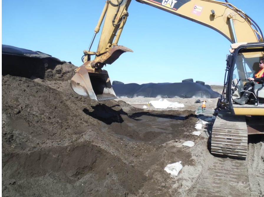
Photo No. 4 – 10 May 2014 Excavator loading soil from Stockpile J 1.3. View facing west.
