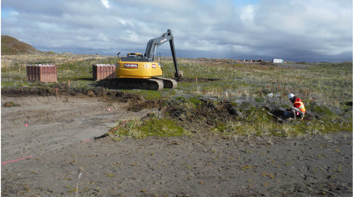
Photo No. 43 – 20 September 2014 Collecting step-out samples from Soil Removal Area 2. View facing east.
