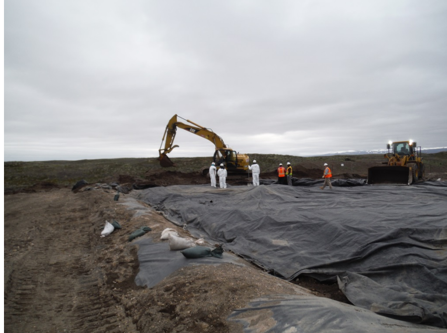
Photo No. 12 – 02 June 2014 Removing the liner from Stockpile J 1.5 in Storage Area J 1. View facing east.
