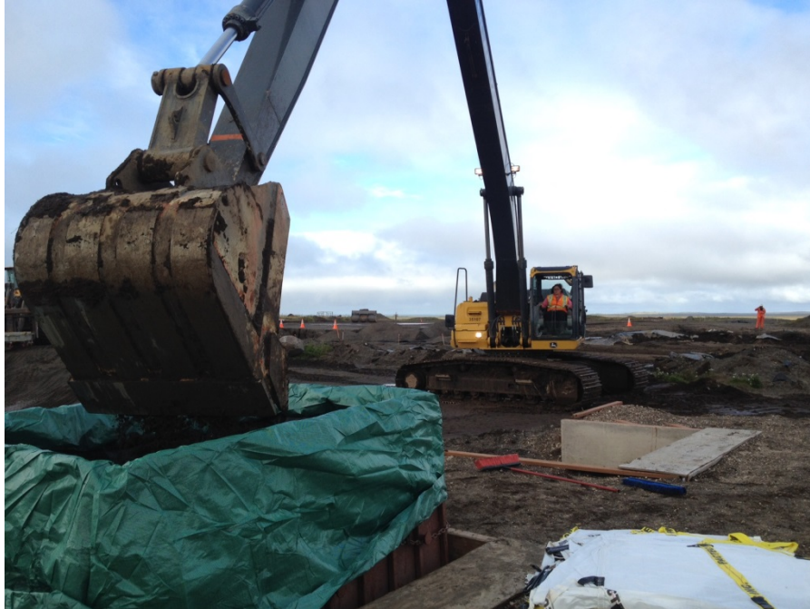
Photo No. 41 – 17 September 2014 Long-reach excavator filling super sack from stockpile CA 4. View facing northeast.
