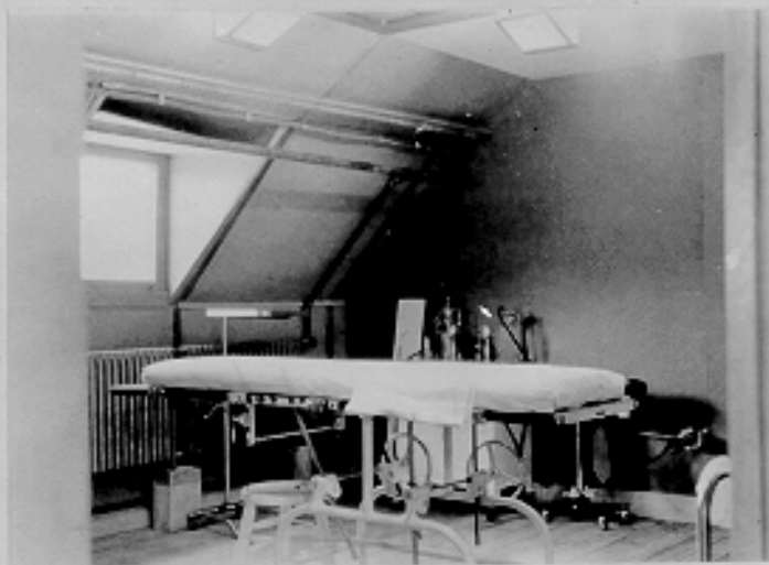
Hospital surgery building, interior view of operation room before painting. Nome Garri- son, Alaska. 6-28-43
