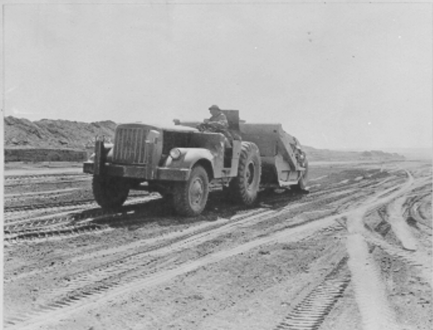
Showing carryall spreading material on "C" (C496) runway. Fort Glenn, Umnak Island, Alaska. 7-4-43
