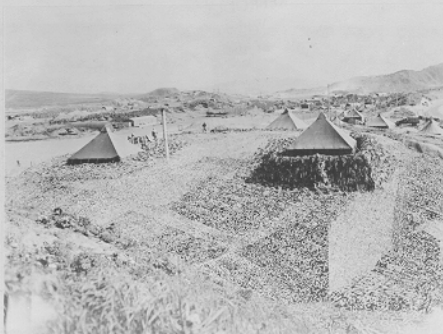
Showing complete camouflage on top of T- (C506A) hangar #1. Adak, Alaska. 6-29-43
