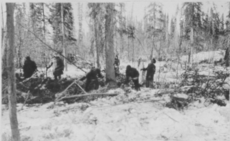
Cutting power and telephone poles. CAA Garrison, Galena, Alaska. 3-30-43
