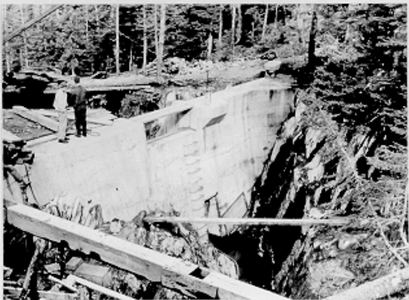
Upstream face of Cove Creek Dam. Alaska Railroad Passage Canal, Whittier, Alaska. 9-4-43
