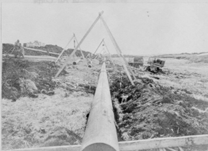
Pipe held with tripods for welding. Amchitka, Alaska. 5-19-43
