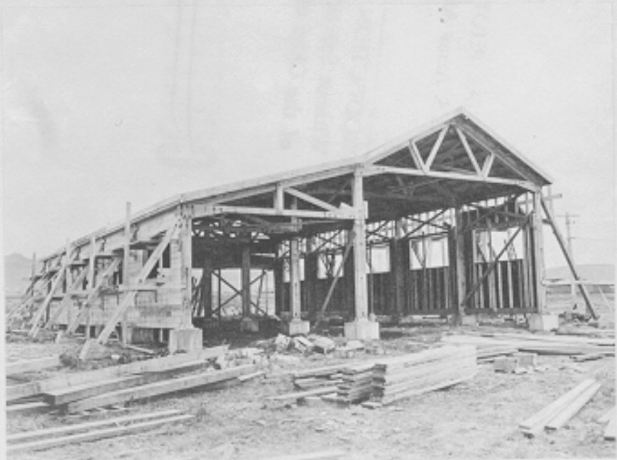
(G501A) Machine shop construction. Fort Glenn, Umnak Island, Alaska. 8-10-42
