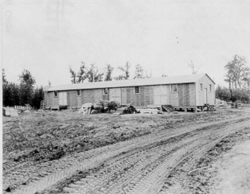
(C500) T/O Warehouse - completed (exterior). CAA Bethel, Alaska. 8-2-43
