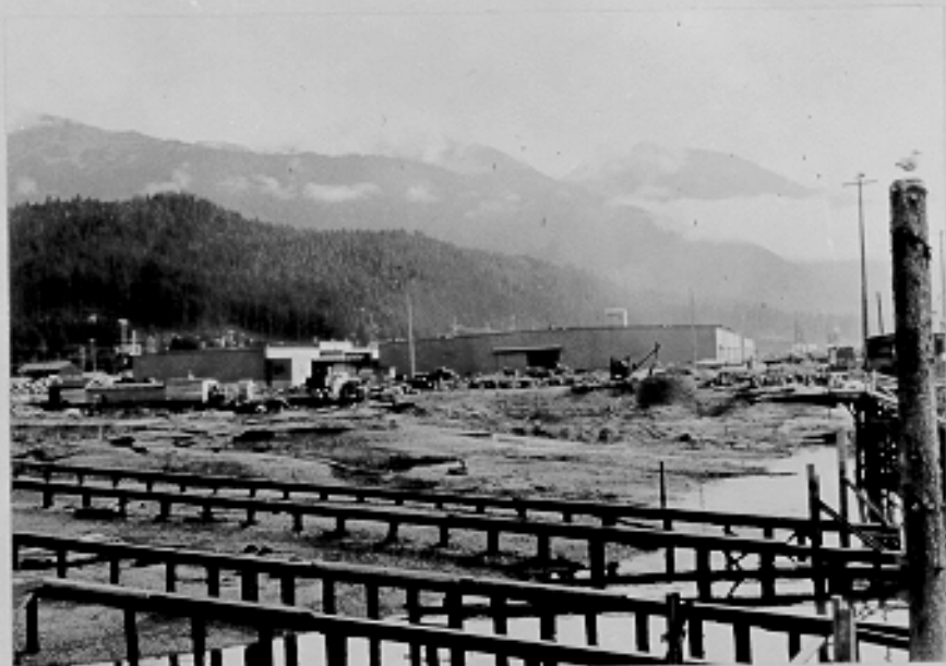
Dock unit #1 - Marine Ways in foreground - looking southeast from cannery oil dock. Excursion Inlet, Alaska. 9-7-43
