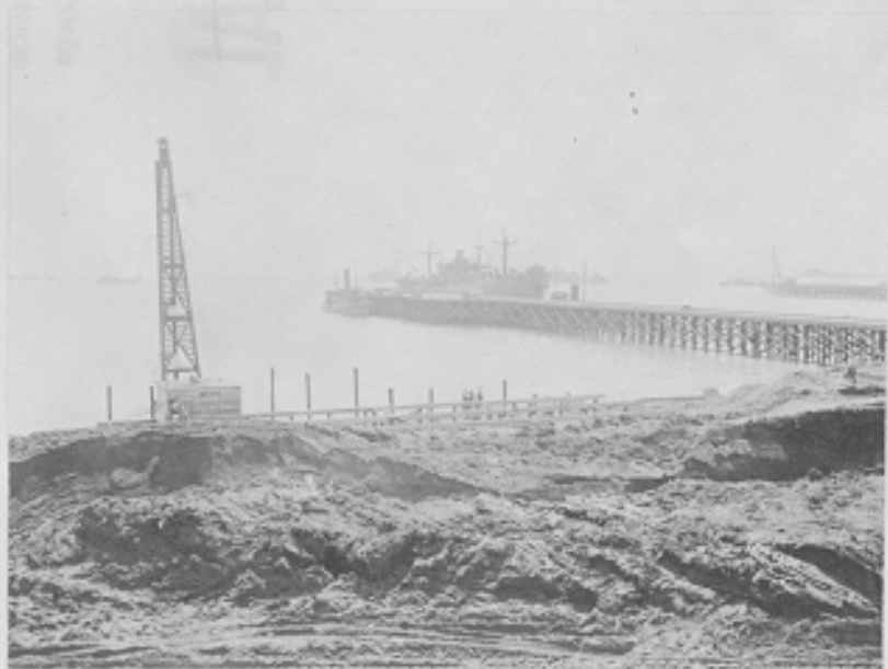
Dock and marine way construction. Attu Island, Alaska.
