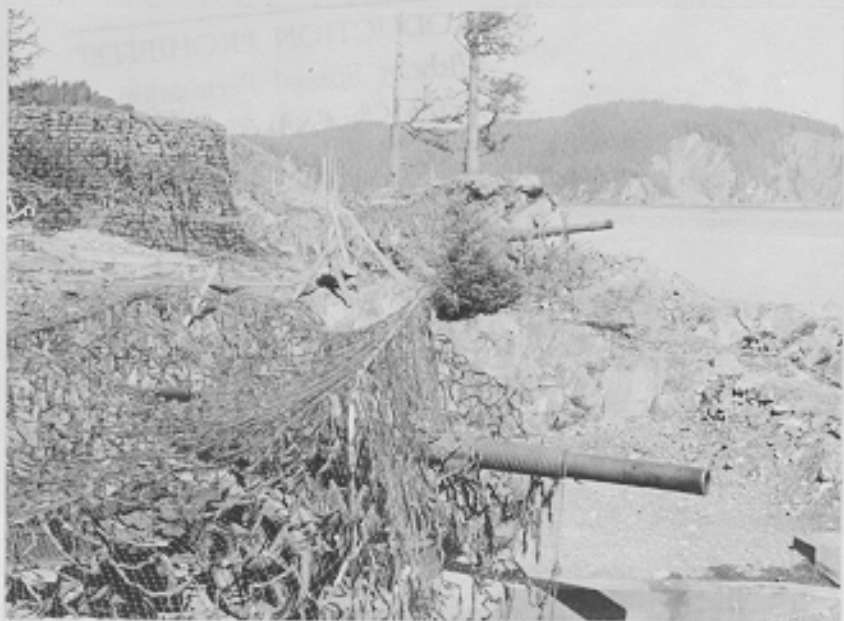
(C504A) Panama Mounts #2 and #3, looking north. Rocky Point, Battery 293, Seward, Alaska. 5-10-43
