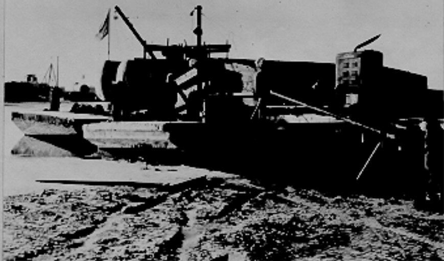
Average type conditions on barge lightering gas storage. Nome Garrison, Alaska. 10-9-42
