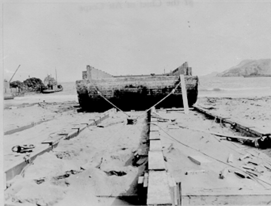
(C502) Front view of barge on Marine Ways. Adak, Alaska. 3-29-43
