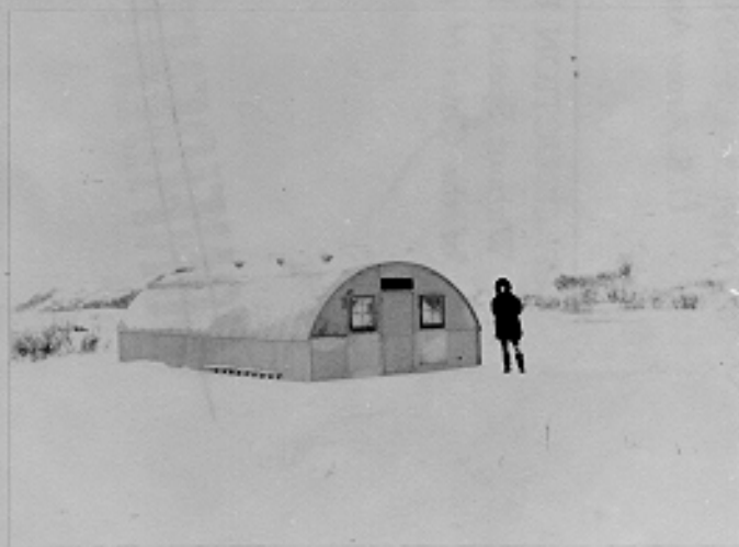
Quonset hut in ice, Anvil Creek, north end of hospital area. Nome Garrison Project, Alaska. 1-17-43
