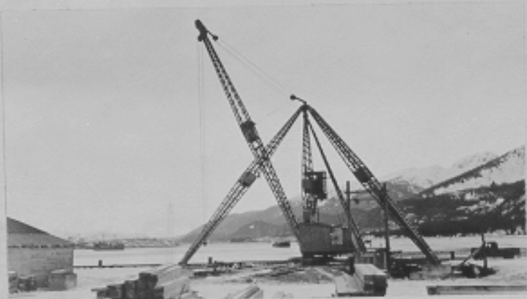
Stiffleg derrick. Juneau Port Expansion Project, Alaska. 1-17-43
