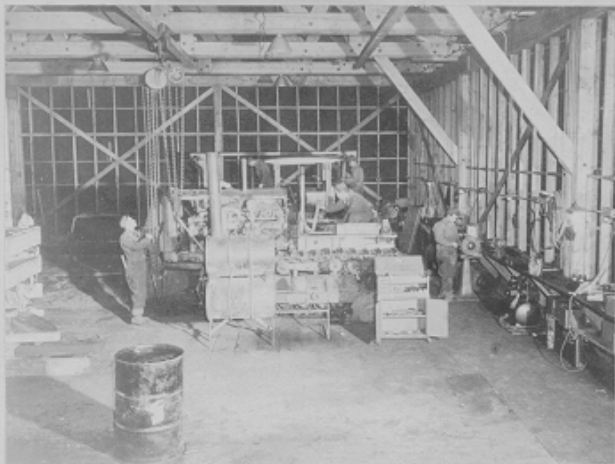
(C501) Construction area, cat repair shop. Fort Glenn, Umnak Island, Alaska. 11-8-42
