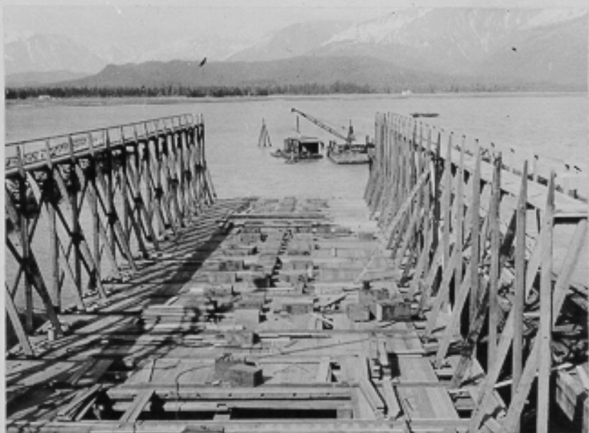
Marine railway cradle, looking northeast. Seward, Alaska. 6-1-43
