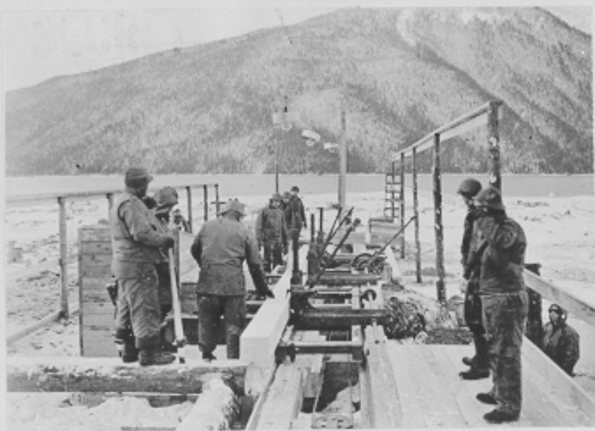
Saw mill and south creek - 331st Engineer (C510) Operation. Excursion Inlet, Alaska. 12-18-42
