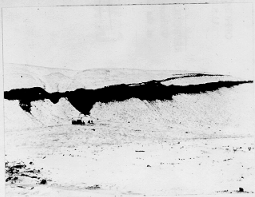
Idak Road in construction on Idak Peak. Fort Glenn, Alaska. 12-13-42 (C492D)
