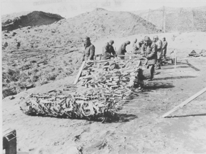
(C506B) Engineers threading garlands through chicken wire for Air Corps gas tanks. Adak, Alaska. 3-29-43
