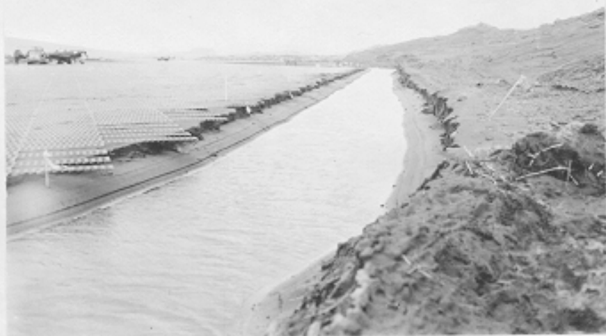
Drainage ditch along east side of Runway "A", Longview, Alaska. 11-5-42
