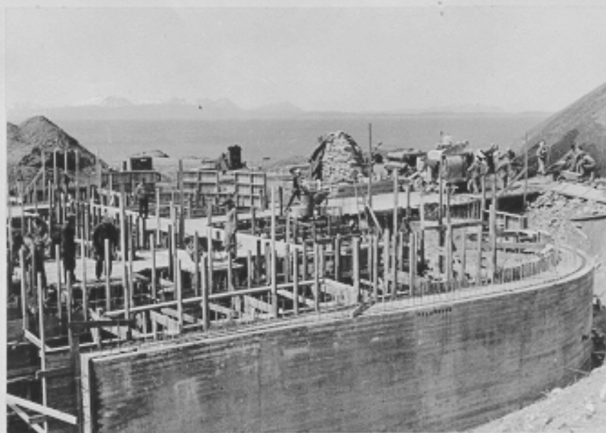
(C504) Walls and footings, 8" battery #403. Chiniak Point, Fort Greely, Alaska. 6-1-43
