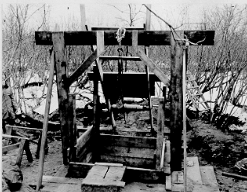
Dug well in Air Corps area. CAA Bethel, Alaska 3-6-43
