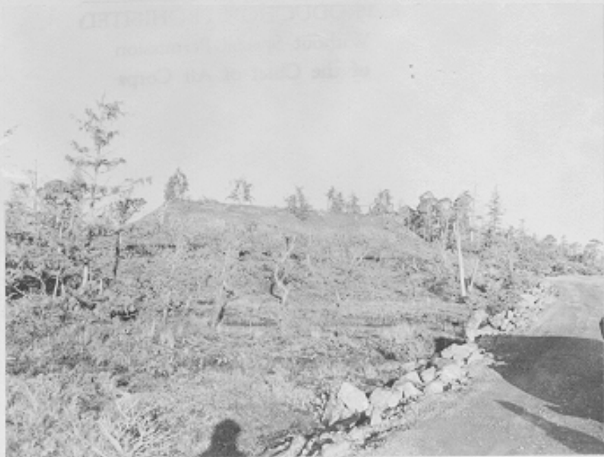
Completed camouflage on tank No. 6 in Operations Reserve Gasoline System. Looking northeast from (C506C) 300' away. Annette Island Landing Field, Alaska. 2-20-43
