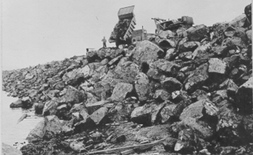
Placing rock armor plating on breakwater. Amchitka, Alaska. 8-1-43
