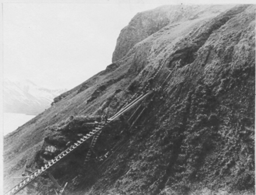
(C488A) Tramway trestle construction. AWS Cape Wislow, Alaska. 6-15-42
