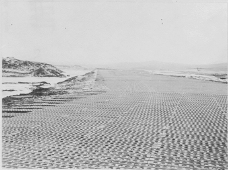
(C496J) Completed portion of runway "B". Adak, Alaska. 1-4-43
