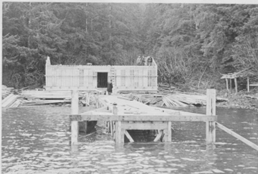
Construction of Powder Magazine and dock for construction. Excursion Inlet, Alaska. 4-22-43
