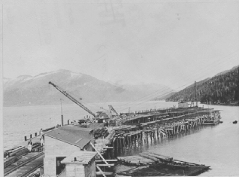
Whittier dock under construction. Alaska Railroad Passage Canal Connection. 9-26-42
