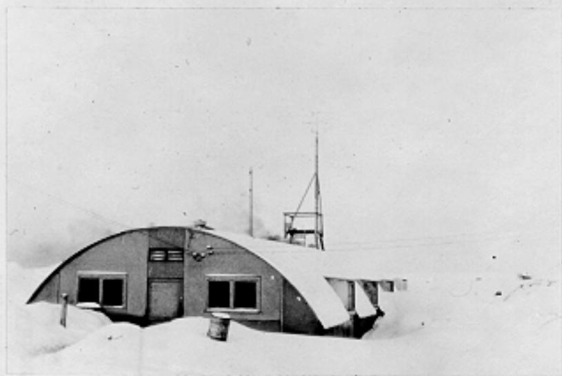
Air Corps weather station. Quonset hut (24 x 60) showing winter conditions. Fort Morrow, Port Heiden, Alaska. 1-24-43
