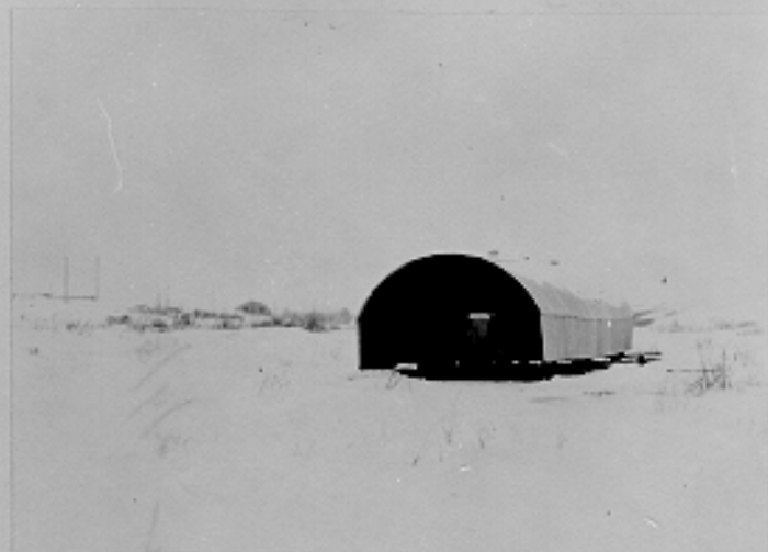
Quonset hut being jacked up prior to moving - Anvil Creek, north end hospital area. Nome Garrison Project, Alaska. 1-17-43
