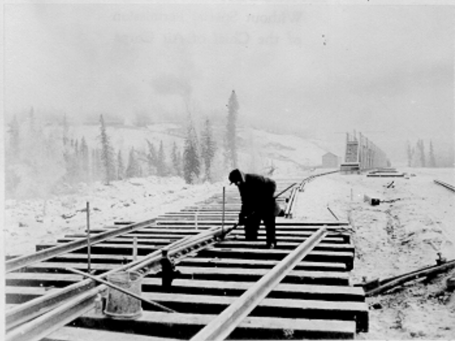
(C507A) Railroad spur to gasoline loading racks, Fort Richardson. 12-1-42
