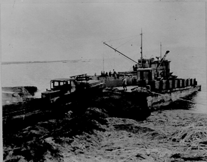
Unloading runway steel from barge. Attu Island, Alaska. 6-2-43
