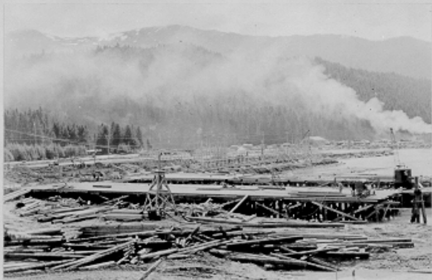
Marine Ways and Marine repair shop, looking southeast. Excursion Inlet, Alaska. 7-13-43
