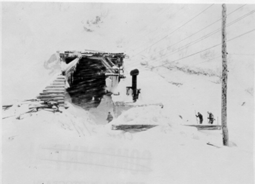
Snow shed at south portal of Passage Tunnel showing drifted snow at entrance and sides. Alaska Railroad Cut-Off Project, Whittier, Alaska. 1-10-43
