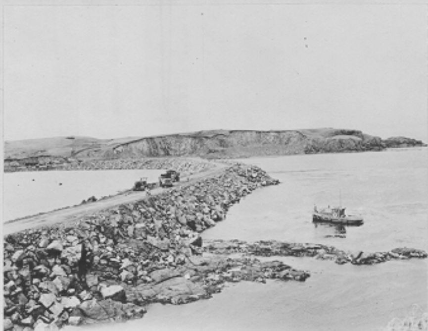
(C497A) Roadway on breakwater. Quarry in background. Amchitka, Alaska. 8-1-43
