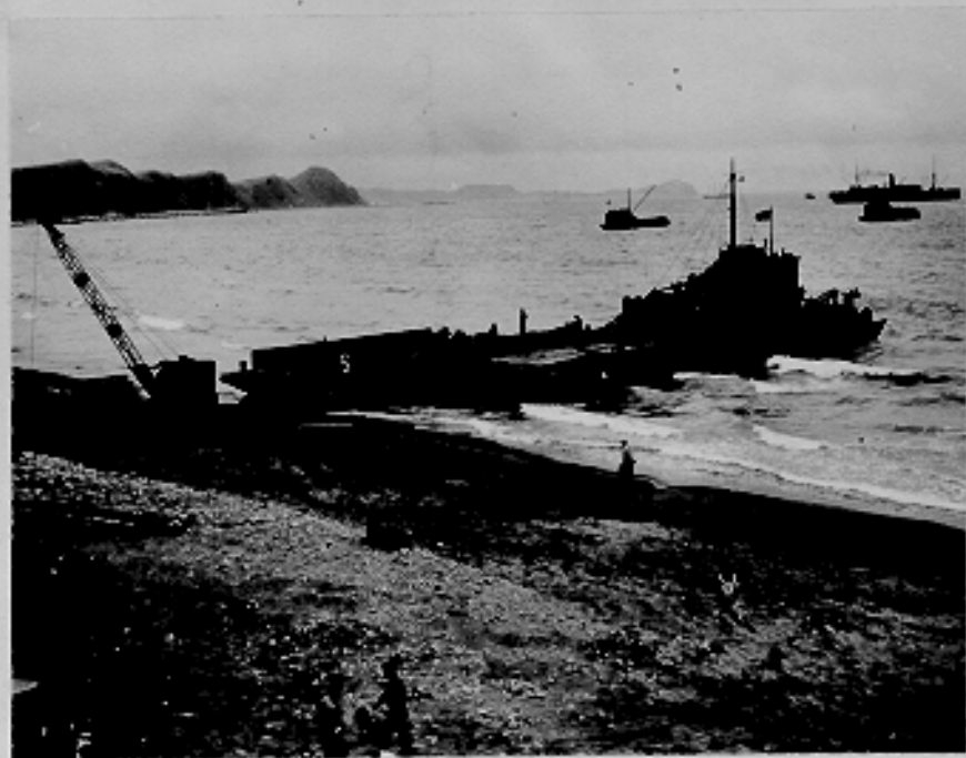
(C498) First barge unloading of heavy equipment. Adak, Alaska. 8-31-42
