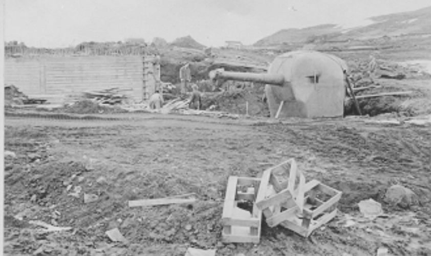
Installing 6" Gun. Dutch Harbor, Alaska. November, 1942
