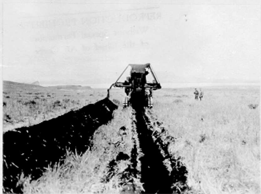
Ditch digger working on permanent water supply line. Fort Glenn, Alaska. 8-10-42
