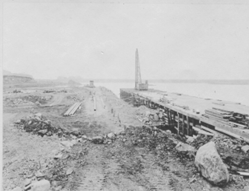
Kirilof dock and fill, looking northeast. Amchitka, Alaska. 7-29-43
