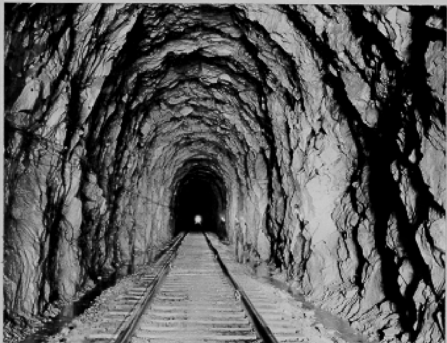
Turnagain Tunnel interior, looking through toward Bear Valley. Whittier, Alaska. 6-10-43
