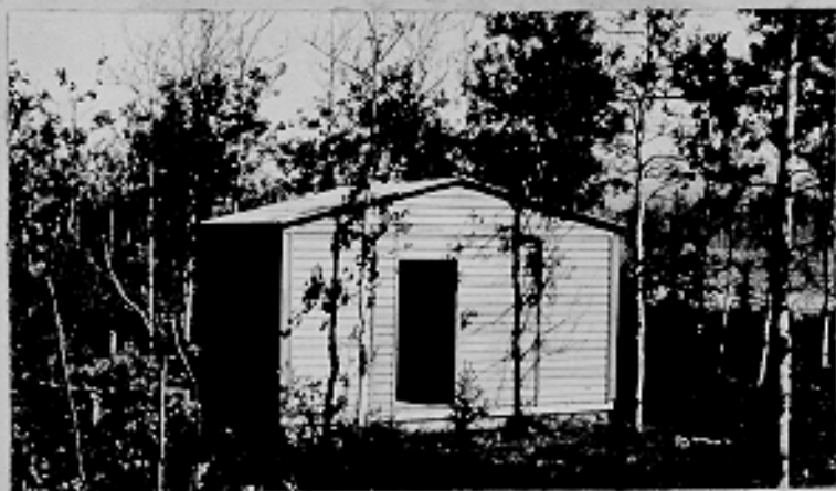
Yakutat hut, Revetment "A", Fort Richardson, Alaska. 6-20-42
