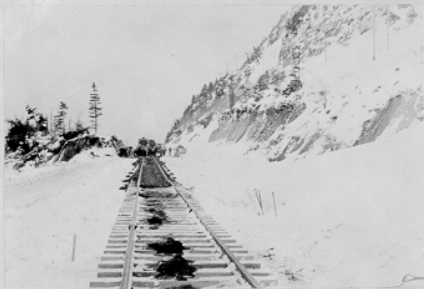
Looking south from station 63 + 00 towards ballasting operations. Alaska Railroad out-off Project, Whittier, Alaska. 4-5-43
