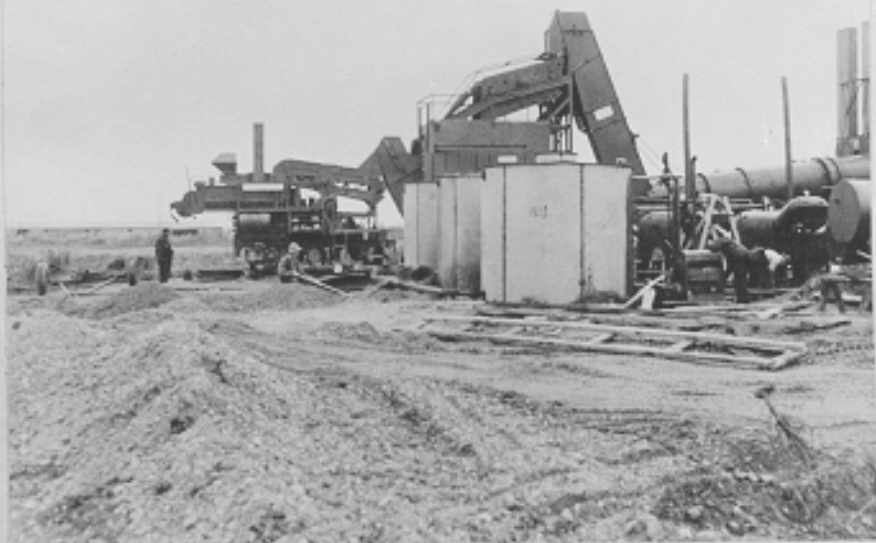
View of asphalt plant. Ladd Field, Alaska. 8-20-43
