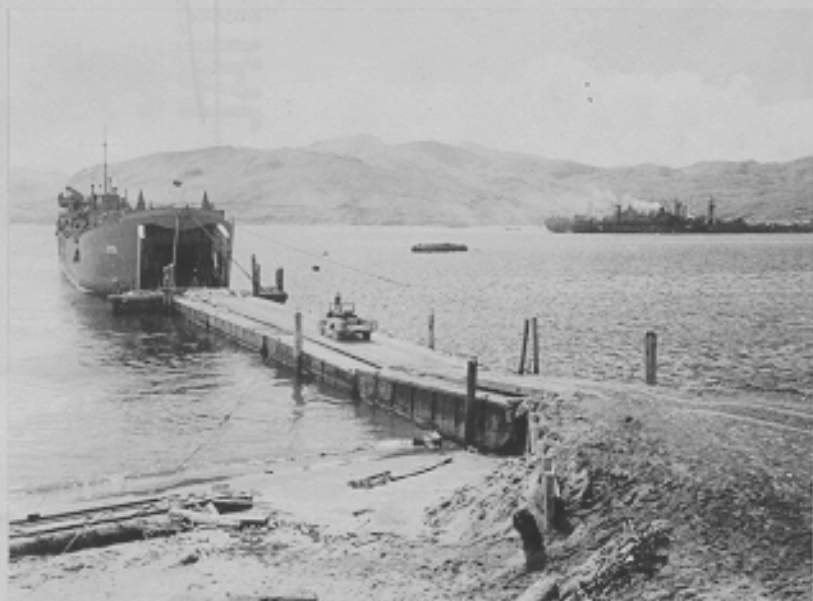
LST dock. Adak, Alaska. 8-12-43 (C491D)
