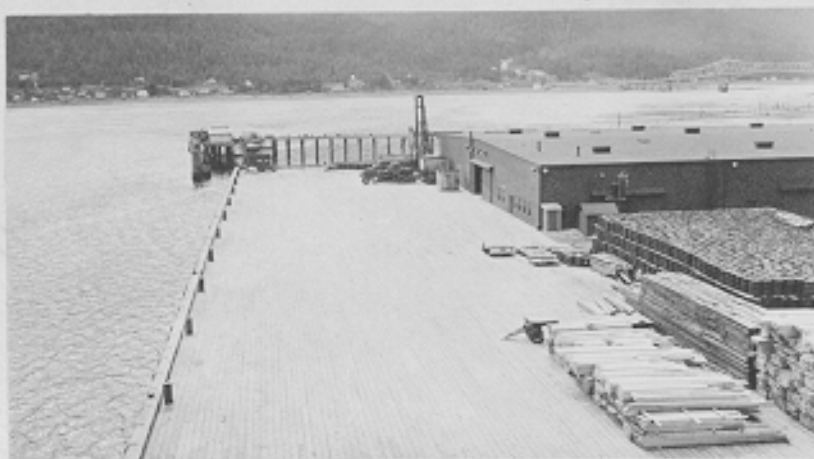
(C500C) Looking west along wharf. Juneau Port Expansion, Alaska. 5-17-43
