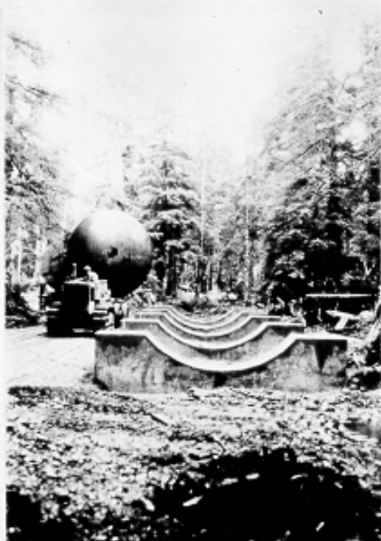
ACOR tank in transit to concrete saddle foundations. Yakutat Landing Field, Alaska. 9-9-42
