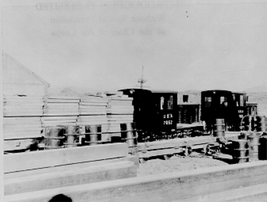
Maintenance and operation at Kougarok Railroad (C507B) (Narrow Gauge) Nome Garrison Project. 10-15-42
