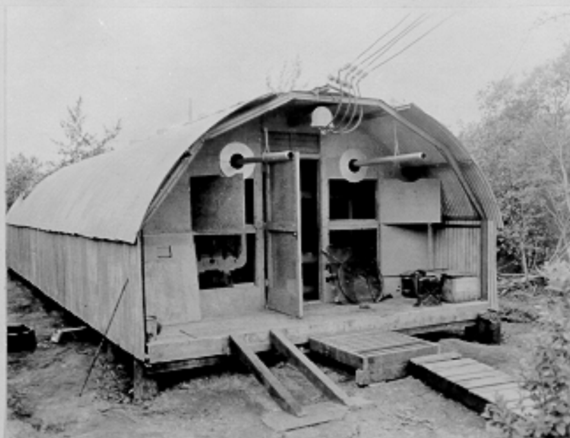
Exterior of powerhouse, rear view. CAA Bethel, Alaska. 7-12-43
