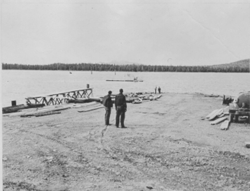
Looking at seaplane ramp from road inter- section. Annette Island, Alaska. 4-7-43
