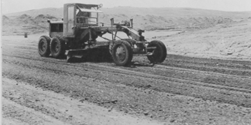
Grading "C" runway. Fort Glenn, Umnak Island, Alaska. 7-4-43
