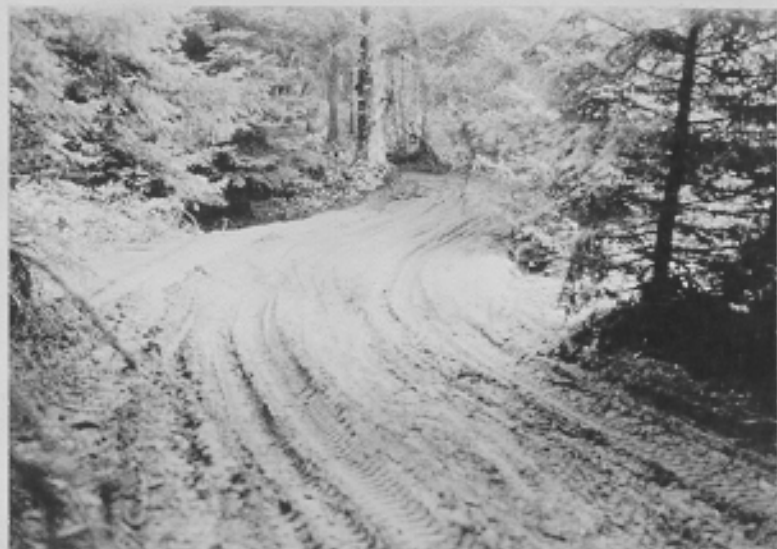
Typical section of road to Ocean Cape - Point Carrew. Yakutat Landing Field, Alaska. 9-23-42
