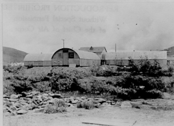
Exterior view of hospital supply building constructed in "T" shape using three Quonsets. Nome Garrison, Alaska. 6-28-43
