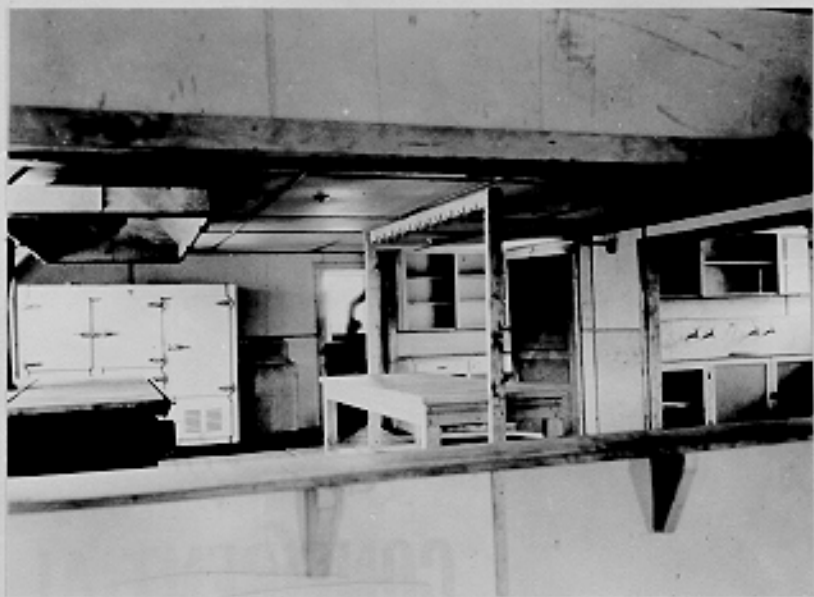
Mess hall (kitchen). CAA Bethel, Alaska. 3-6-43
