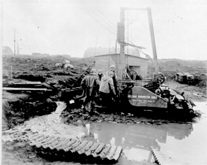
Well digger, drilling at bakery. Cold Bay, Fort Randall, Alaska. 11-8-42.
