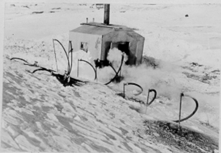
View of steam thaw points. Nome Garrison, Alaska. 3-29-43
