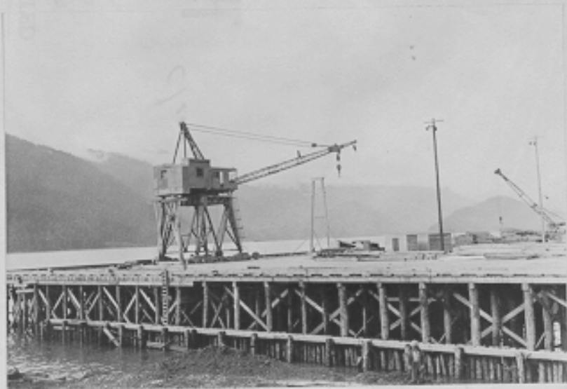
Partially erected 20-ton Gantry crane on ship dock #2, looking northwest from cannery canning building. Excursion Inlet, Alaska. 9-7-43
