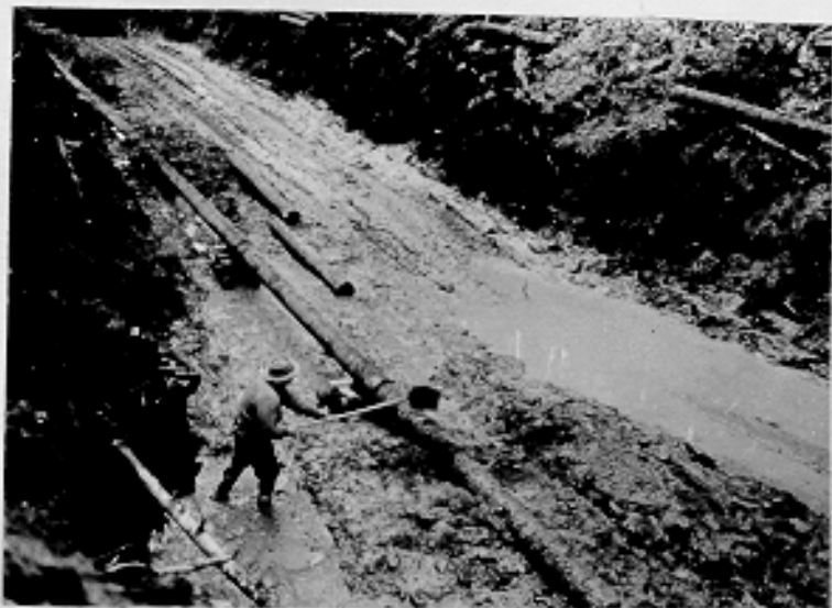
North Ramp Road showing muskeg. Excursion Inlet, Alaska. 4-28-43
