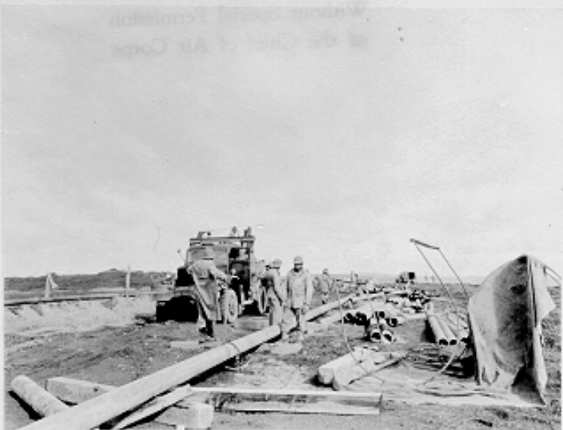
Welding pipe for dock water line. Fort Randall, Alaska. 8-27-43
