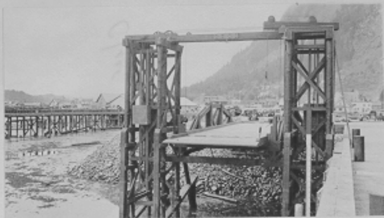
Gridiron transfer bridge. Juneau Port Expansion, Alaska. 5-17-43
