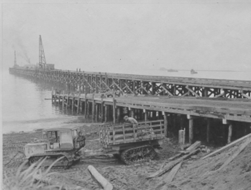
LST ramp construction, 98% complete. Attu Island, Alaska. 7-17-43
