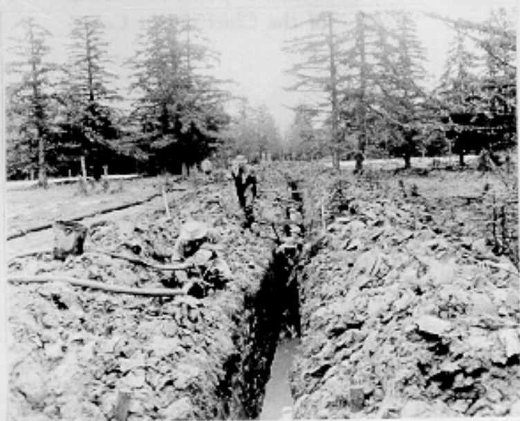
View showing difficulties encountered in installing 4" sewer line from ACS area at Mile 11 to Mendenhall river. CAA Garrison, Juneau, Alaska. 4-20-43 (C494H)
