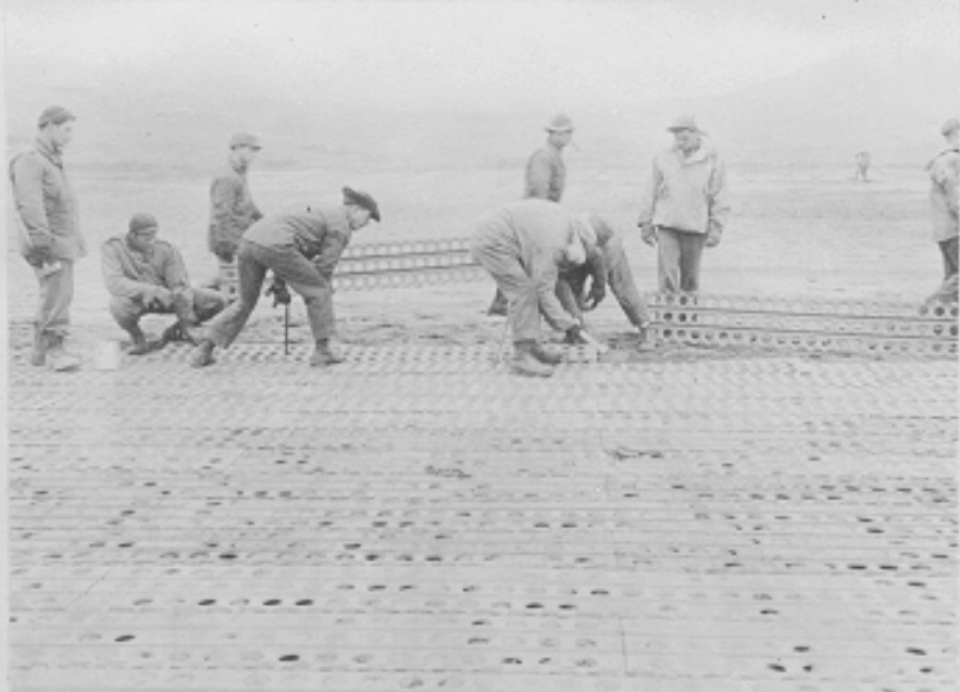
Laying steel mat runway "A", Alexai Point, Attu Island, Alaska. 7-11-43
