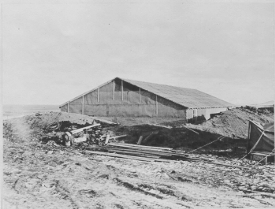
Completed warehouse in area G. Fort Glenn, Alaska. 12-22-42
