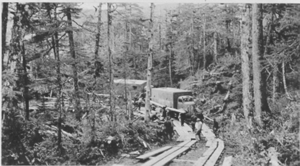
(C488D) Landing and moving mobile radar equipment to site. View of 2 pieces of equipment following first one around curve to top of hill. 3" x 12" planks used. Jeanie Point, Montague Island, Alaska. 5-22-42
