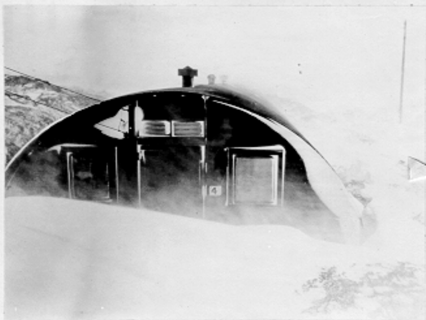
(C488E) Snowbank against Quonset Hut -- capacity 10 men. At some Alaska stations temperature often down to 70 below. Engineers and Engineer supervised civilian workers as well as troops occupied these shelters. Fort Randall, Alaska. 11-21-42
