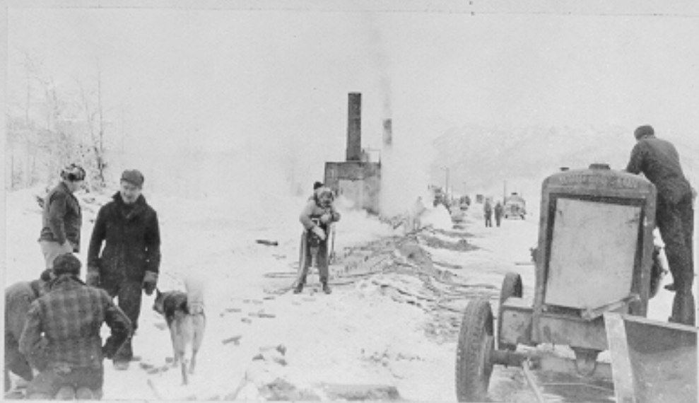
Drilling holes for steam thawing of trench. (C513E) Fort Richardson, Alaska. 12-27-41
