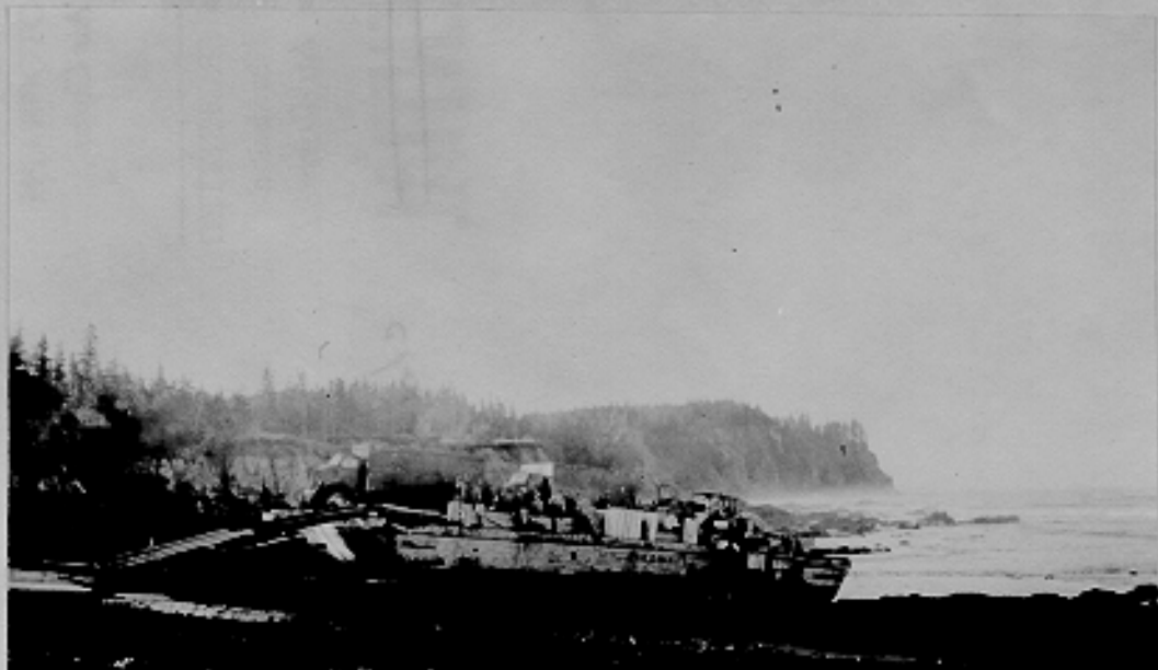
(C498A) Landing and moving mobile radar equipment to site. Picture taken in a southerly direction. Mobile site is about 1 mile distant in center foreground. Jeanie Point, Montague Island, Alaska. 5-12-42 - 5:00 a.m.
