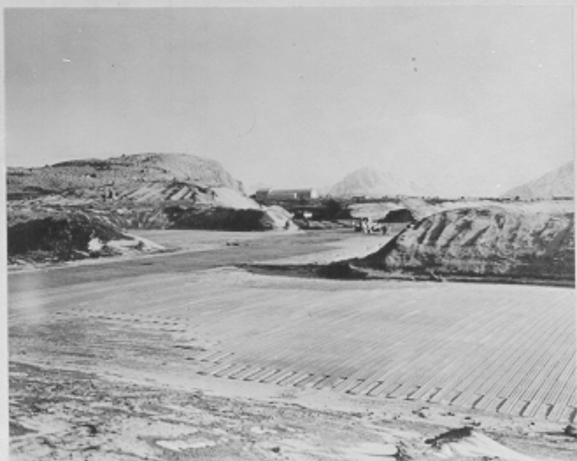
(G496H) Runway "B" revetment. Adak, Alaska. 3-1-43
