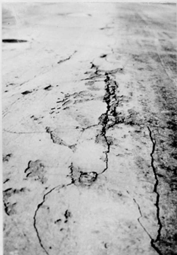
Glacial action beneath runway caused cracks in 1000 feet of west end of east-west runway. Naknek, Alaska. March, 1942
