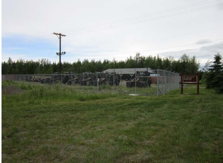
Photo No. 13 – 27 June 2012
