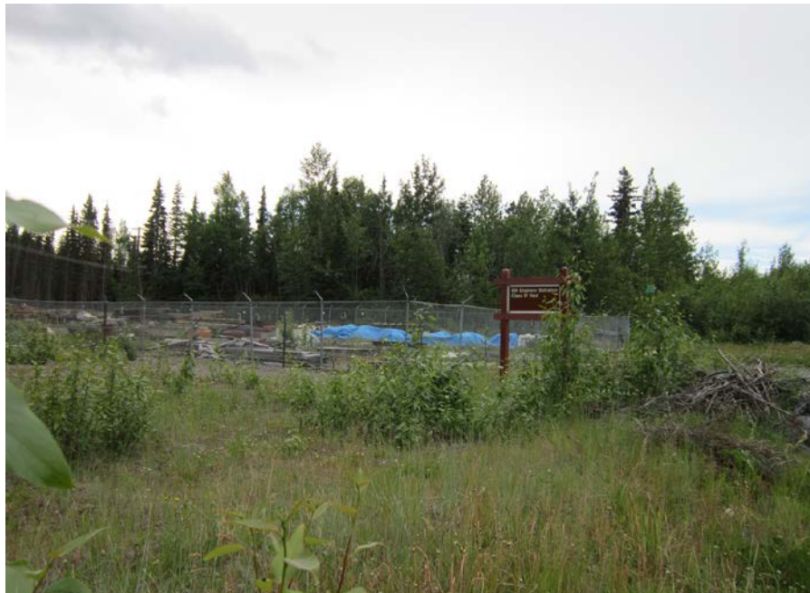
Photo No. 10 – 27 June 2012 U.S. Army 6 th Engineer Battalion Class IV Yard located within the OUE AVMA site area (facing south-southwest).
