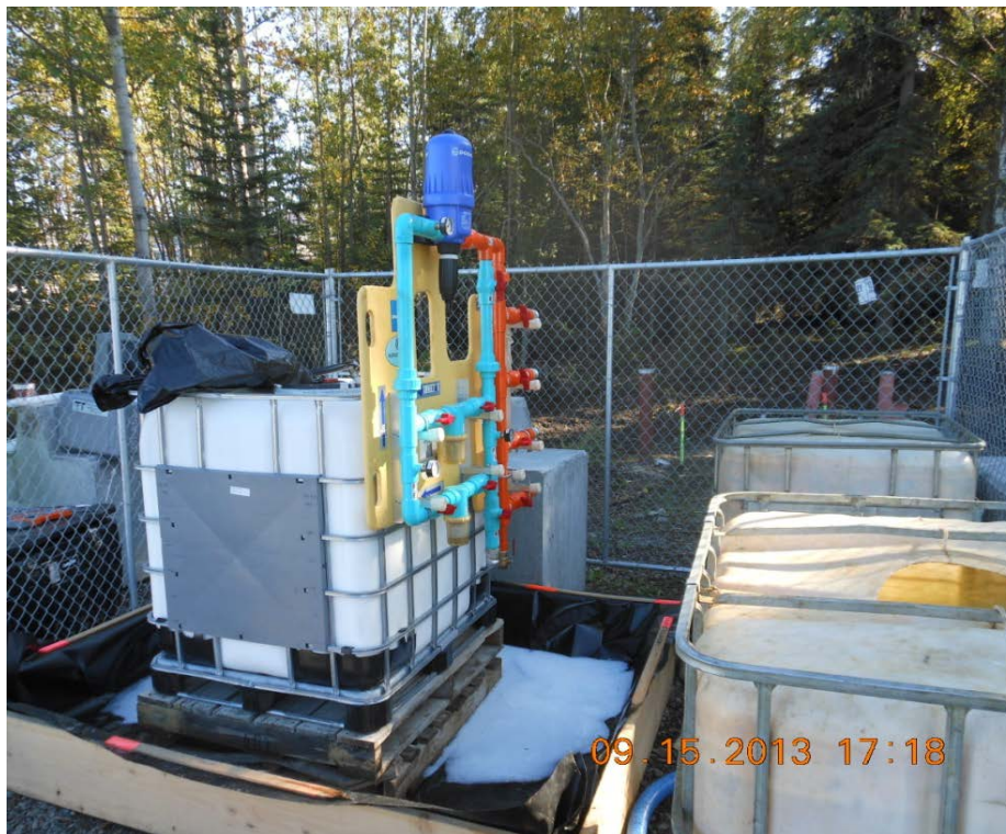
Photograph A-10: Injection system mounted on EVO tote in secondary containment (September 2013). Note rainwater in secondary containment with a few ounces of EVO spilled into it is visibly white
