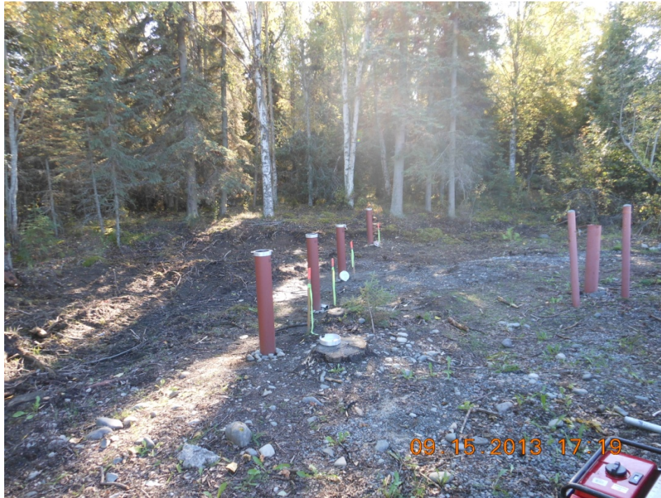
Photograph A-13: Row of injection wells upgradient of performance monitoring well (September 2013)
