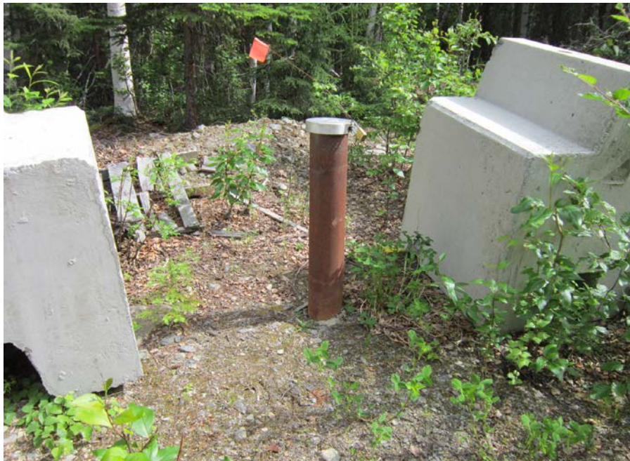
Photo No. 4 – 27 June 2012
