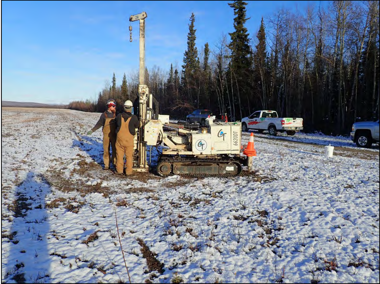
Photograph C.3-17. Drilling TW19 in the Chena Flood Control Project.
