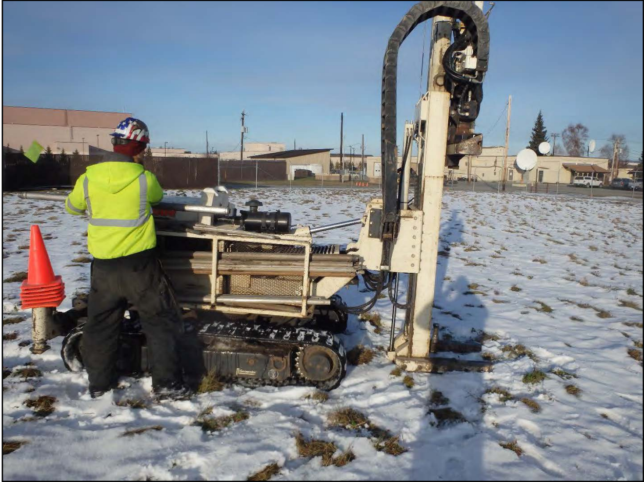
Photograph C.3-9. View of drilling of 19PS-FST1-SB02.
