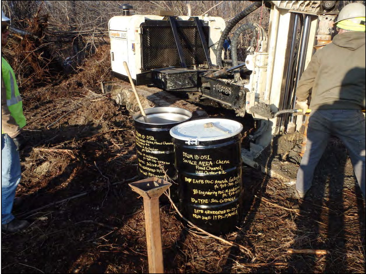
Photograph C.2-2. Containment of soils extracted from 19PS-MW02A.
