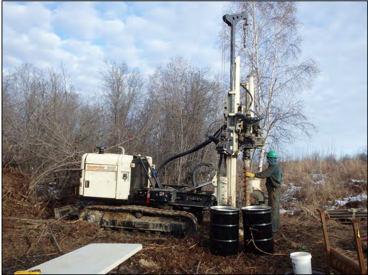
Photograph C.2-1. Drilling of 19PS-MW02A.
