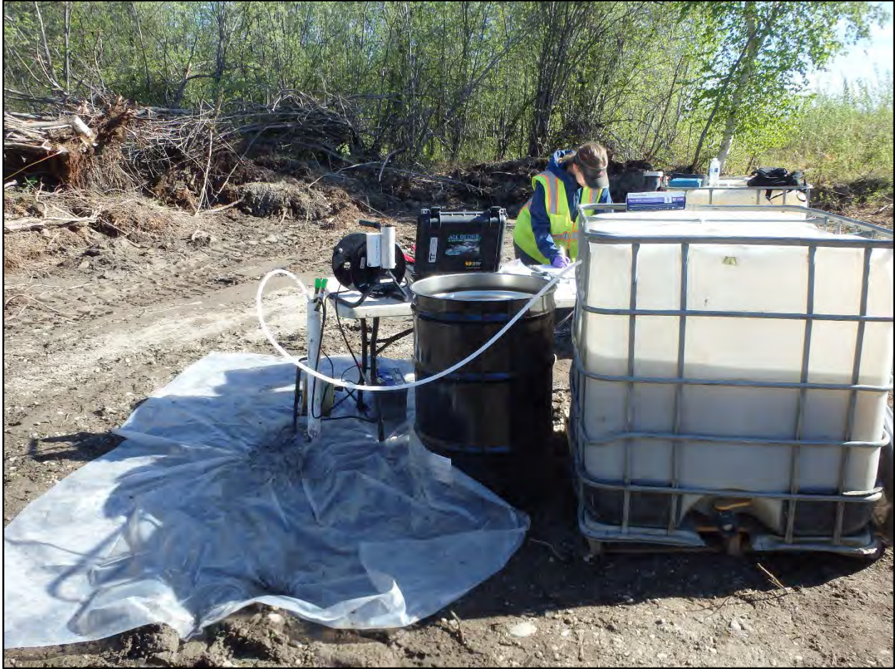
Photograph C.2-18. Purging process during development of 20PS-MW02D.
