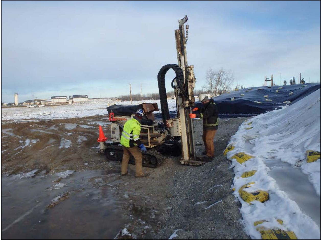
Photograph C.3-3. View of drilling of 19PS-FFTA-ENT-SB06.
