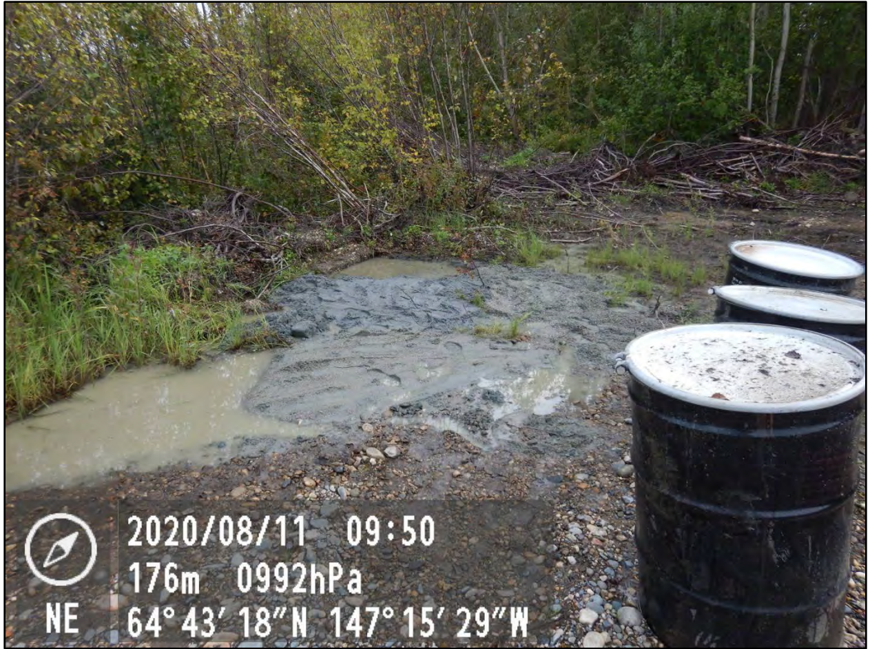
Photograph C.6-2. Surface disposed soils from Well Cluster #1 drums 121, 122, and 130.
