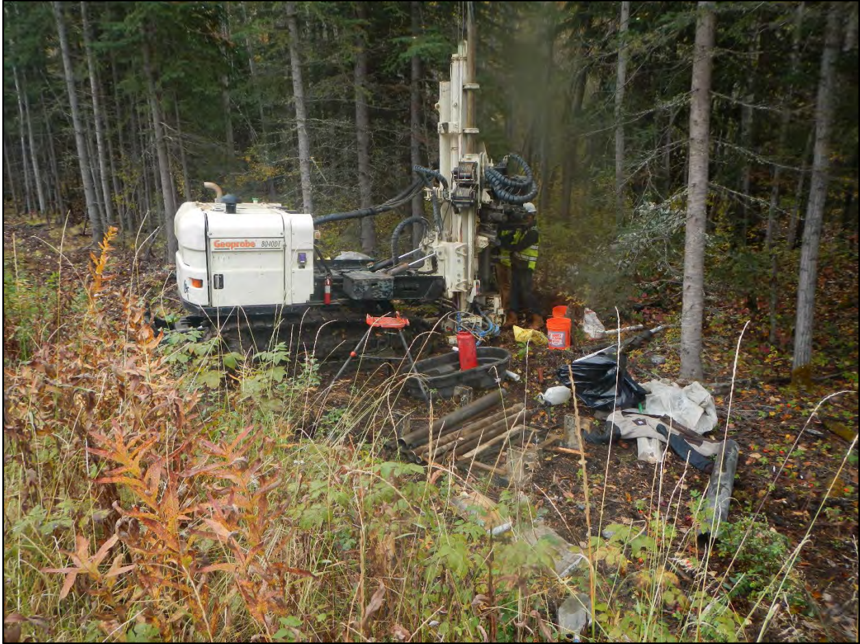
Photograph C.4-3. Screen and casing being placed at MW-13.
