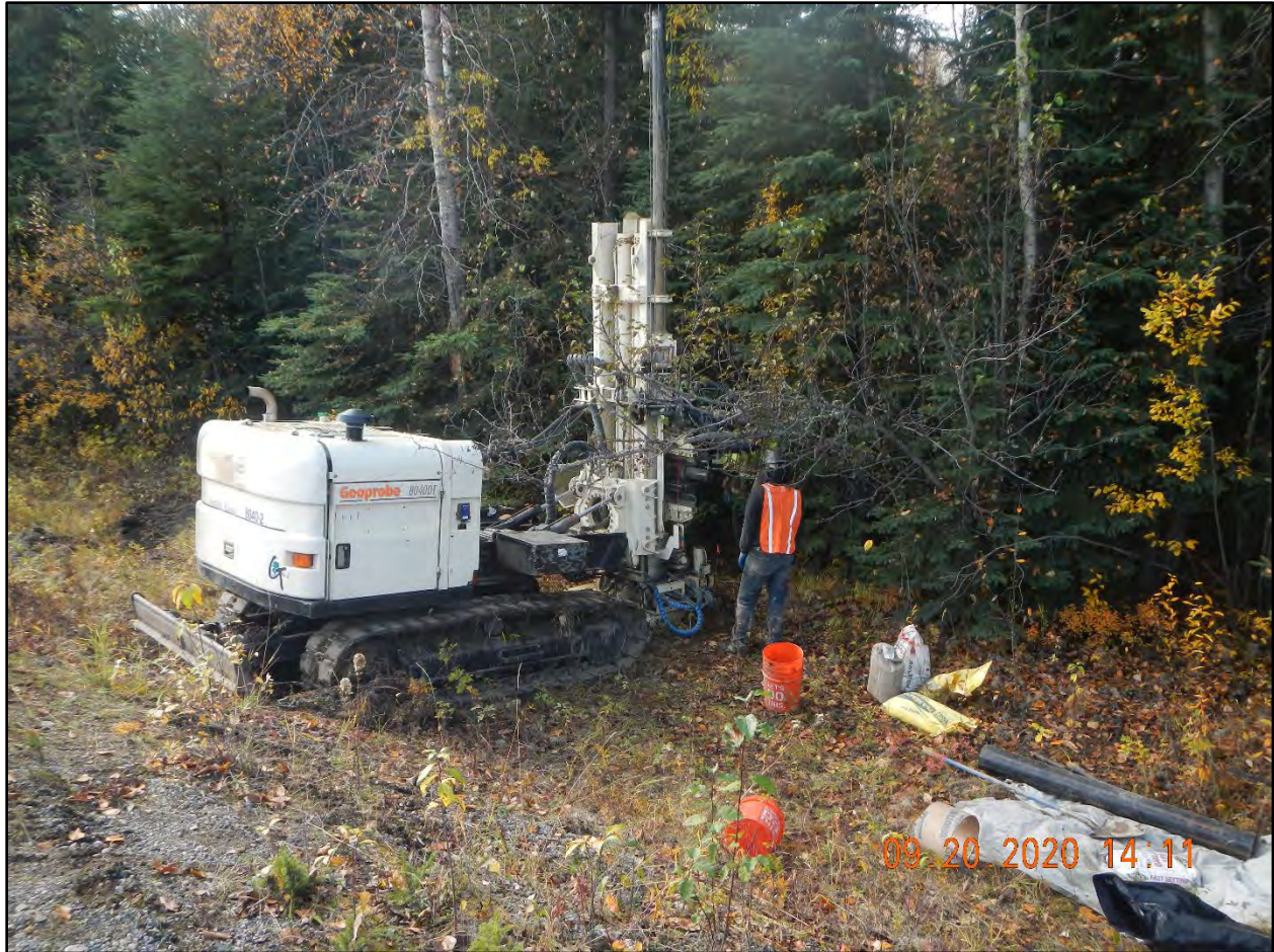
Photograph C.4-10. Drilling of MW-1.
