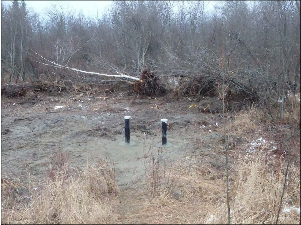
Photograph C.2-12. View of completed wells 19PS-MW2A and 19PS-MW2B in Well Cluster #2 area.
