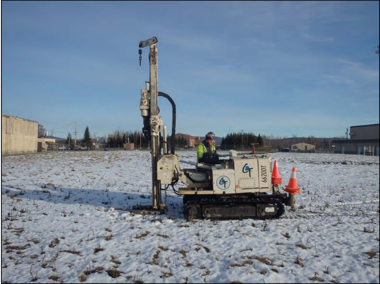
Photograph C.3-6. View of drilling of 19PS-FST1-SB06.
