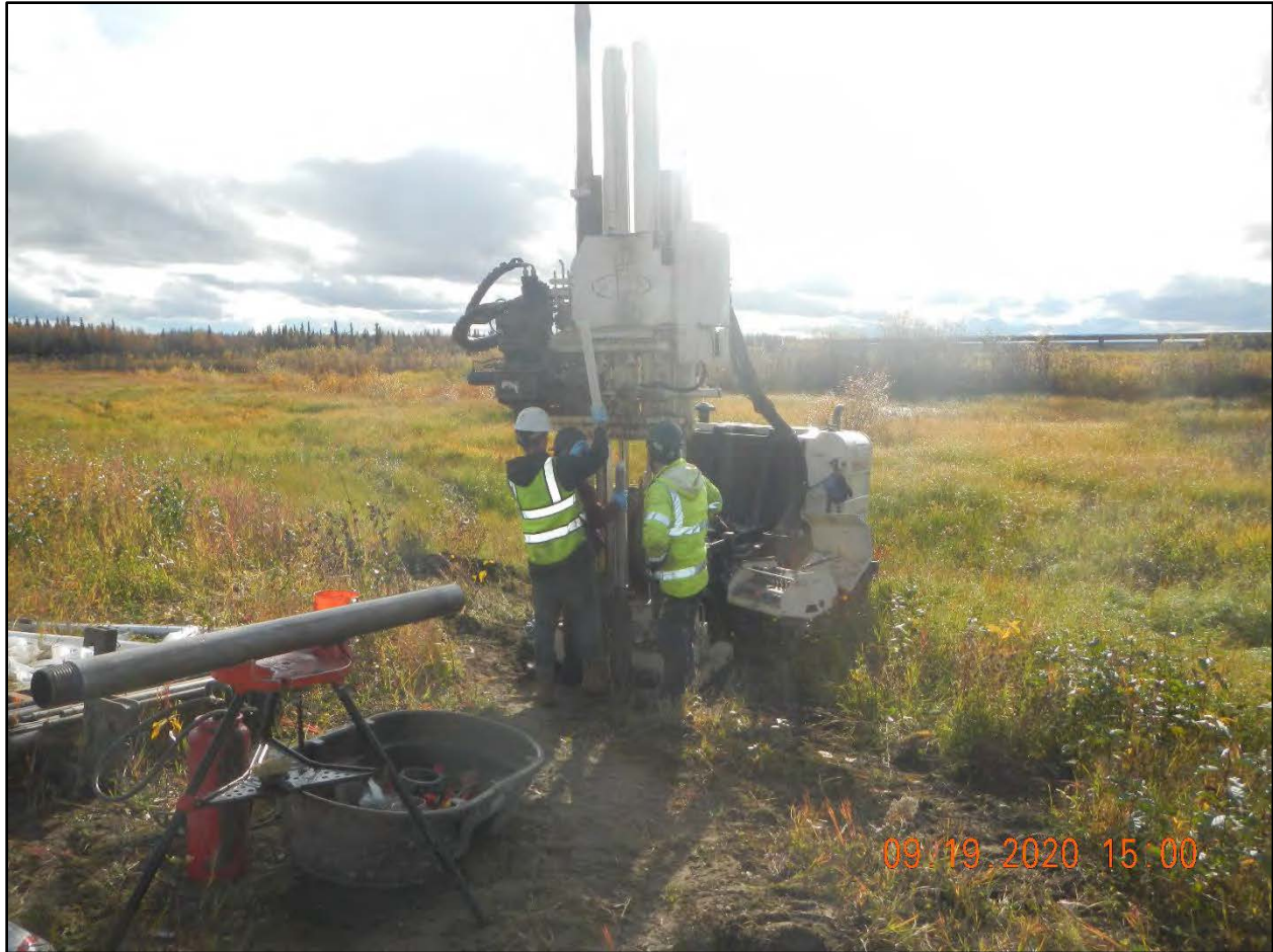
Photograph C.4-9. Installation of MW-23.
