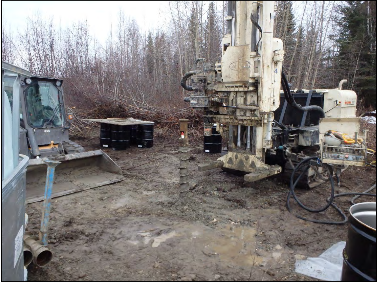
Photograph C.2-10. View of the installation of 19PS-MW01A.
