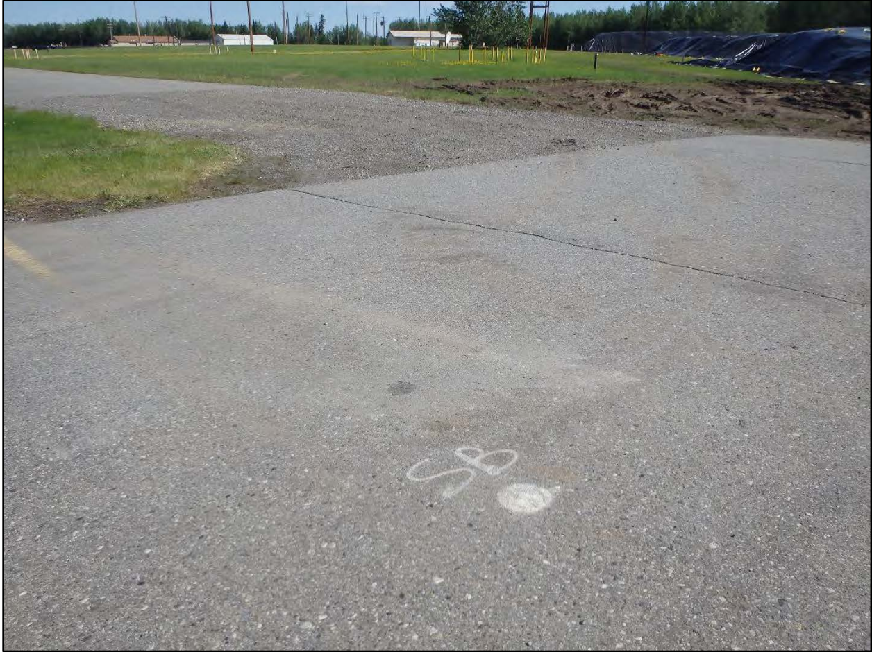
Photograph C.3-13. Asphalt patch for soil borings drilled through asphalt.
