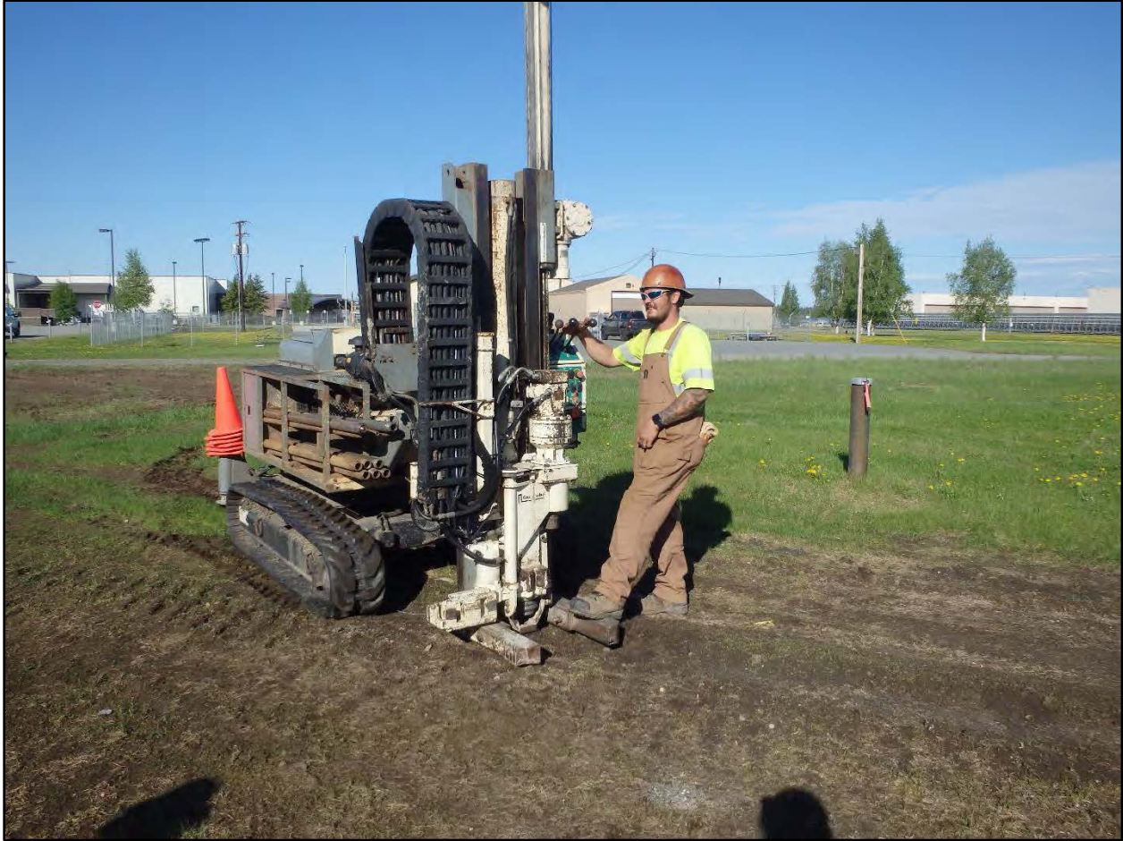
Photograph C.3-11. Drilling of 20PS-FFTA-ENT-SB11.
