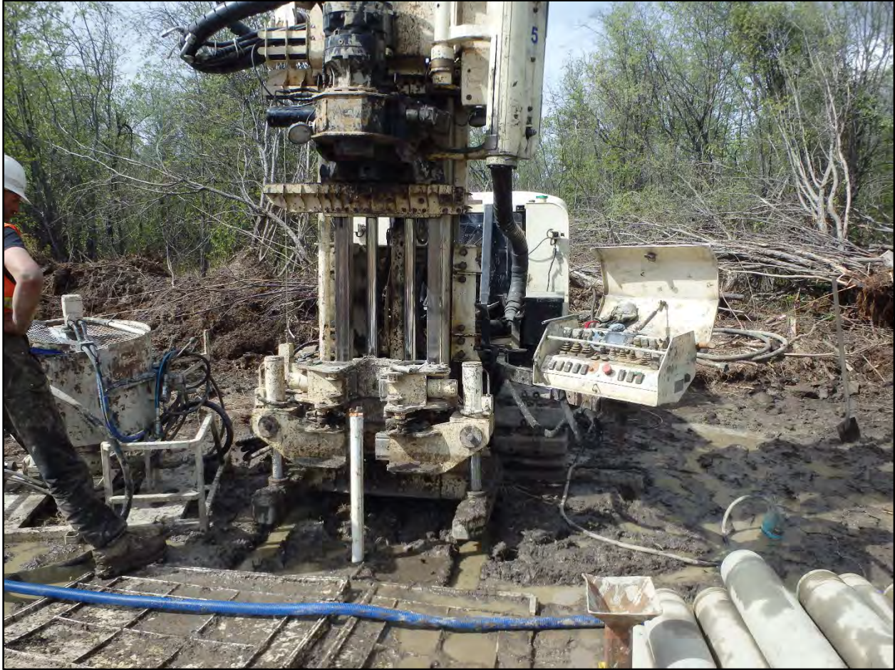
Photograph C.2-17. Installation of 20PS-MW02D.
