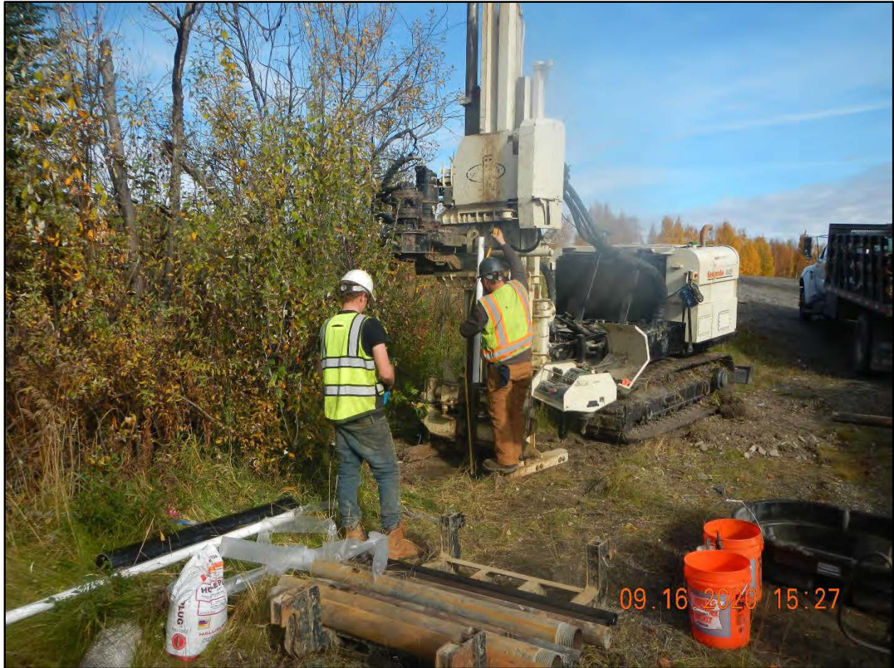
Photograph C.4-8. Setting Well MW-12.
