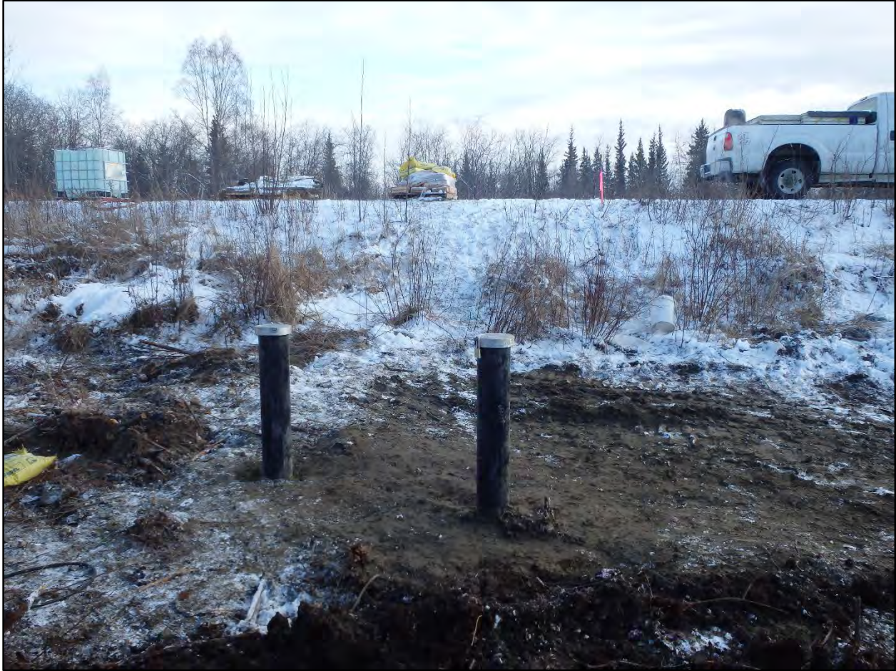
Photograph C.2-8. View of newly installed 19PS-MW02A and 19PS-MW02B.
