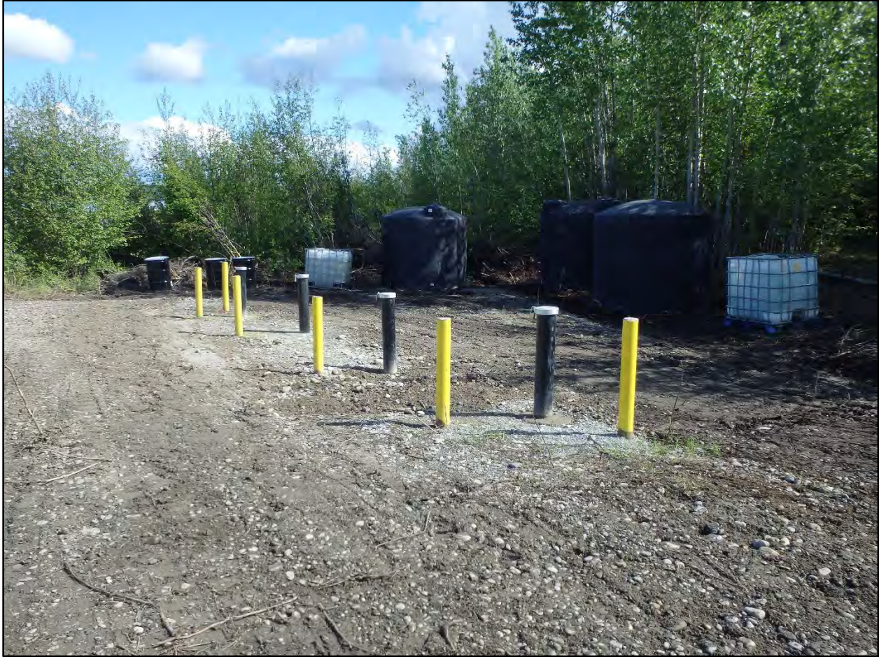
Photograph C.2-21. Well completions at Well Cluster #1.
