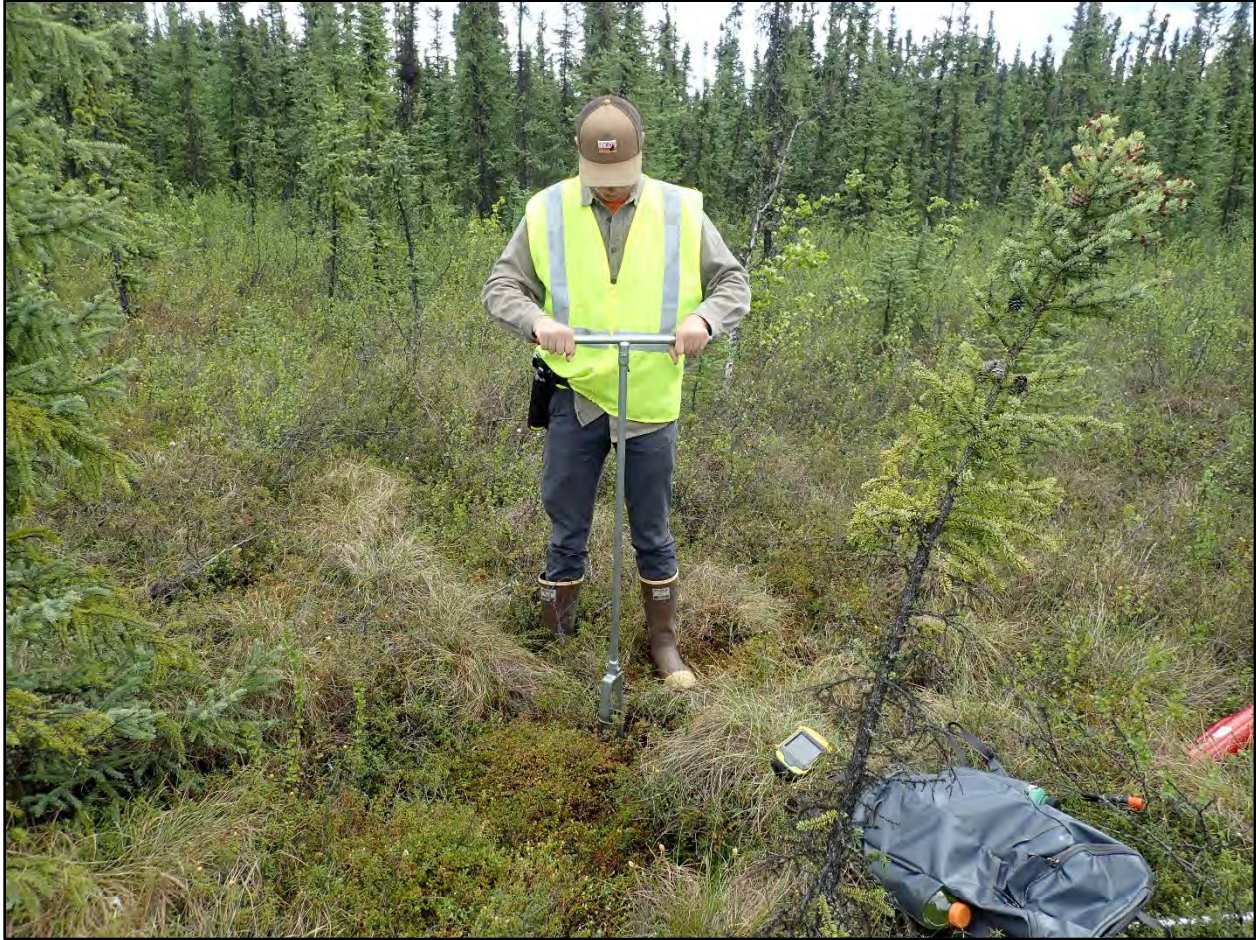
Photograph C.3-28. Attempt to install piezometer at TW43. Unable to penetrate frozen soil.
