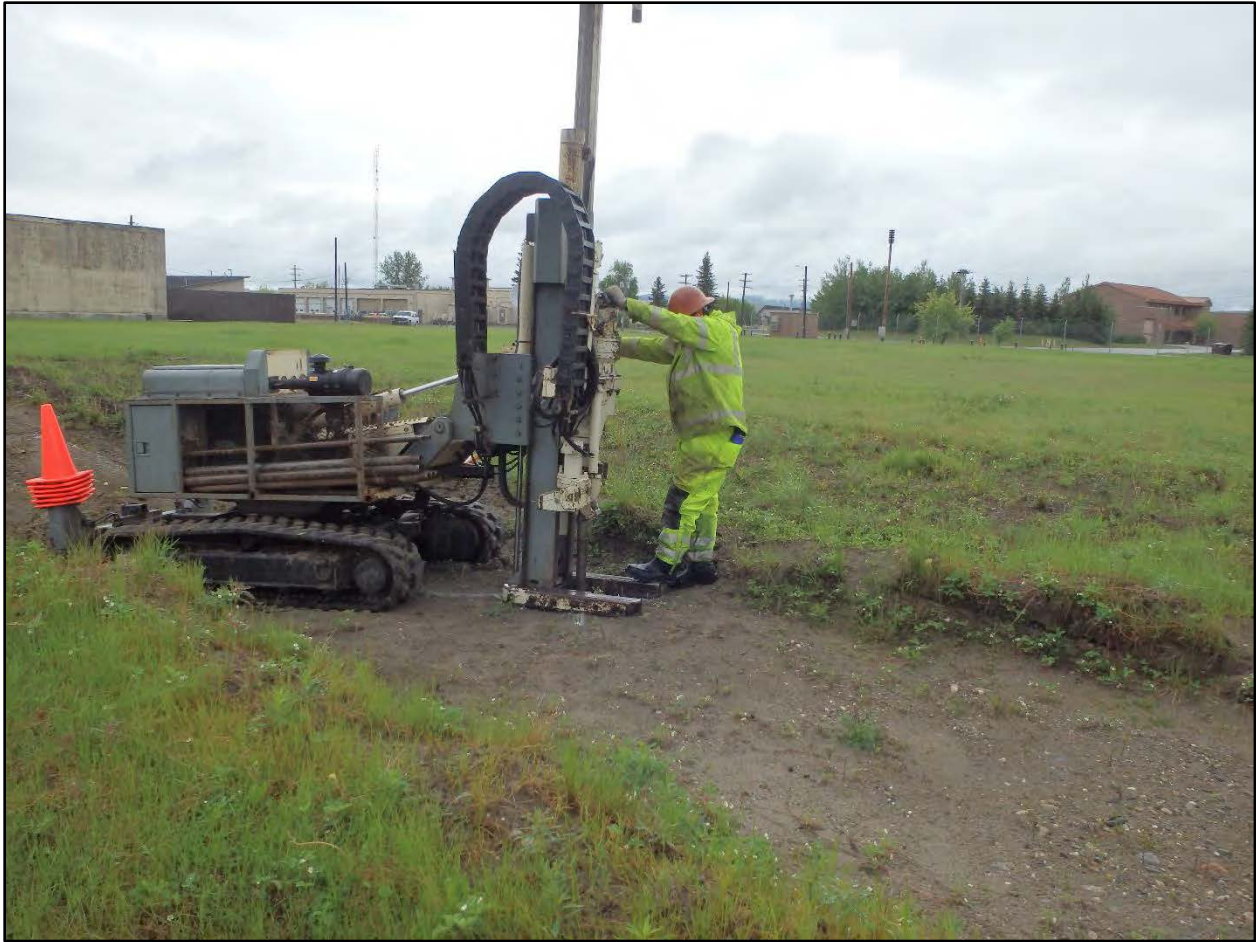
Photograph C.3-14. Drilling of 20PS-FST1-SB13.
