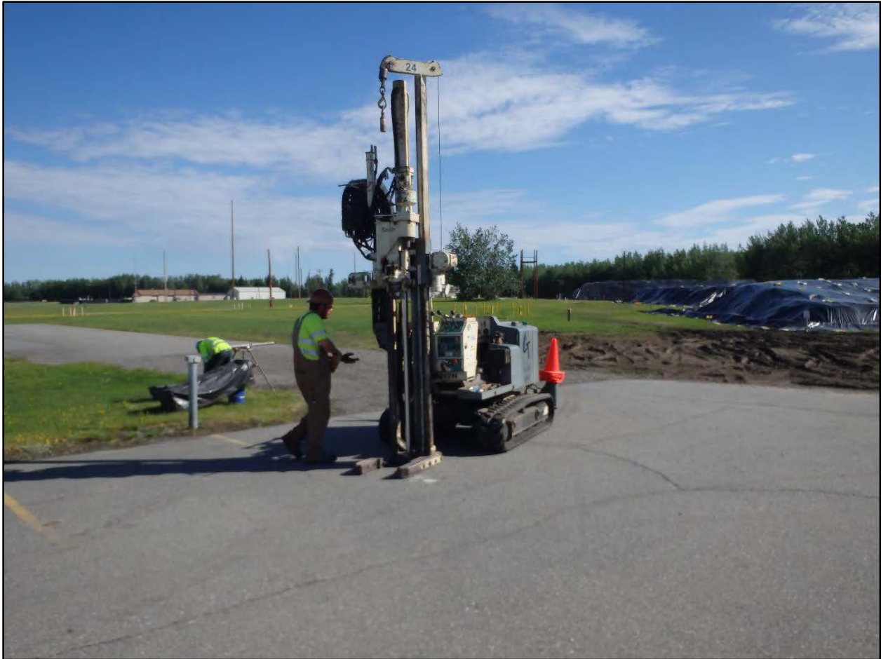
Photograph C.3-12. Drilling of 20PS-FFTA-ENT-SB14.
