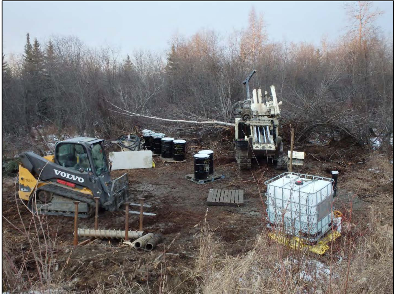
Photograph C.2-6. Overview of the drilling operation at 19PS-MW02B.
