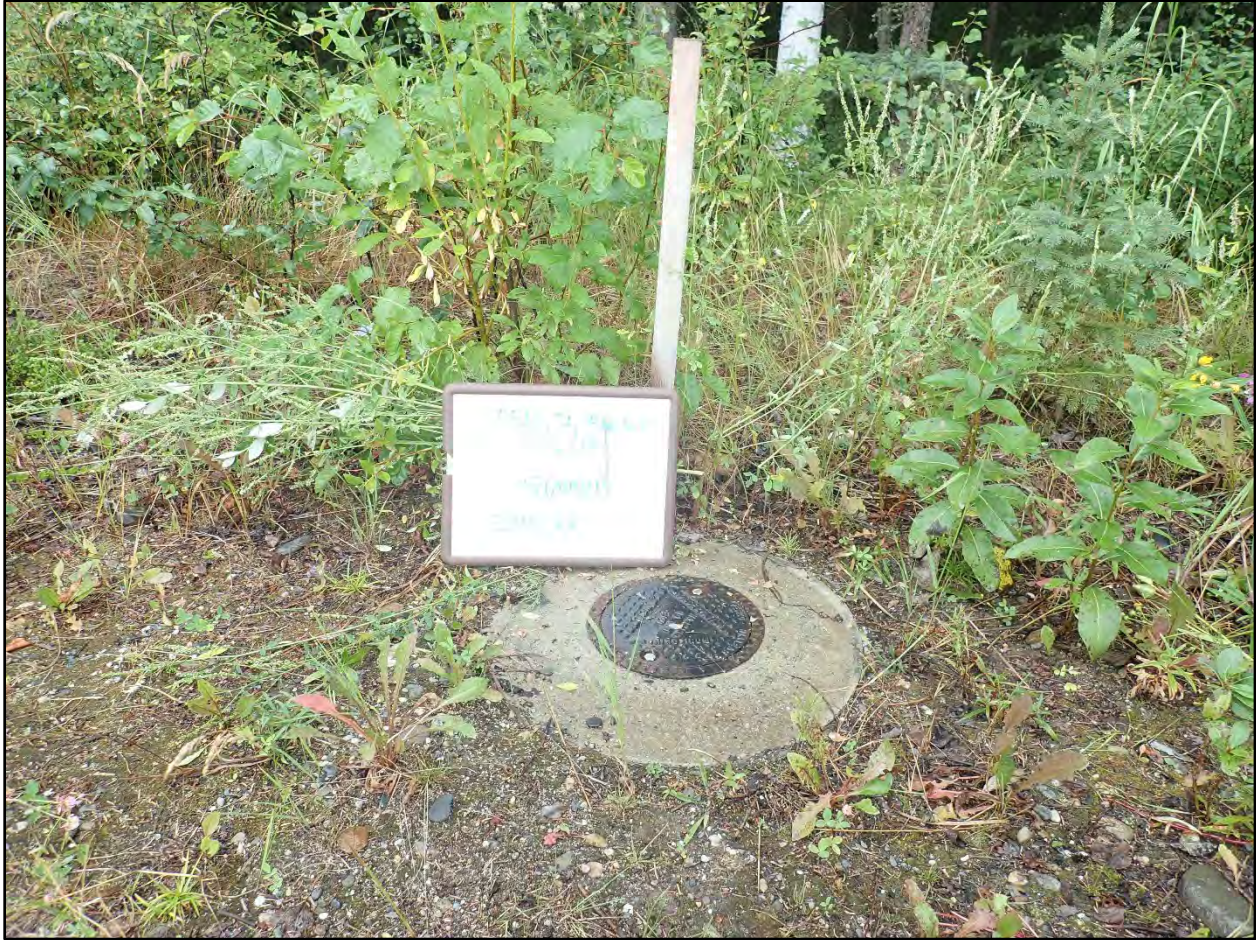
Photograph C.1-5. View of 51MB2B flush mount.
