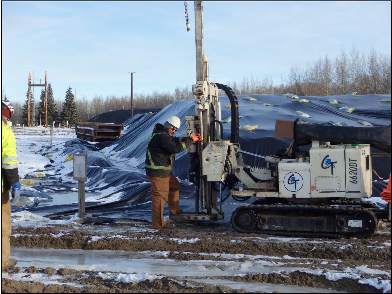
Photograph C.3-4. View of drilling of 19PS-FFTA-ENT-SB10.
