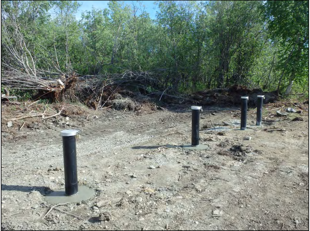
Photograph C.2-20. Well completions at Well Cluster #2.
