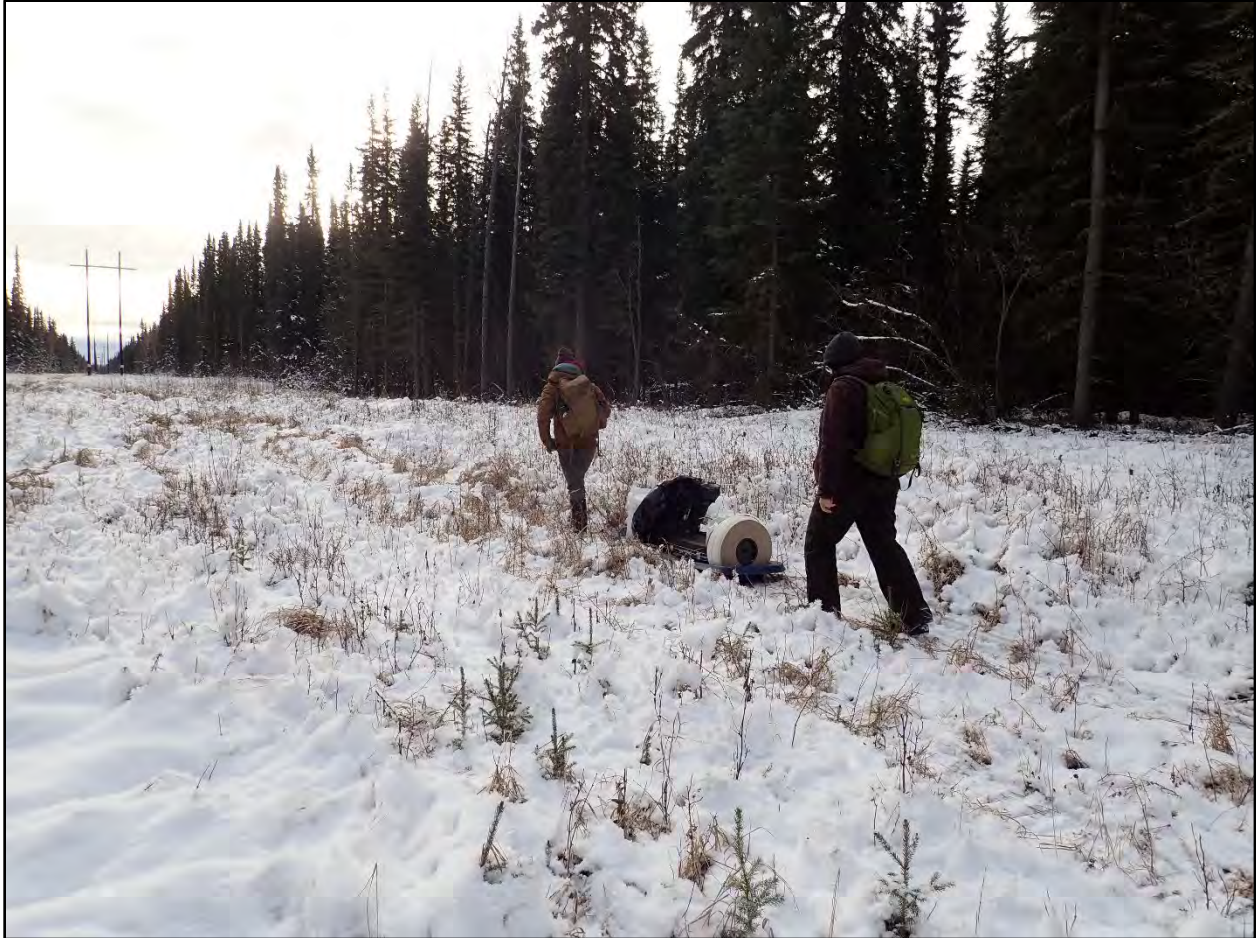
Photograph C.3-18. Drilling TW01 along DLA pipeline in Moose Creek.
