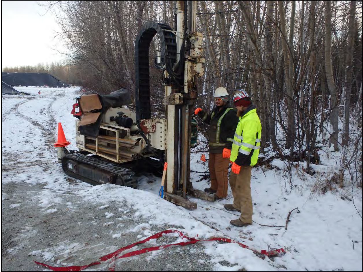
Photograph C.3-1. View of drilling of 19PS-FFTA-ENT-SB05.
