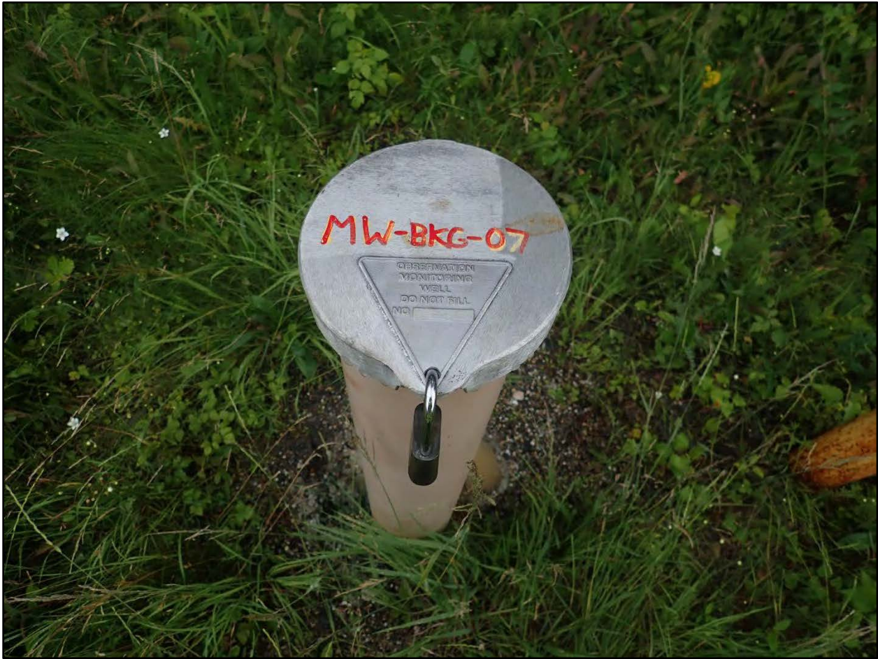
Photograph C.1-3. View of MW-BKG-07 with lid closed.
