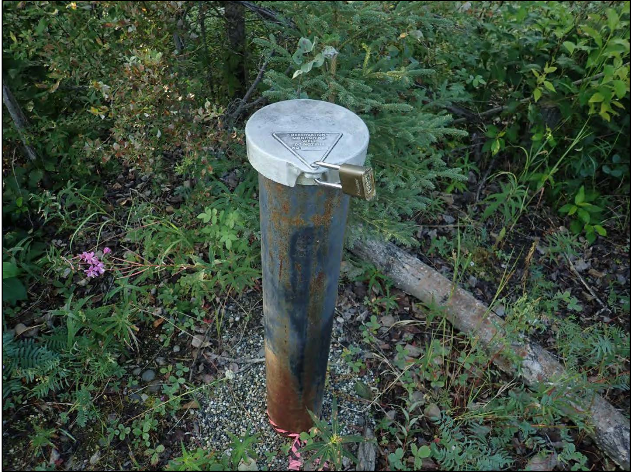
Photograph C.1-11. View of MW-BKG-10 with lid on.
