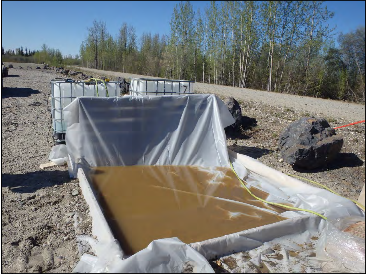
Photograph C.2-15. View of the decon pad for casing and rod cleaning.
