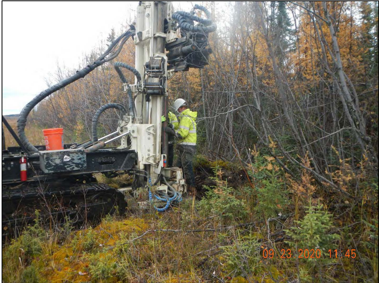
Photograph C.4-11. Drill rod connection during drilling.
