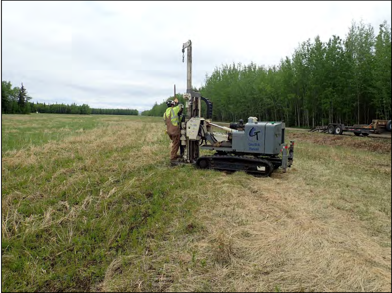
Photograph C.3-23. Geoprobe drill rig drilling TW46 in Chena Flood Control Project.
