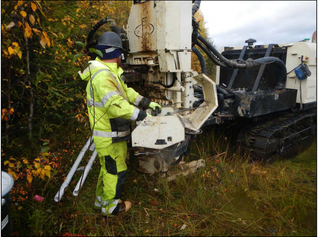
Photograph C.4-1. Drilling of MW-17.
