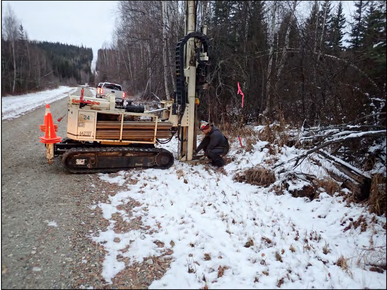
Photograph C.3-19. Setting SP-16 well screen at TW01.
