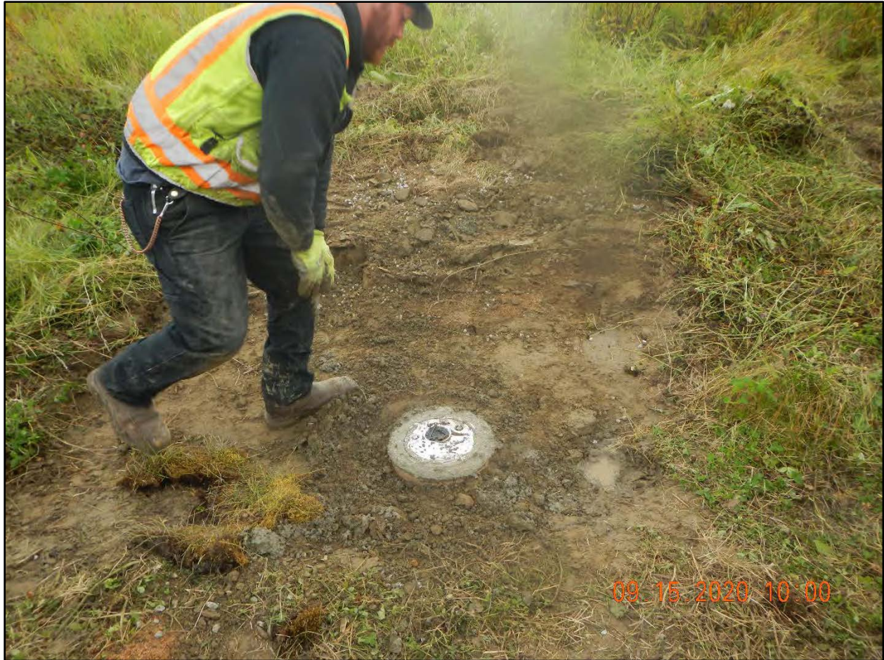
Photograph C.4-7. Pouring pea gravel as base for flush mount.
