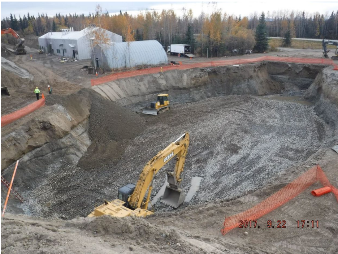
Burn Pit exvavation-2018
