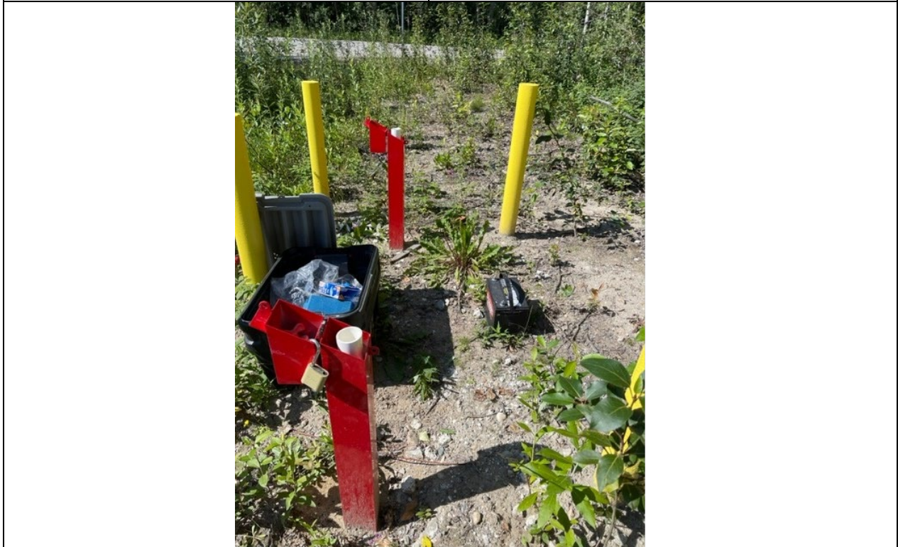
Photo No.: 016 Date/Time: 7/20/2024 @ 1303 Direction: South Description: Monitoring wells NPD-20 and NPD-40. Photo By: J. Blankenship
