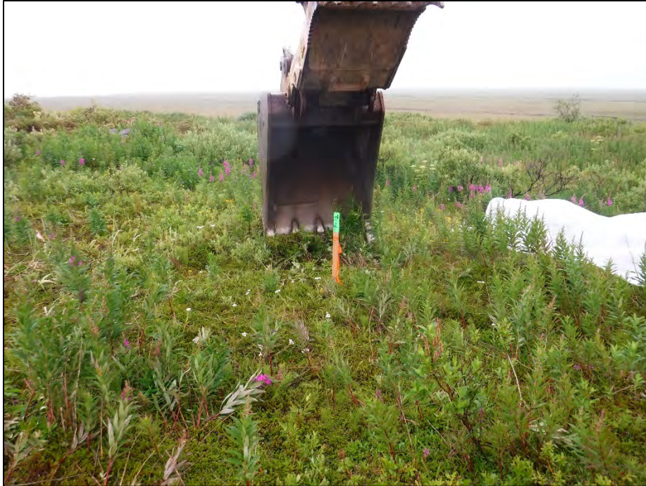
Photograph 63: TP-12 excavation location overview, facing northwest. 25 Jul 2018.
