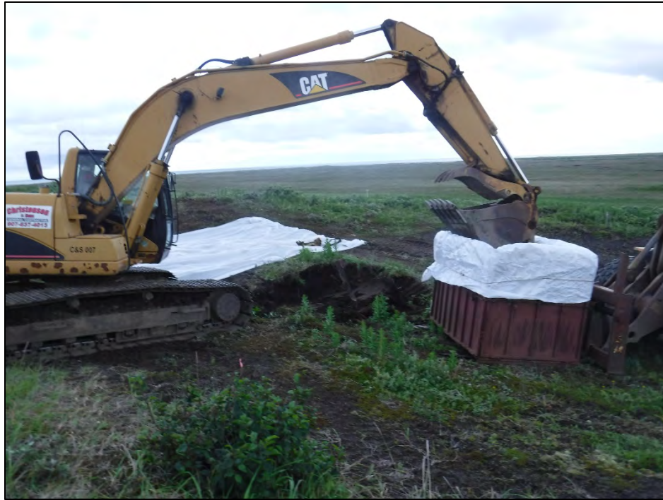
Photograph 29: TP-11 excavation and debris, facing west. 22 Jul 2018.
