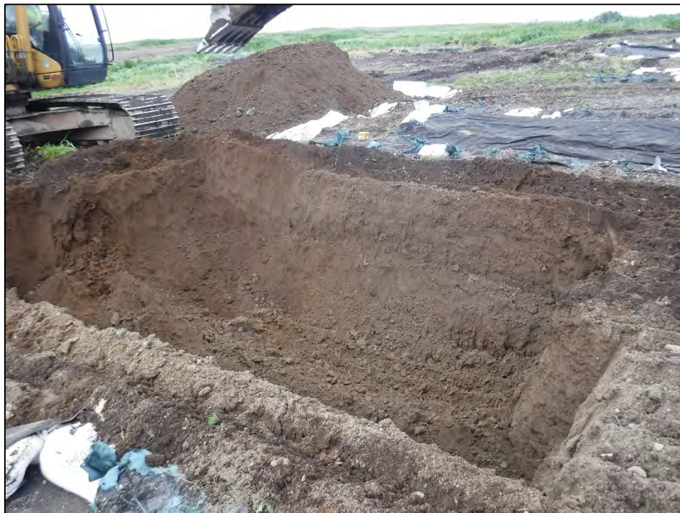
Photograph 50: TP-14 excavation, facing southwest. 23 Jul 2018.
