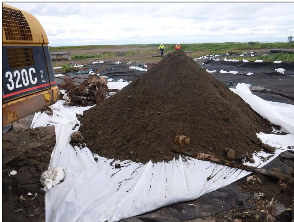
Photograph 40: TP-13B excavated debris, facing west. 22 Jul 2018.
