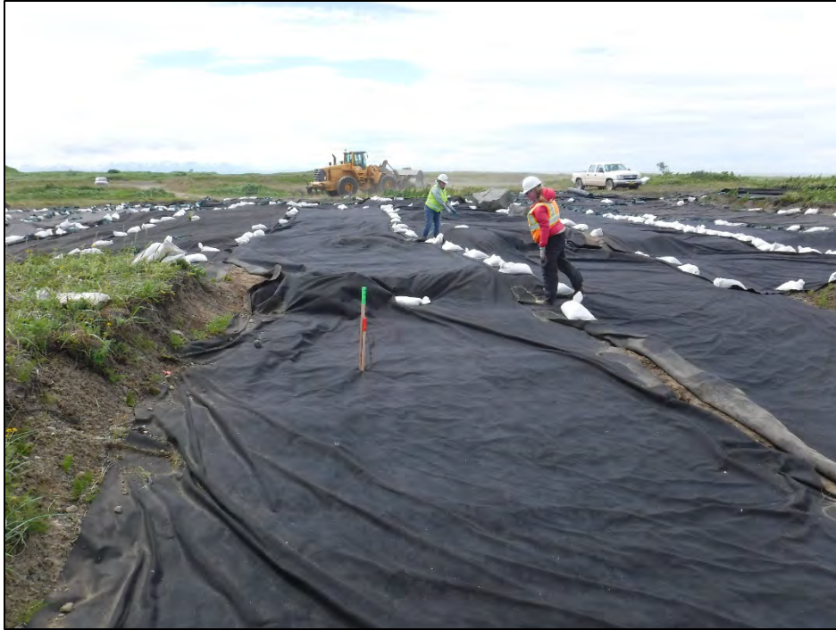
Photograph 5: Test Pit 10 reconnaissance and preparation, facing south. 18 Jul 2018.
