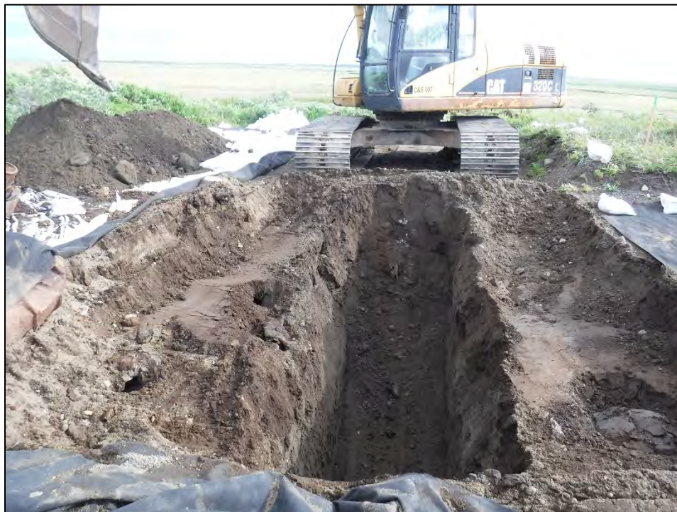
Photograph 8: TP-10 excavation finalization, facing northeast. 19 Jul 2018.
