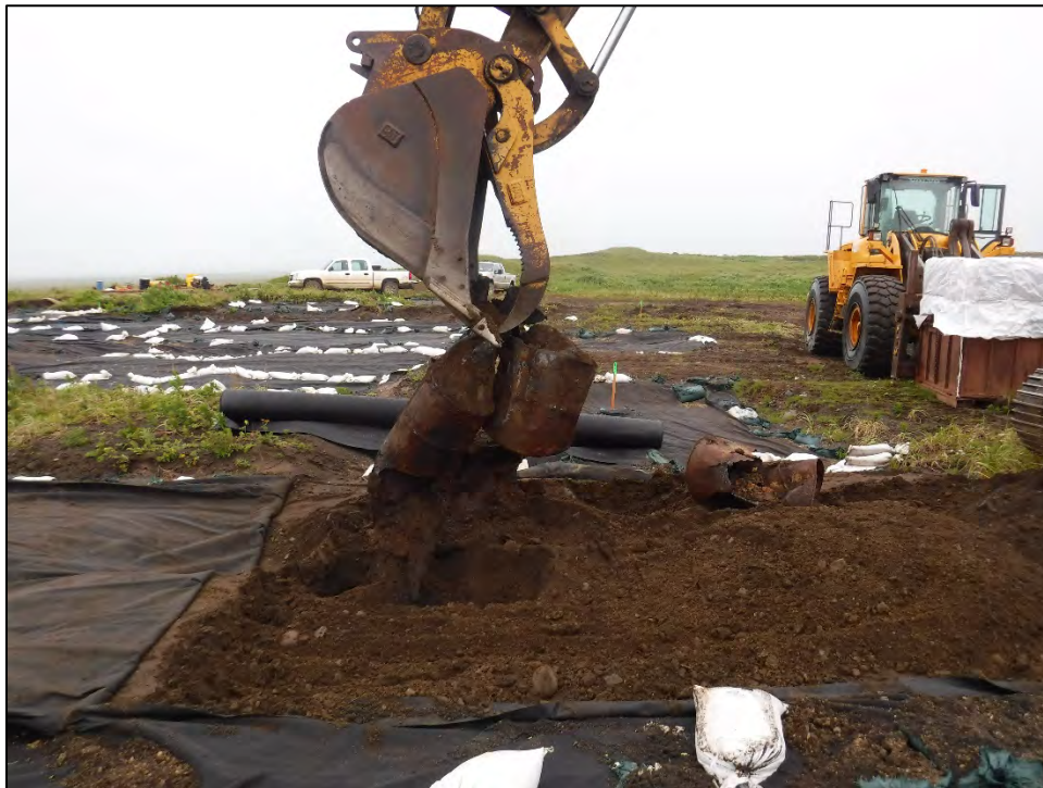
Photograph 46: TP-15 excavation and debris, facing east. 23 Jul 2018.
