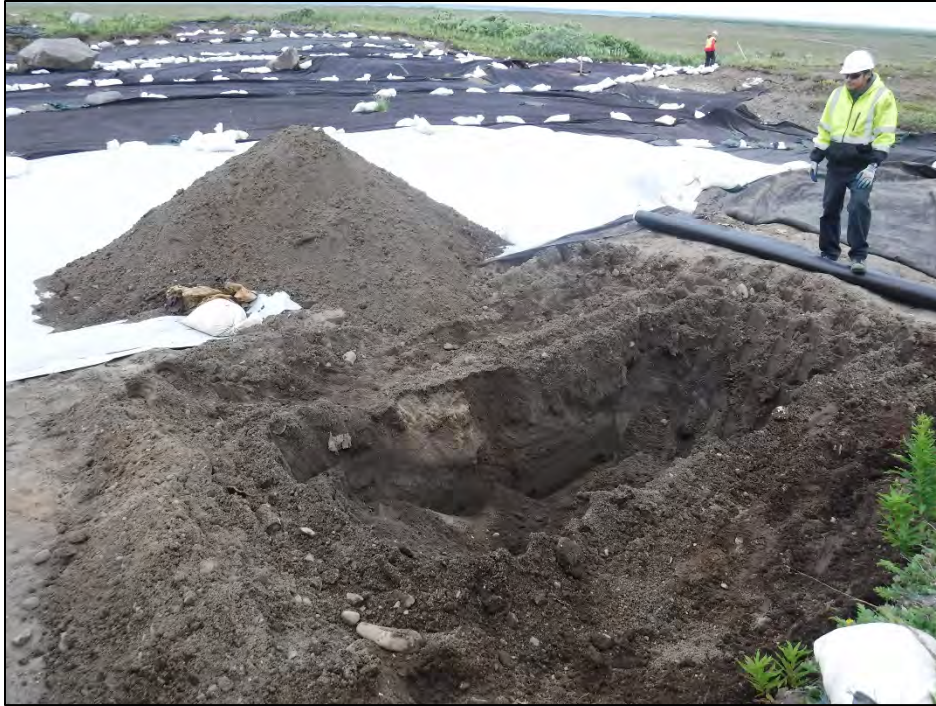
Photograph 37: TP-13A excavation finalization, facing northwest. 22 Jul 2018.
