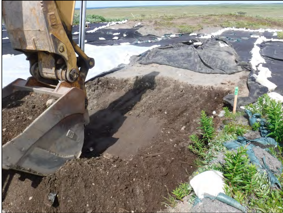
Photograph 35: TP-13A excavation location overview, facing north. 22 Jul 2018.
