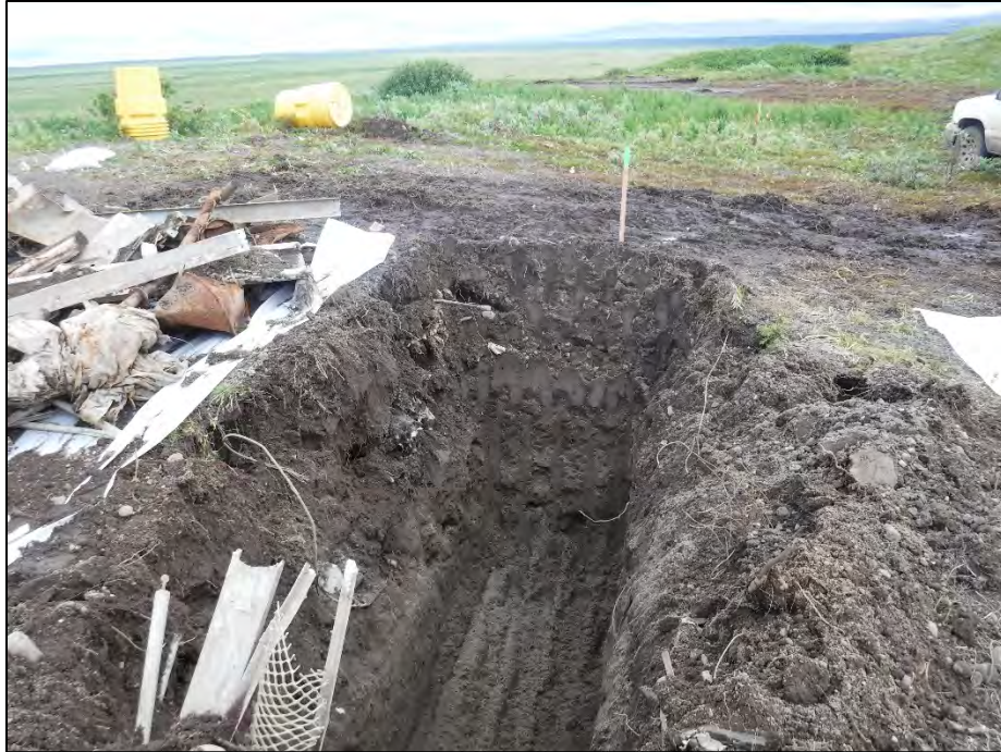
Photograph 59: TP-17 excavation finalization, facing east. 24 Jul 2018.
