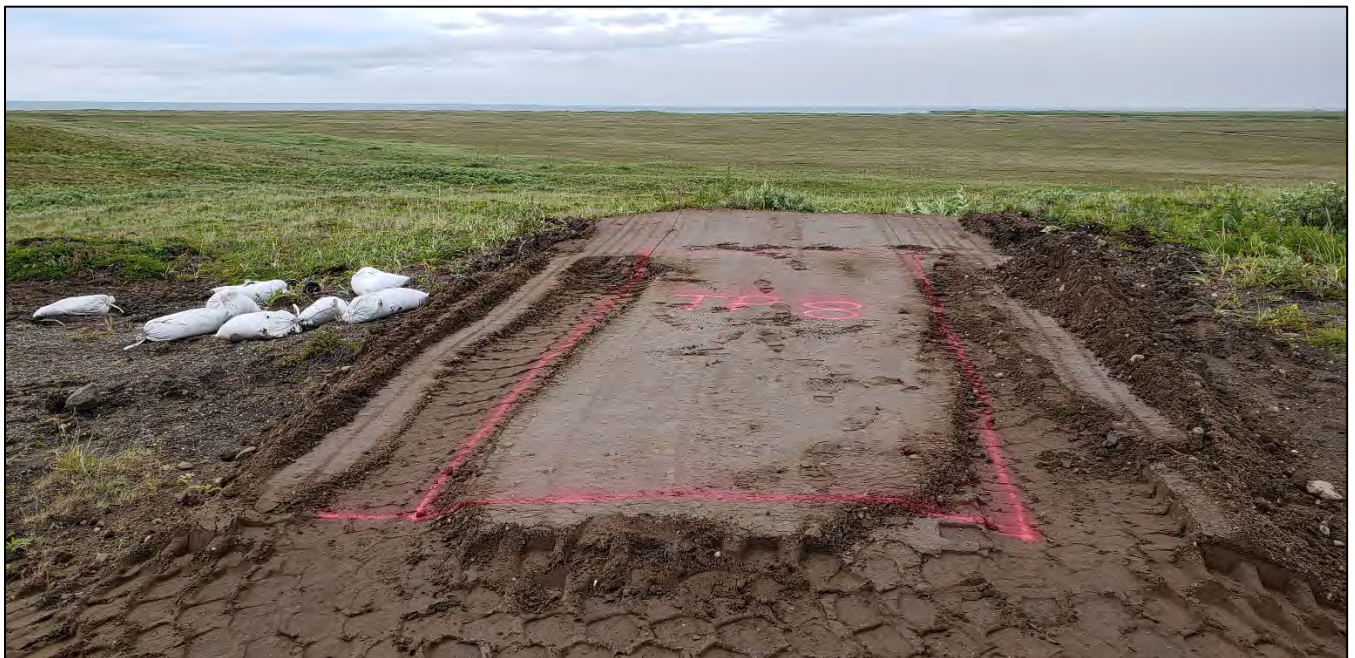
Photograph 22: TP-08 backfilled and marked for survey, facing north. 21 Jul 2018.
