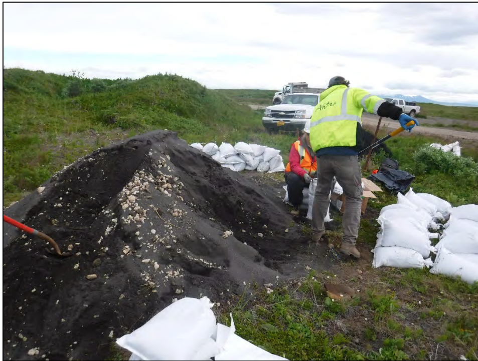
Photograph 16: Filling sandbags, facing south. 20 Jul 2018.
