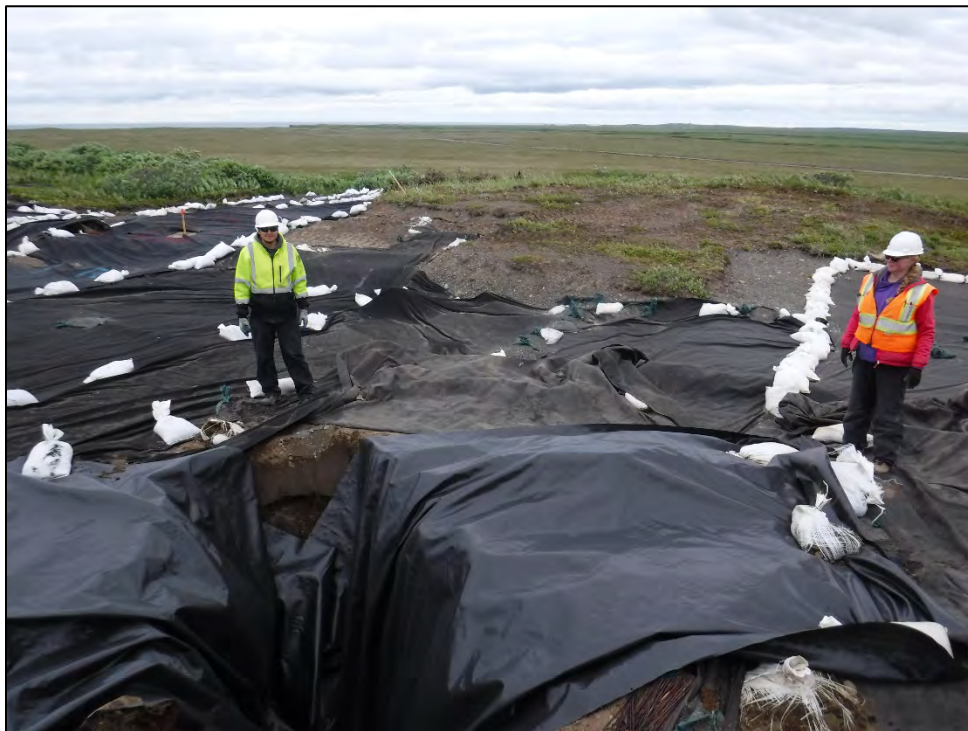
Photograph 42: TP-13B backfill preparation, facing north. 22 Jul 2018.
