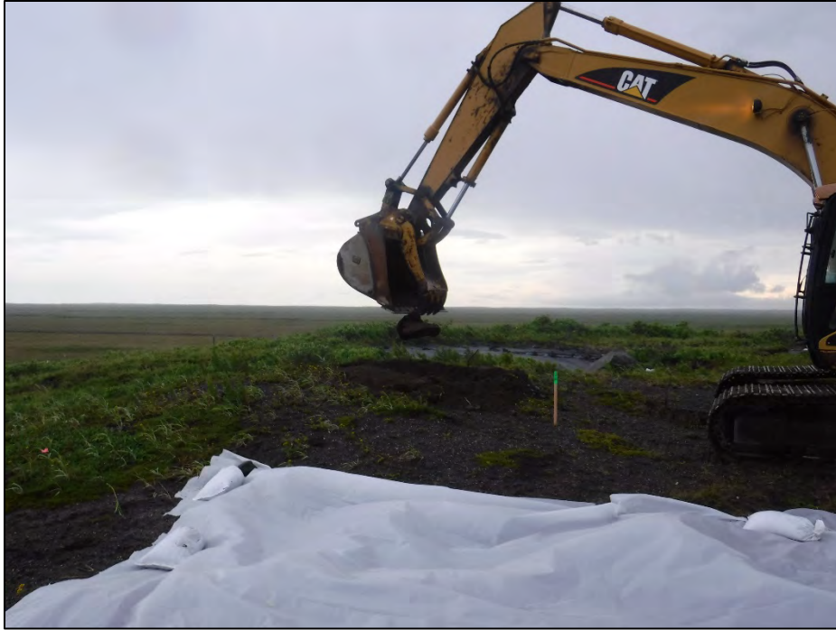
Photograph 19: TP-08 excavation and debris, facing north. 21 Jul 2018.
