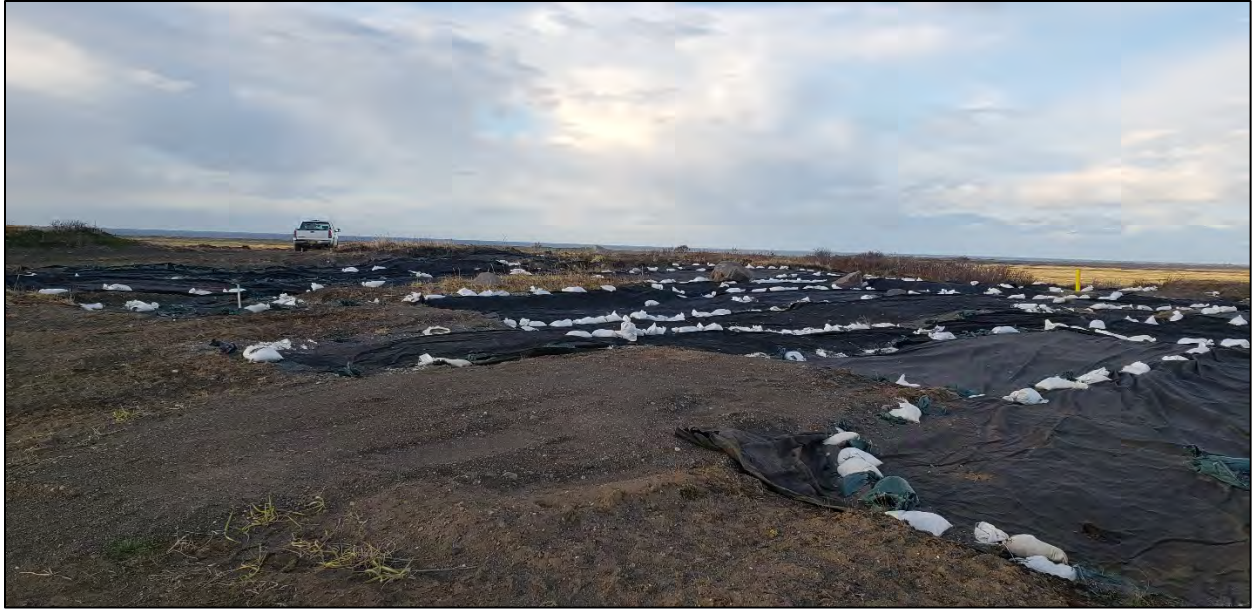
Photograph 77: Site overview after 2018 field work conclusion, facing northwest. 02 Nov 2018.
