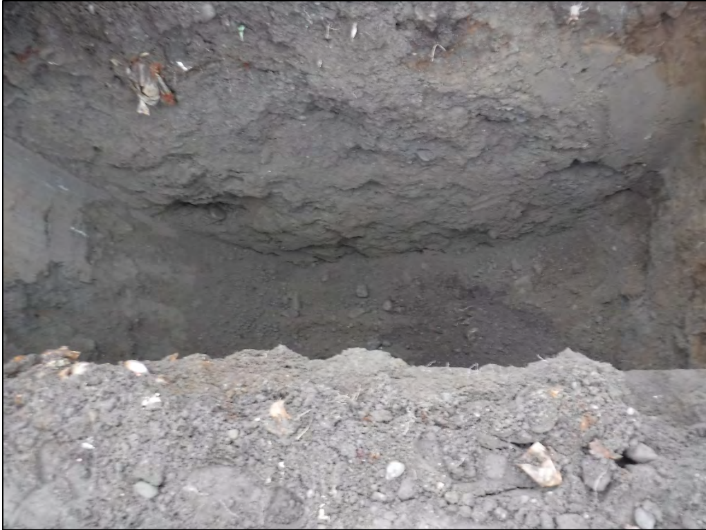
Photograph 25: Close-up of finalized excavation at TP-09. 21 Jul 2018.
