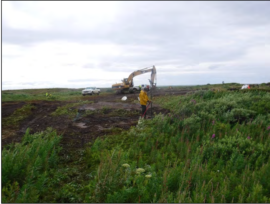
Photograph 69: Site survey in the foreground, equipment decontamination (right) and MW-06 well development (left) in the background. 26 Jul 2018.
