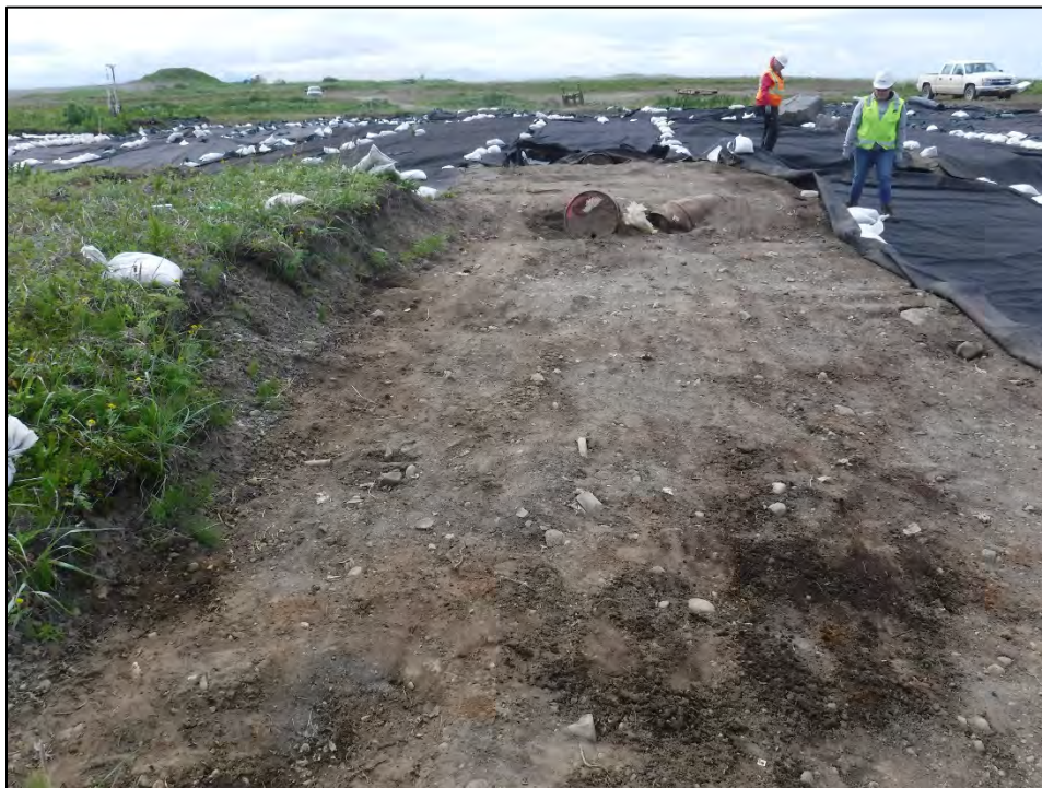
Photograph 6: TP-10 reconnaissance and preparation, facing south. 18 Jul 2018.
