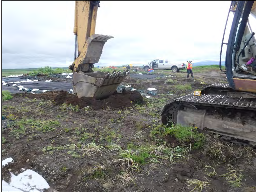
Photograph 49: TP-14 excavation location overview, facing northeast. 23 Jul 2018.
