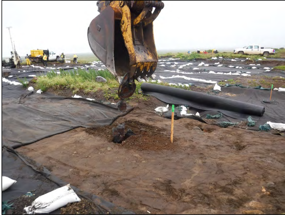
Photograph 45: TP-15 excavation location overview, with MW-10 installation in the background, facing north. 23 Jul 2018.
