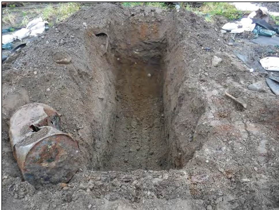
Photograph 48: Close-up of finalized excavation at TP-15. 23 Jul 2018.
