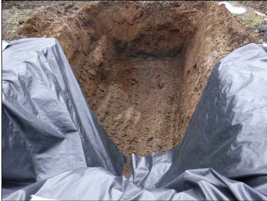
Photograph 51: Close-up of excavation finalization at TP-14. 23 Jul 2018.
