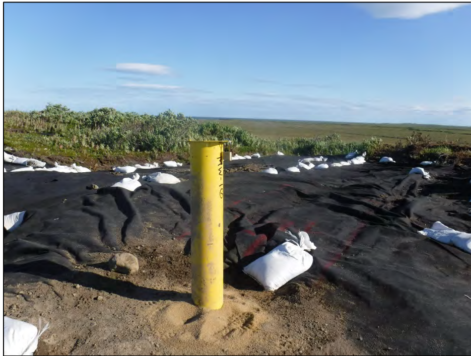
Photograph 76: MW-10 monument re-establishment. No water observed in well and no further well-development or sampling possible, facing north. 29 Jul 2018.
