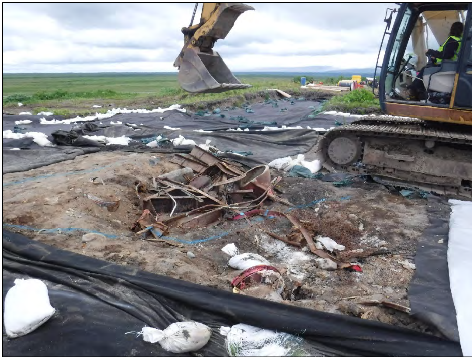
Photograph 38: TP-13B excavation location overview, facing northeast. 22 Jul 2018.
