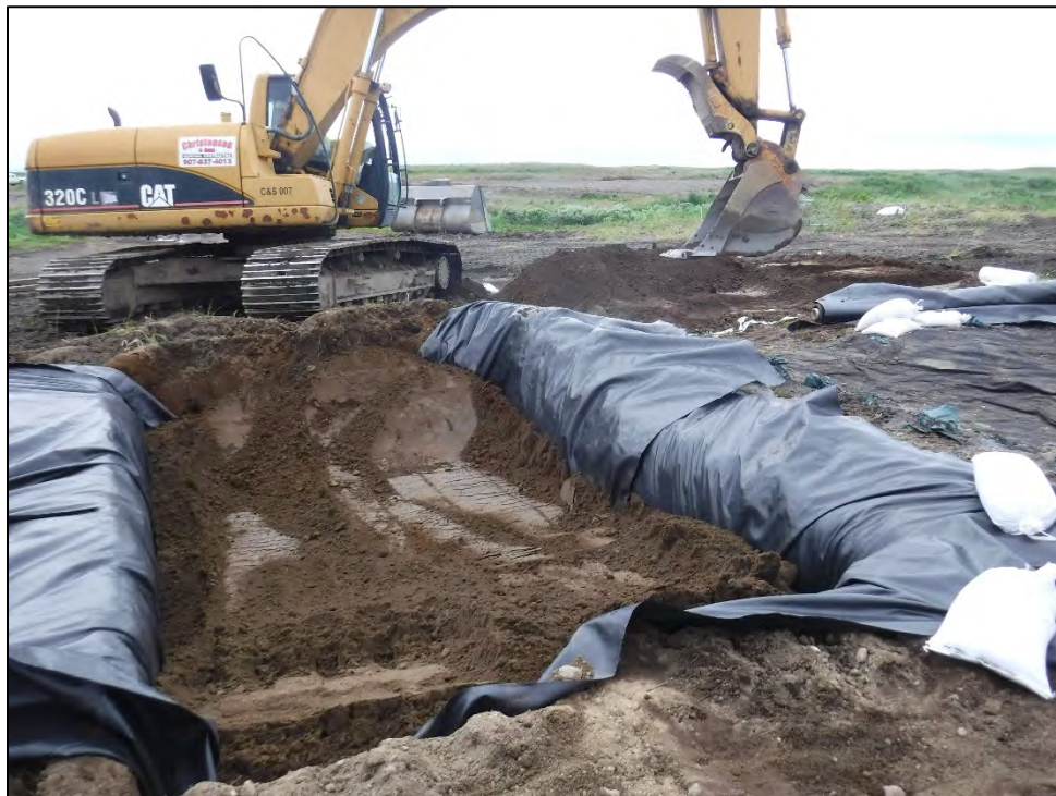
Photograph 52: Backfilling TP-14, facing south. 23 Jul 2018.
