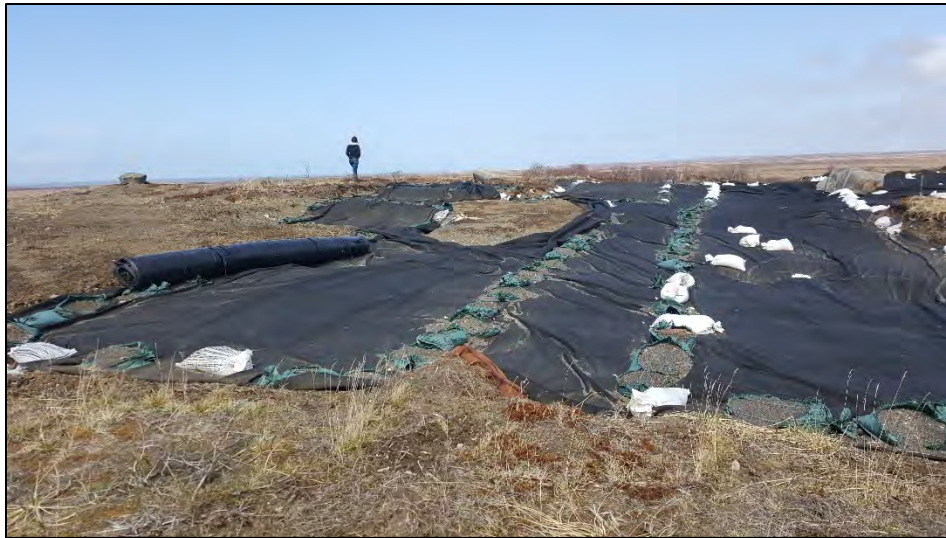
Photograph 1: Site reconnaissance, facing north. 01 May 2018.
