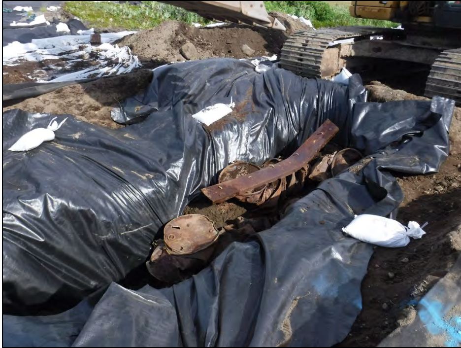
Photograph 11: Backfilling TP-10 with all debris segregated for co-location of MW-10, facing north. 19 Jul 2018.
