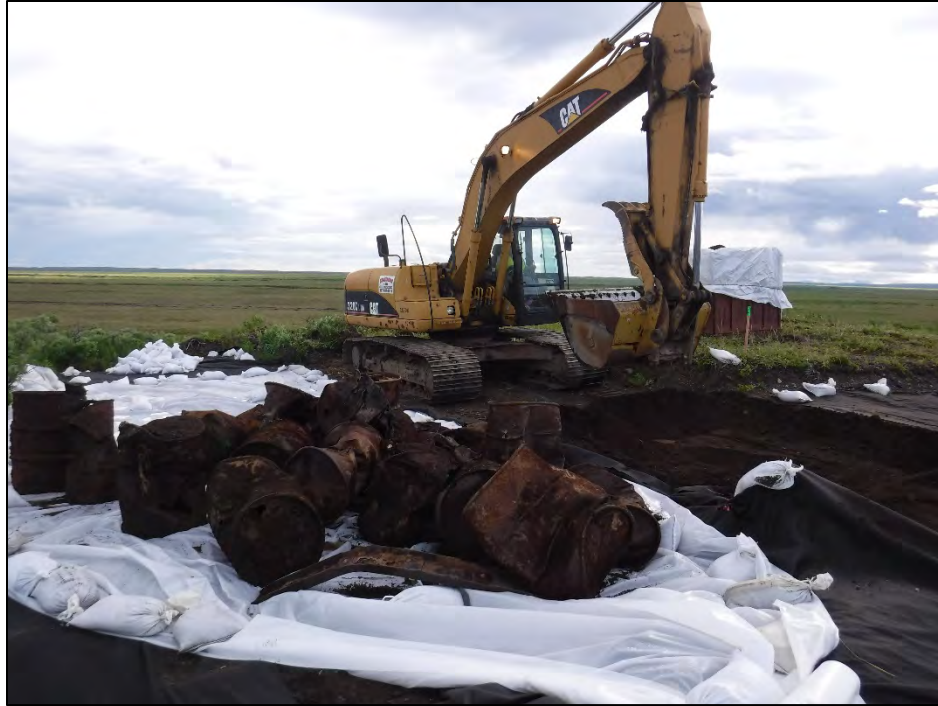
Photograph 7: TP-10 excavation and debris, facing northeast. 19 Jul 2018.
