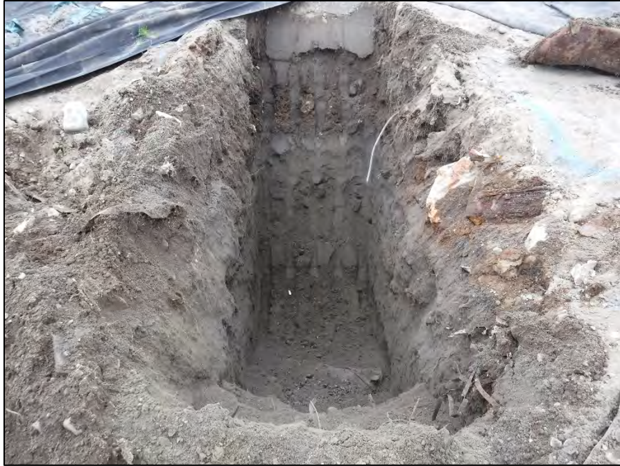
Photograph 41: Close-up of finalized excavation at TP-13B. 22 Jul 2018.
