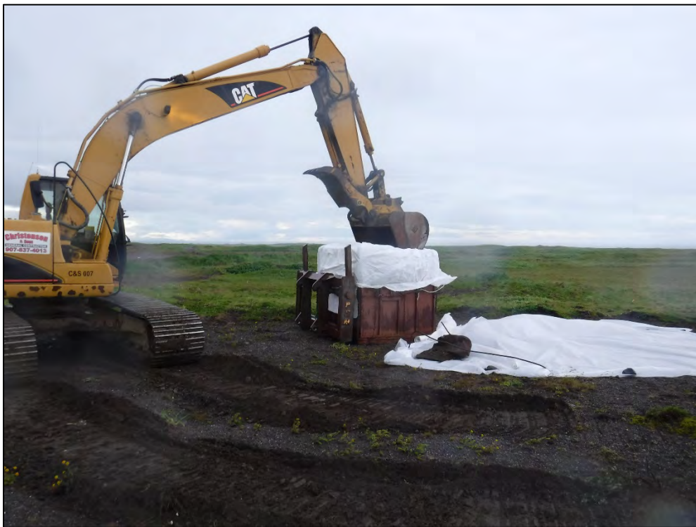
Photograph 20: TP-08 excavated debris, facing west. 21 Jul 2018.
