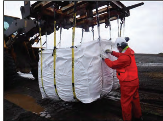
Figure 2: Supersack weighing at staging area. Profile view.
