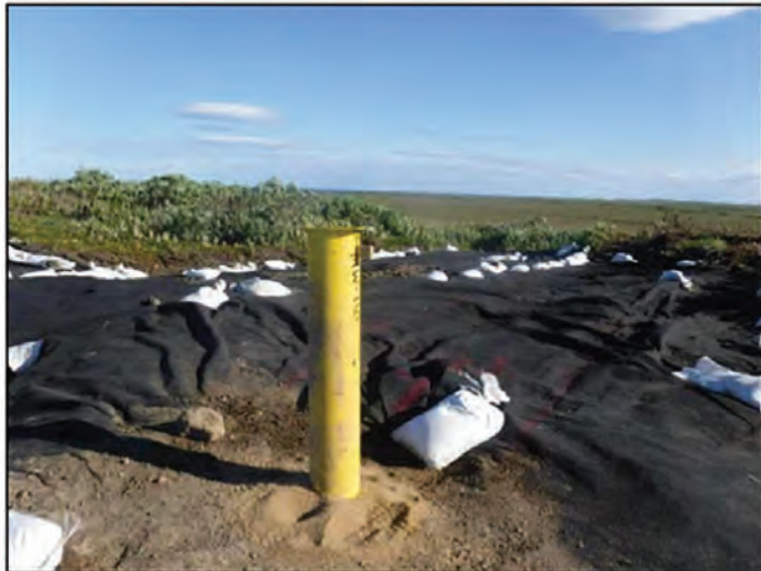
Figure 3: Monitoring Well NLF-MW-10 after monument installation rework. View NW.
