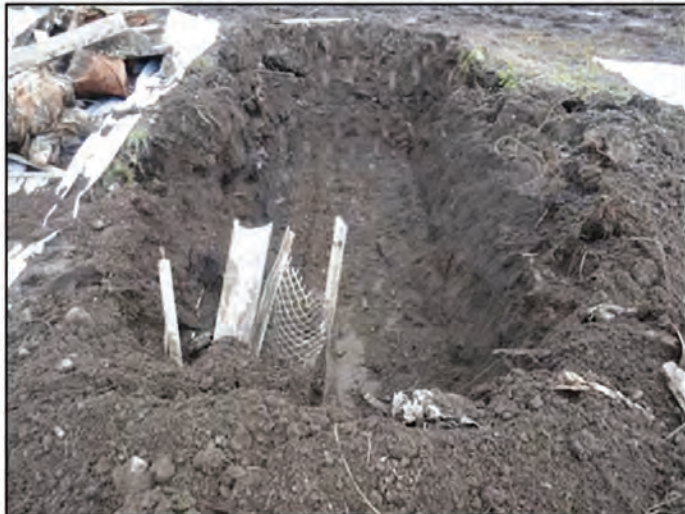
Figure 3: Excavation at NLF-TP-17. View NE.
