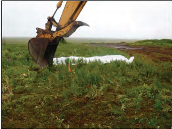
Figure 1: Potentially PCB bearing soil cap removal at NLF-TP-12. View N.
