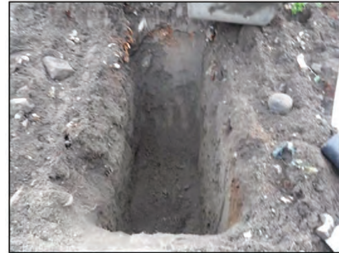
Figure 4: Testpit NLF-TP-09 excavation.
