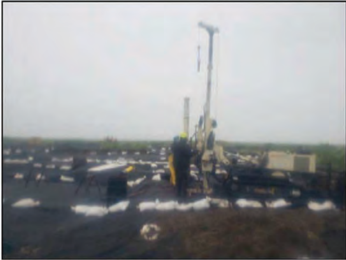
Figure 5: Drilling SB-10. View SW.
