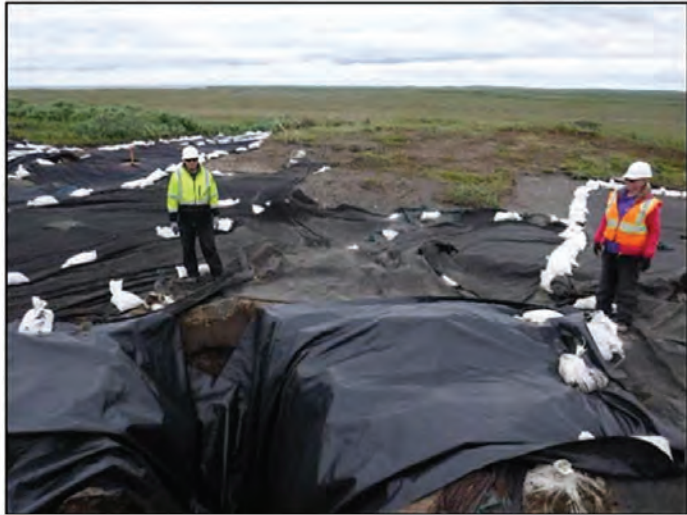
Figure 5: Backfilling NLF-TP-13. View S.
