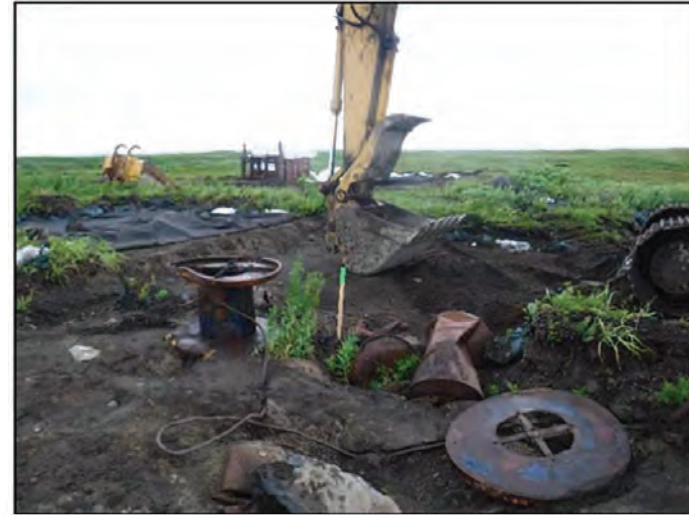
Figure 2: Testpit NLF-TP-09 activities. View NW.
