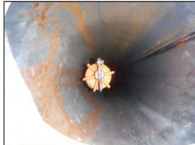
Figure 4: Monitoring Well NLF-MW-10 view inside of reworked monument.
