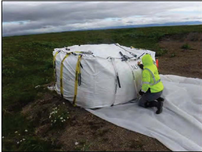
Figure 5: PCB waste labeling at staging area.
