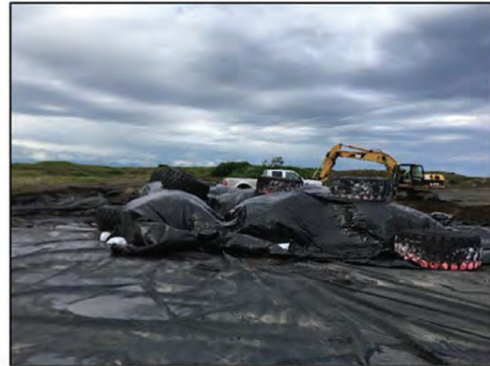
Figure 2: Supersacks covered with lining for weather protection.
