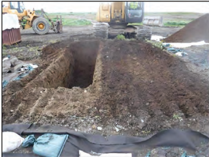
Figure 3: Excavation at NLF-TP-14. Expansion to W. View S.
