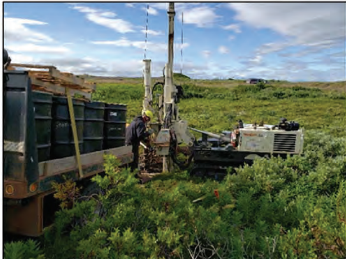
Figure 7: Drilling NLF-SB-06. View E.
