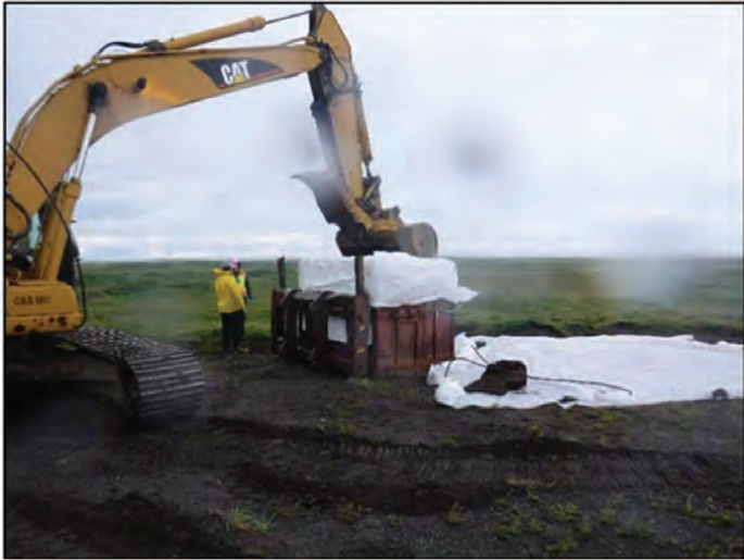
Figure 1: Testpit NLF-TP-08 activities. View NW.
