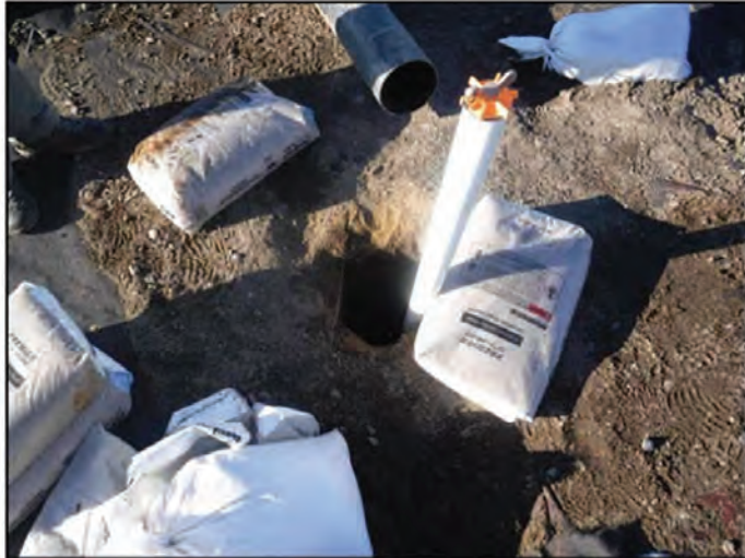
Figure 1: NLF-MW-10 and sandbags for monument installation rework.
