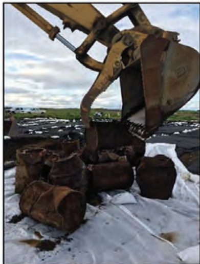
Figure 3: NLF-TP-10 contents (drums). View SW.
