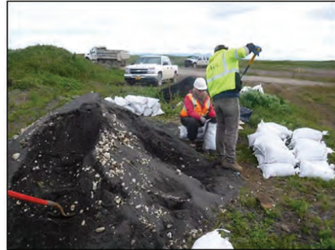
Figure 6: Making sand bags. View E.
