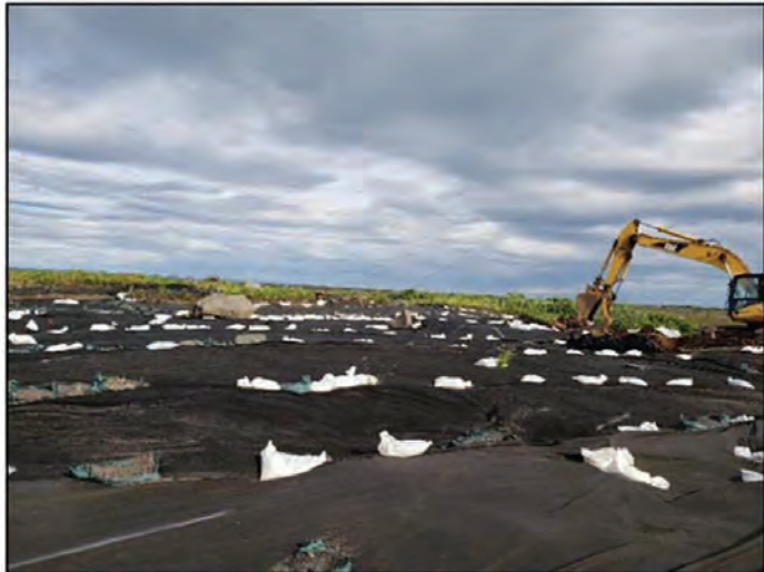
Figure 1: North Landfill Overview, starting Test-Pit NLF-TP-10. View SW.
