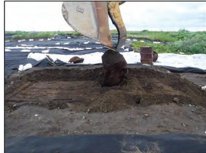
Figure 2: Excavator picking drum from North Landfill. View SW.
