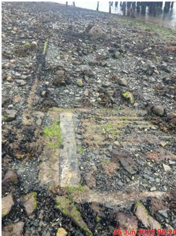
Photograph 30: Concrete vault and associated pipe. View West. 6/25/2025.
