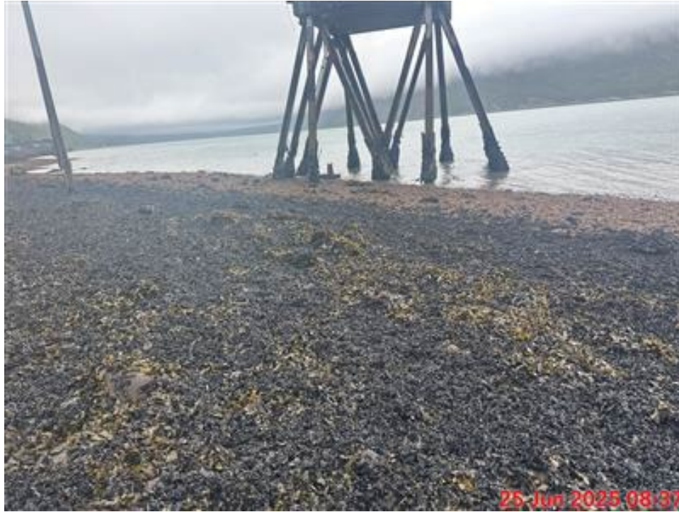
Photograph 37: Seafloor near the North Dolphin. View Northwest. 6/25/2025.
