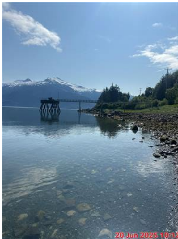
Photograph 2: South Dolphin. View East. 6/20/2025.
