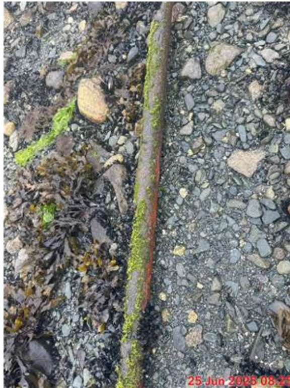
Photograph 32: Pipe running to concrete vault. View Down. 6/25/2025.
