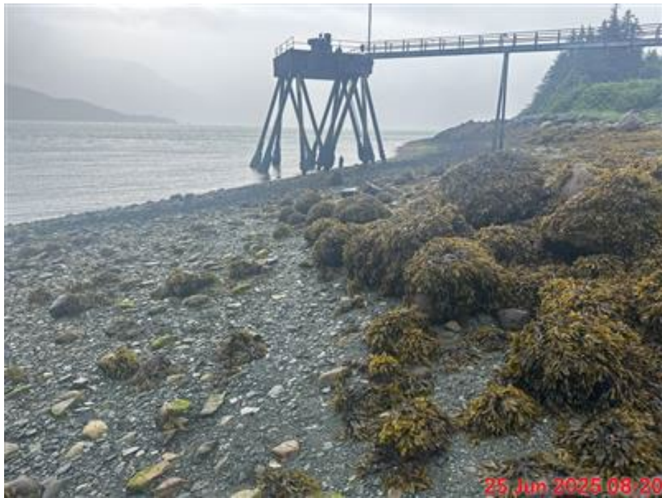
Photograph 26: South Dolphin at low tide. View Northeast. 6/25/2025.
