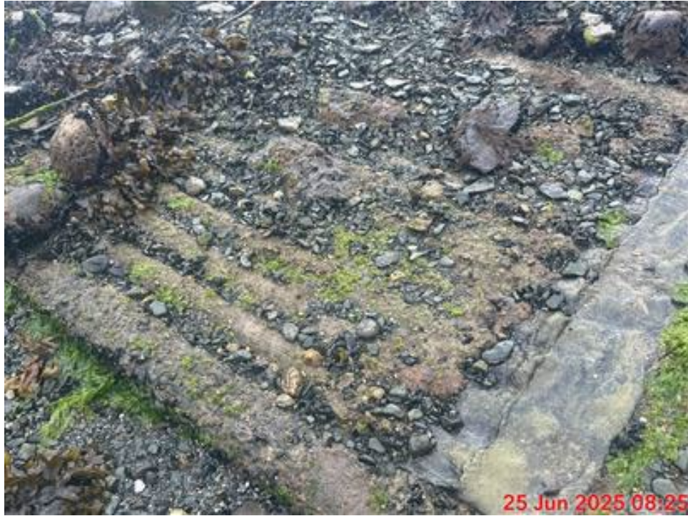
Photograph 31: Concrete vault. View Down. 6/25/2025.
