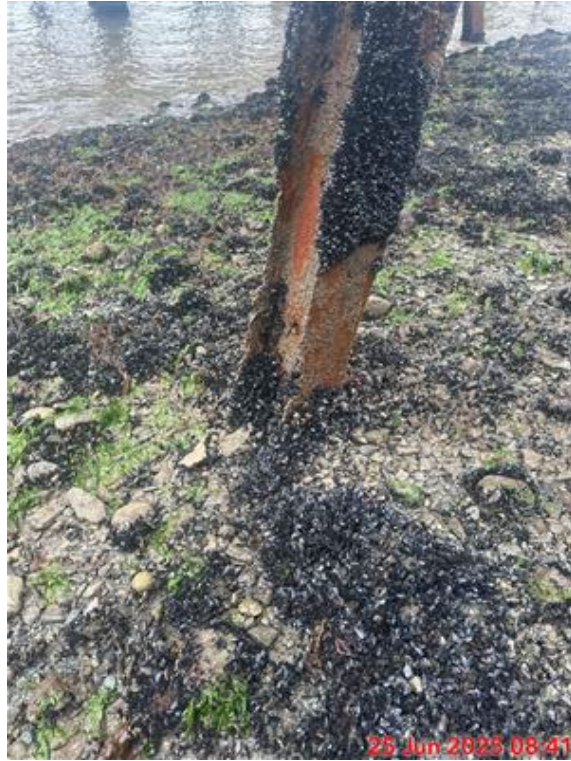
Photograph 41: Leg of HFT Dock. View Northeast. 6/25/2025.
