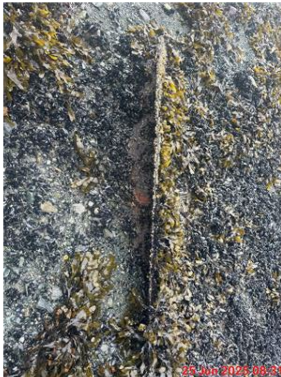
Photograph 34: Metal debris under HFT Dock. View Down. 6/25/2025.
