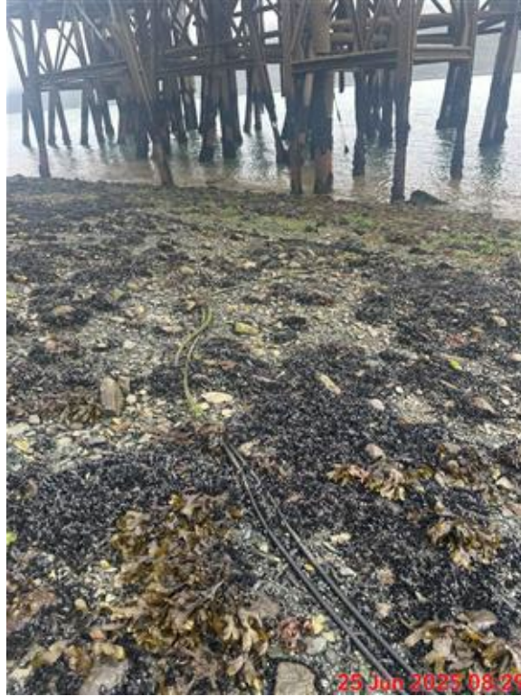
Photograph 33: Seafloor and wires near HFT dock. View Northwest. 6/25/2025.
