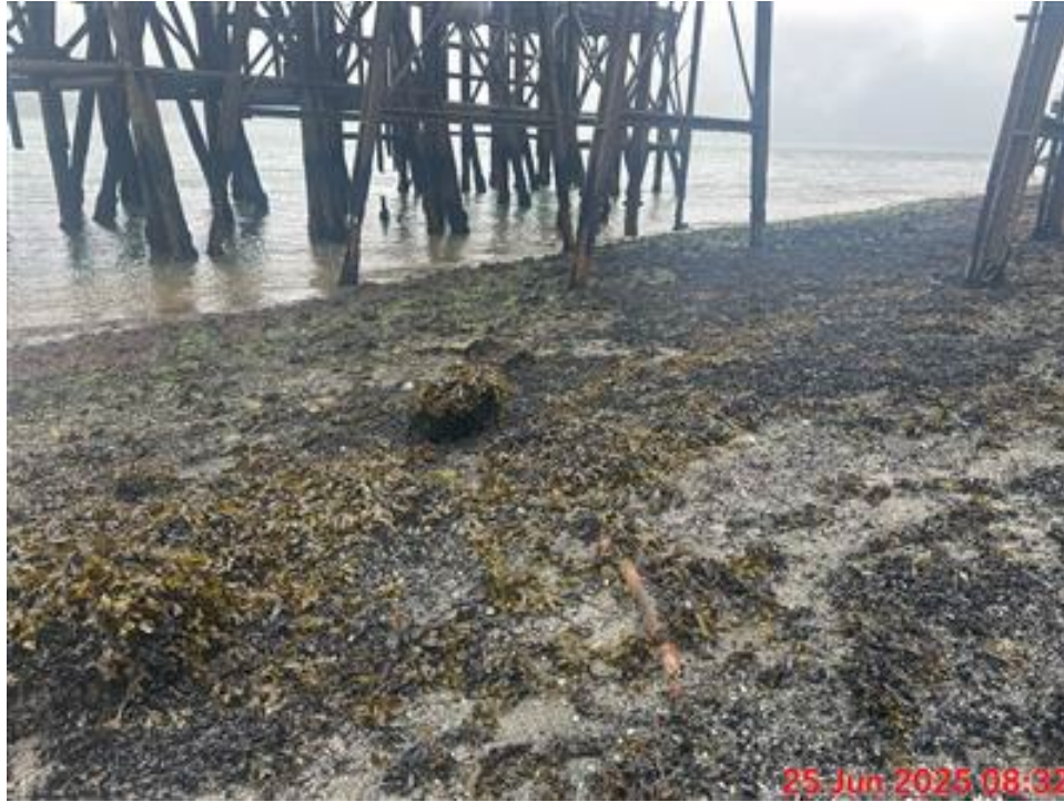
Photograph 35: Seafloor under HFT Dock. View Northeast. 6/25/2025.
