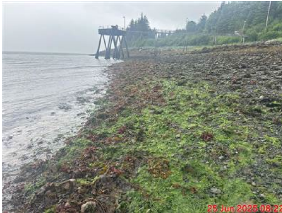
Photograph 28: Seafloor between HFT Dock and South Dolphin. View East. 6/25/2025.
