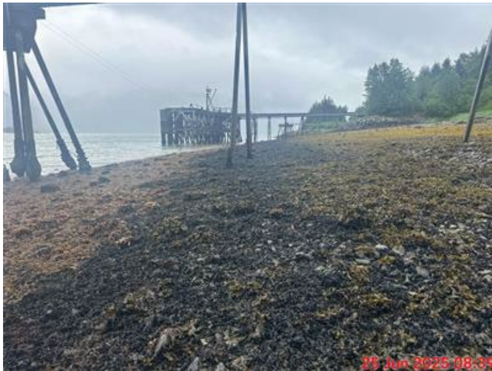
Photograph 40: HFT Dock area viewed from North Dolphin. View East. 6/25/2025.
