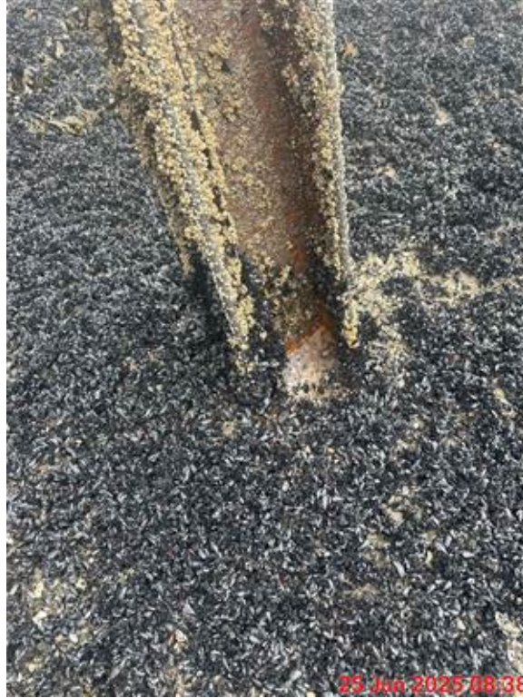
Photograph 39: Leg of North Dolphin. View Down. 6/25/2025.
