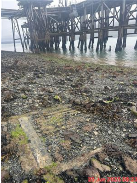
Photograph 29: Concrete vault near HFT Dock. View Northwest. 6/25/2025.
