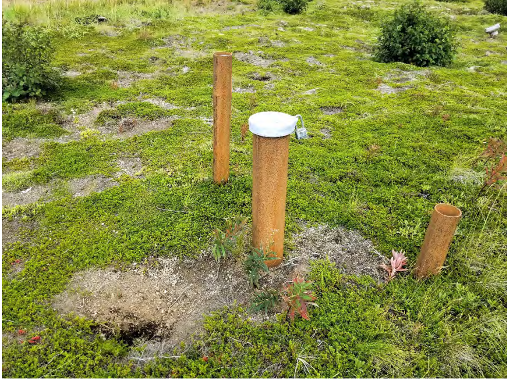
SS006 (FPC-066) - Monitoring Well MW-5 is secure and in good working condition.
