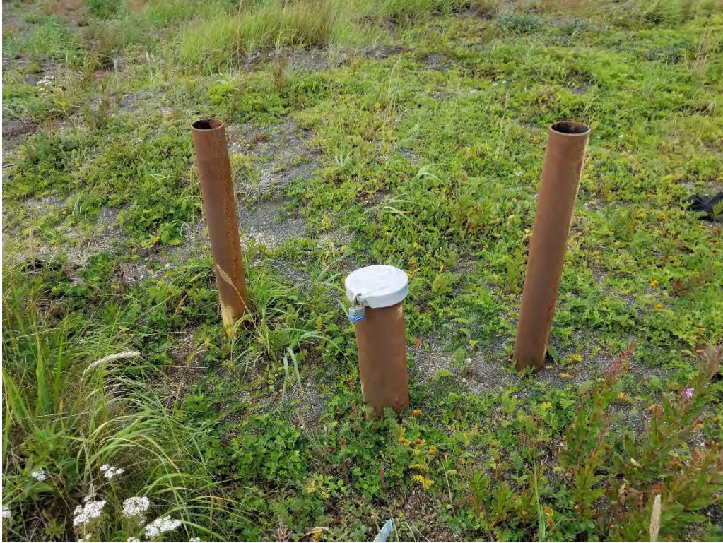
SS06(FPC-215) - Monitoring Well MW-8 is secure and in good working condition.
