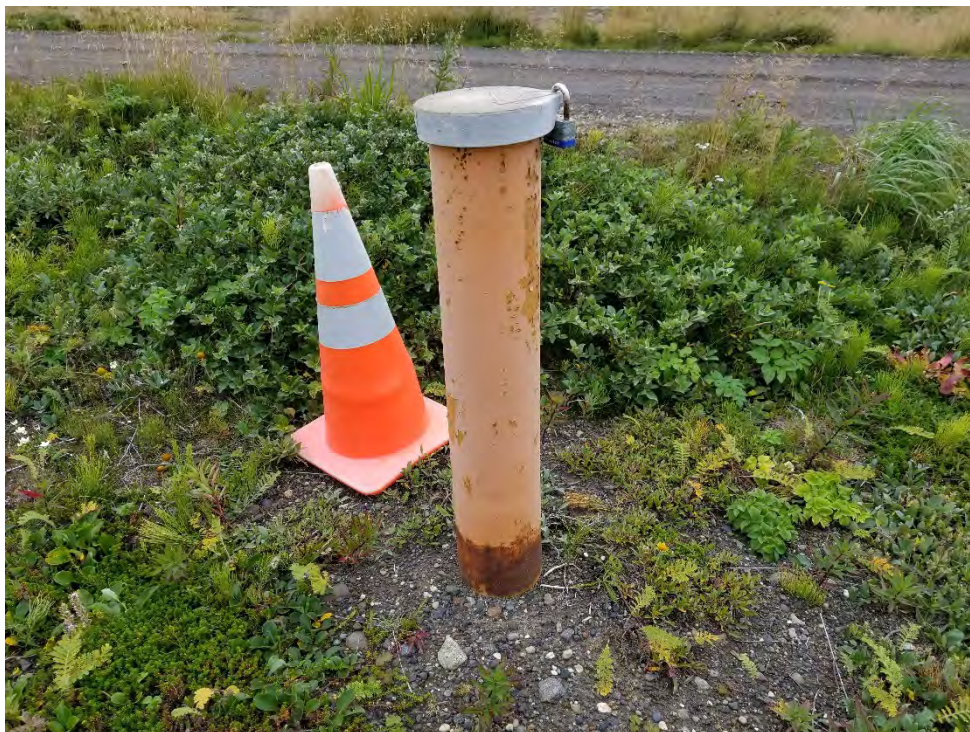
WP002 - Monitoring Well BLO-MW-07 is secure and in good working condition.
