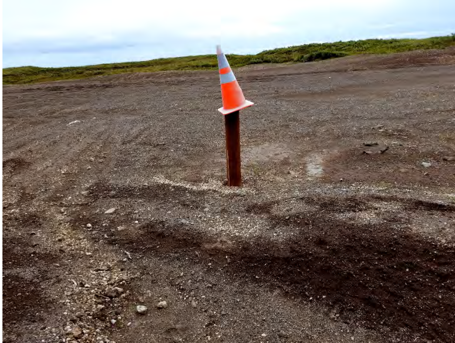
WP002 - Monitoring Well BLO-MW-05 is secure and in good working condition.
