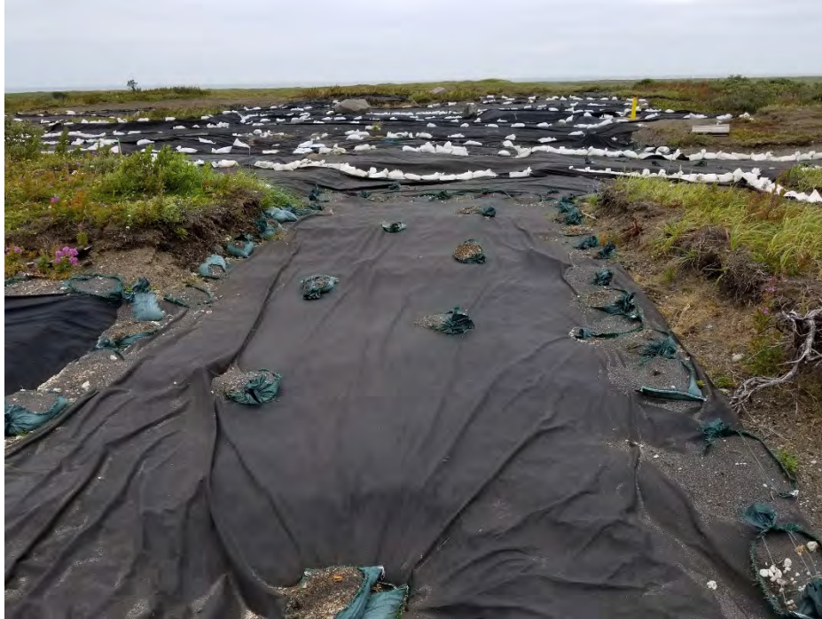
LF007 - General site condition looking west. Note Monitoring Well MW-10 in the background (right). Geo-fabric held in place by sandbags covers most of the site. In the foreground the green sandbags are more weathered than the white sandbags in the background, suggesting this cover consists of different aged materials.
