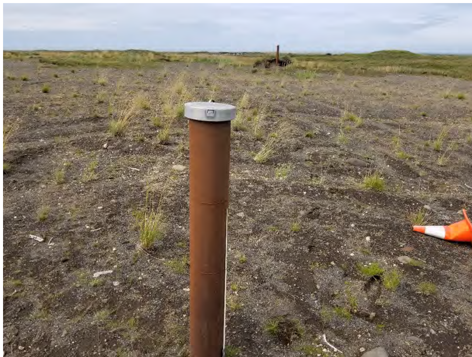
Ground Water Monitoring - Well GLO-MW-04 is secure and in good working condition.
