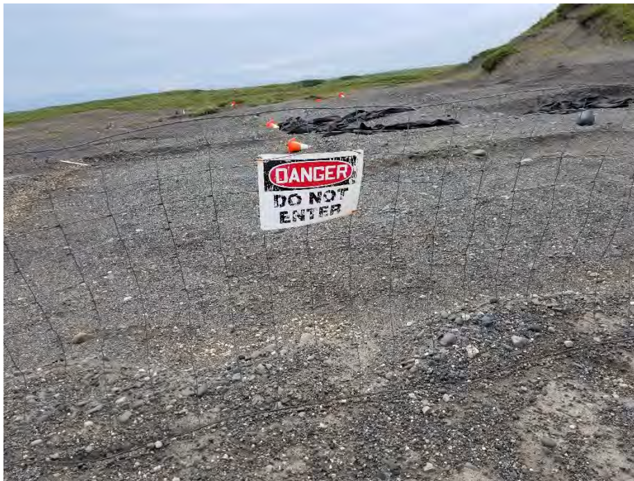
OT001 - Partial fence on the northern boundary of the Soil Removal Areas (and former antenna pads). Note the excavations beyond the fence and the Danger sign attached to the fence.
