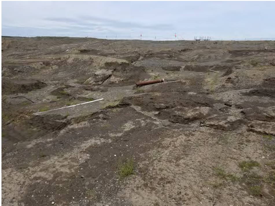
OT001 - A view of the Soil Removal Areas looking back towards the partial fence. Much of this area remains unvegetated with numerous open excavations and channels of erosion. Note in the foreground Monitoring Well PG1-MW-01, which is no longer functioning.
