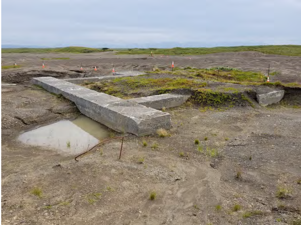
OT001 - A view south looking across a former antenna pad from within the Soil Removal Areas.
