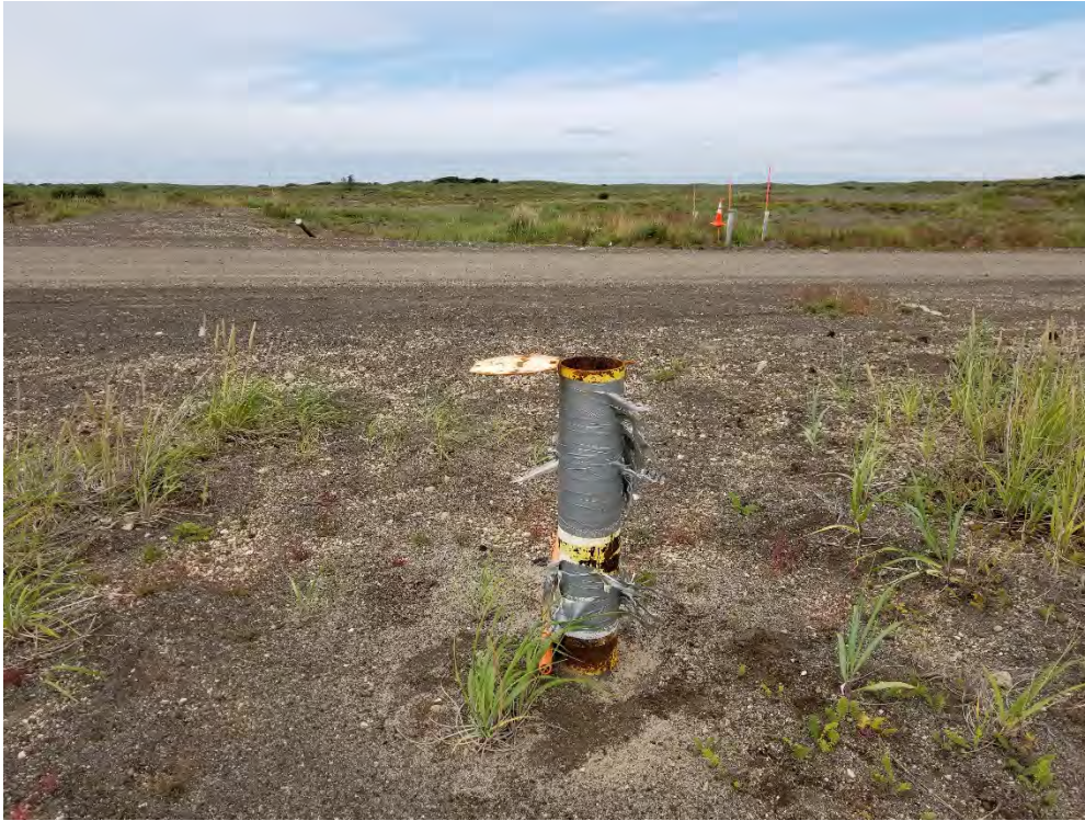
SS006 (FPC-215) - Unlabeled Monitoring Well within at the approximate location of a proposed new Monitoring Well (2016-2017 GW Monitoring Work Plan), south of the road. Although the protective casing is unsecure, the expansion plug is locked, and the well is in good working condition.
