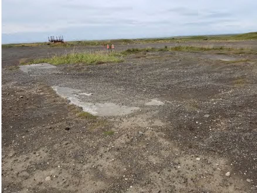
OT001 - Remnant concrete foundation for the Former Composite Building, looking southeast. Much of this area remains unvegetated and as exposed soil. There are several monitoring wells found around the former Port Heiden LRRS, most of which are not labeled. On the far edge of the concrete pad, flanked by bollards with traffic cones is the Monitoring Well UST-MW-02, which is secure and in good condition.
