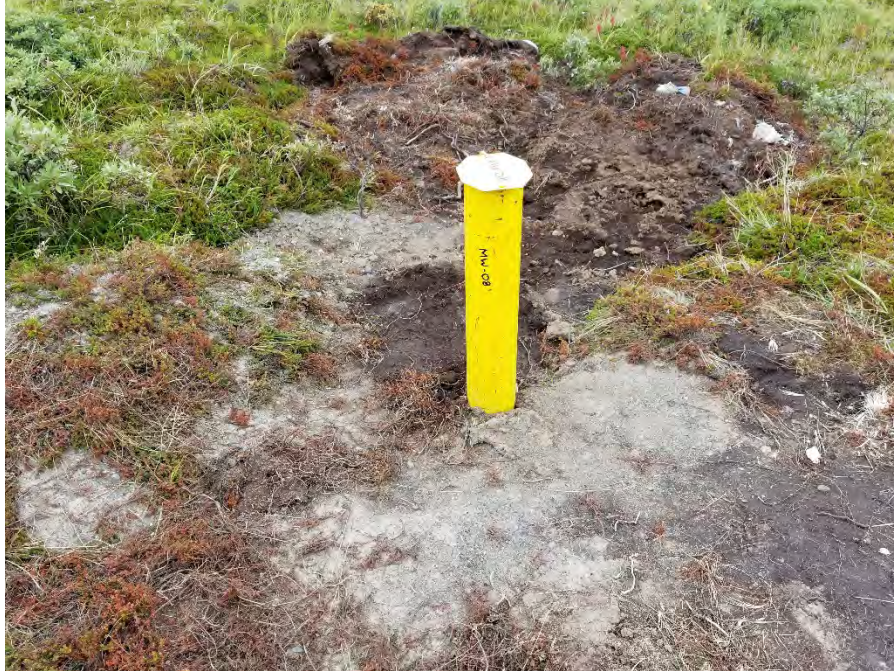
LF007 - Monitoring Well MW-08 is secure and in good working condition. The well appears to have been recently installed based on its new condition and the recent disturbance around it.
