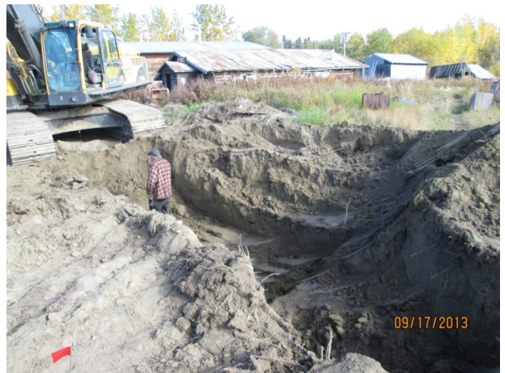
6) Starting Excavation 1 at southern half of site, facing northeast. September 17, 2013.
