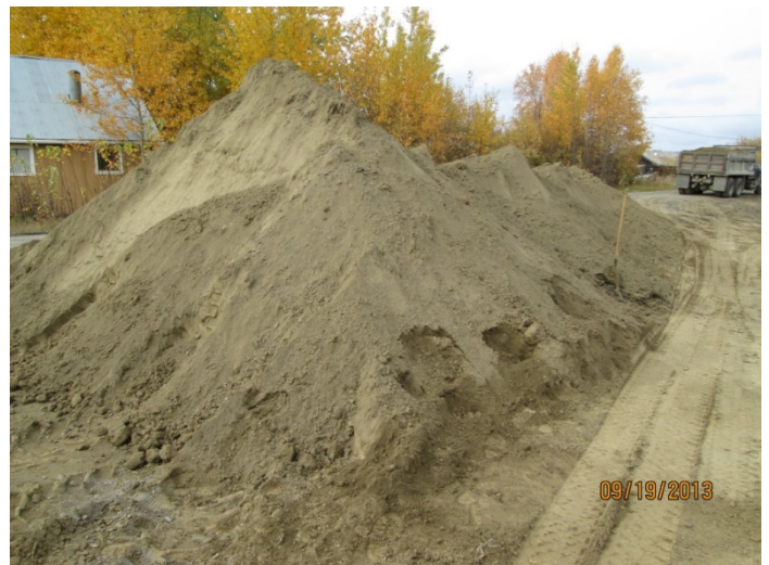
18) Stockpile of clean soil from Excavation 1, facing north. September 19, 2013.
