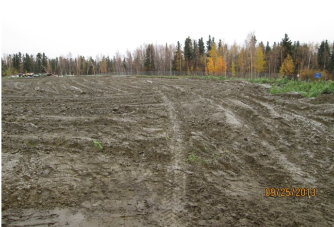
26) Completed landfarm. September 25, 2013.
