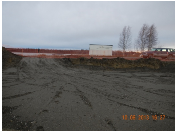
34) Excavation 1, facing south. October 8, 2013.
