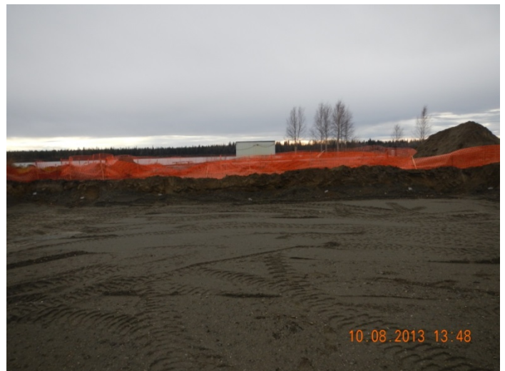
30) Excavation 2, facing south. October 8, 2013.
