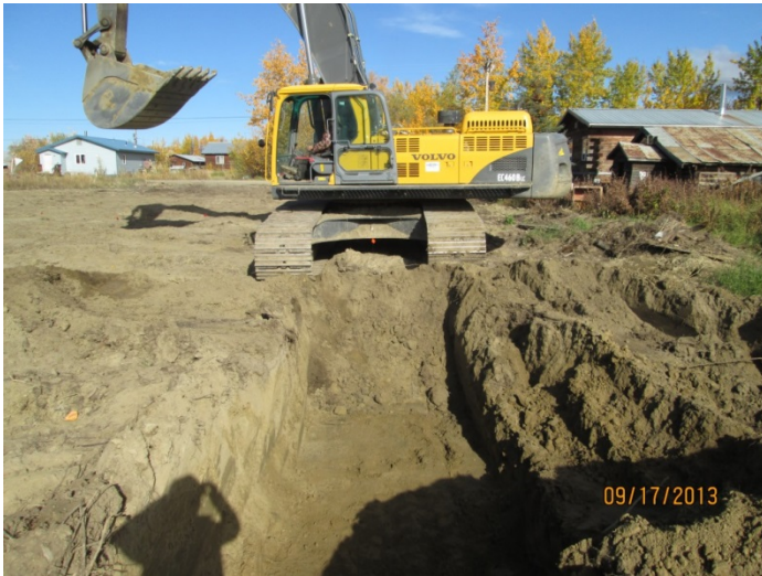
7) Start of Excavation 1, facing north. September 17, 2013.
