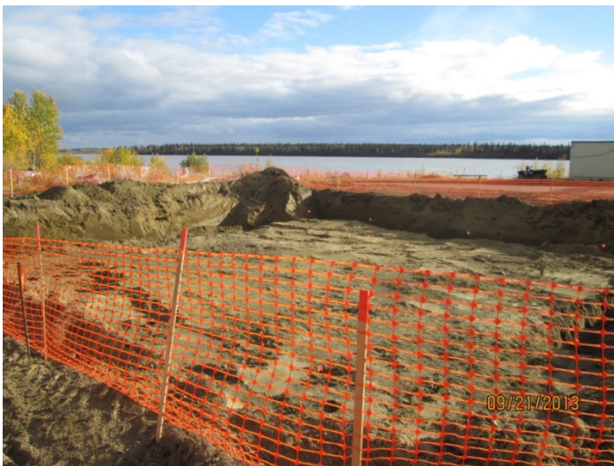
21) Excavation 1, facing southeast. September 21, 2013.
