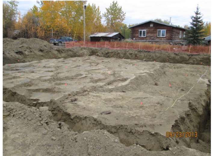
23) Excavation 2, facing northeast. September 23, 2013.
