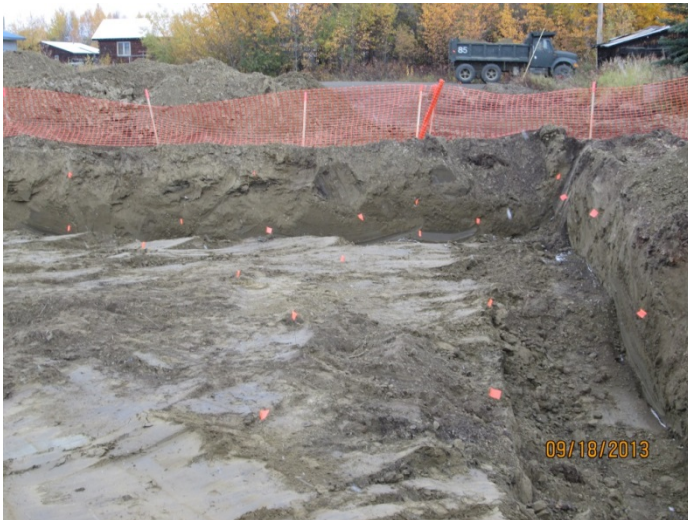
13) Northeast corner of Excavation 1, facing north. September 18, 2013.
