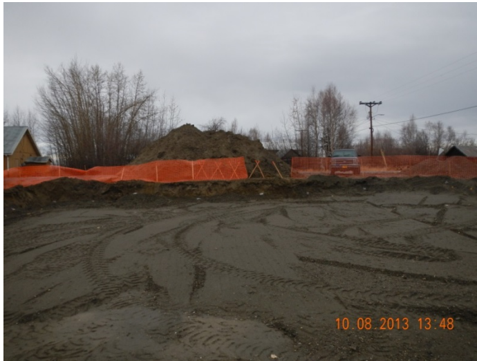
31) Excavation 2, facing west. Clean stockpile in background. October 8, 2013.
