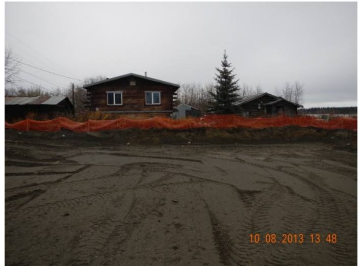
28) Excavation 2, facing east. October 8, 2013.
