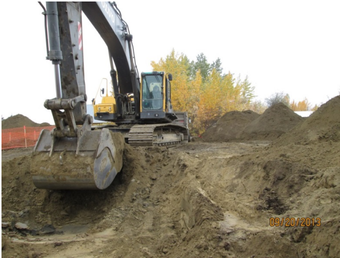
19) Starting Excavation 2, facing southwest. September 20, 2013.
