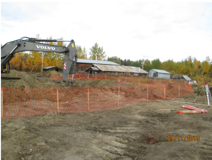
9) Plastic fencing placed around Excavation 1, facing northeast. September 17, 2013.
