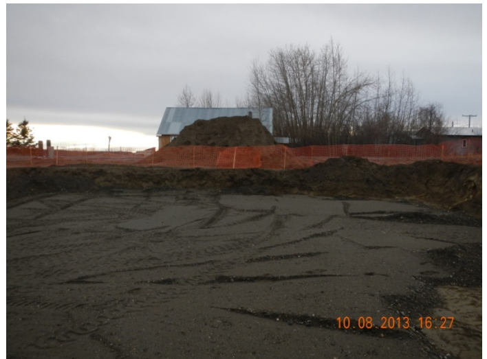
35) Excavation 1, facing west. Clean soil stockpile in background. October 8, 2013.
