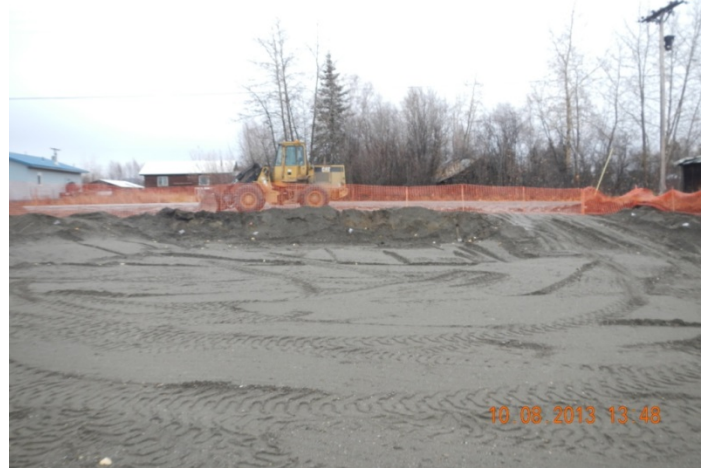
29) Excavation 2, facing north. October 8, 2013.
