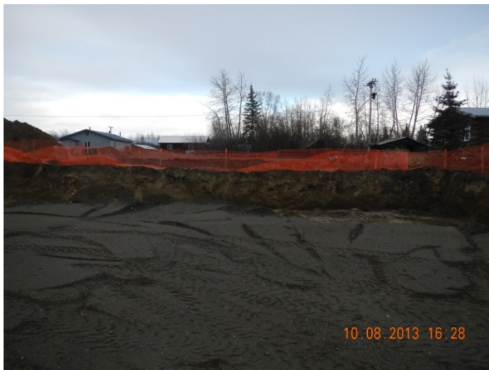
33) Excavation 1, facing north. October 8, 2013.
