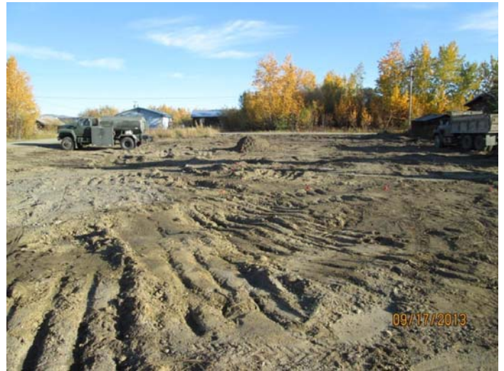
4) September 17, 2013. Site following grubbing, facing north. September 17, 2013.
