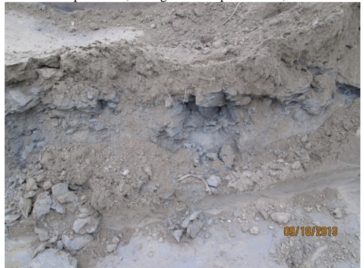
11) Dark gray silt with hydrocarbon odor in southwest portion of Excavation 1, facing south. September 18, 2013.
