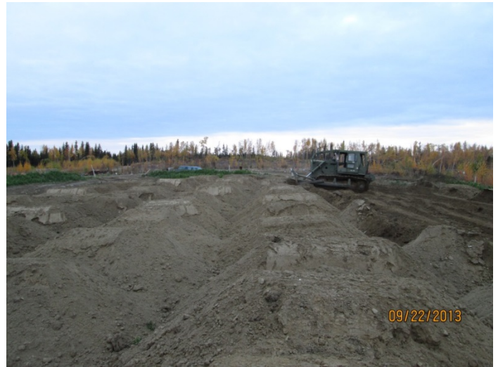
22) Dozer spreading out dumped contaminated soil in landfarm. September 22, 2013.
