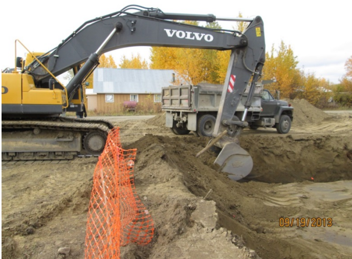
14) Pipe unearthed in southwest corner of Excavation 1, facing west. September 19, 2013.
