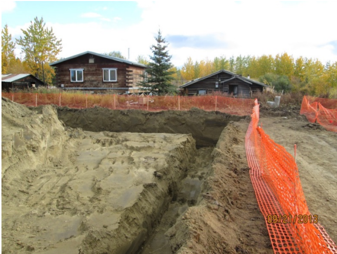
20) Southeast corner of Excavation 2, facing east. September 21, 2013.
