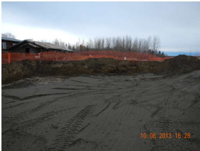
32) Excavation 1, facing east. October 8, 2013.
