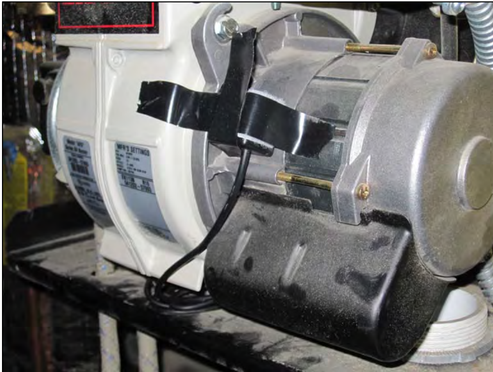
Example of a Runtime DataWatcher motor sensor being installed to monitor an oil boiler.
