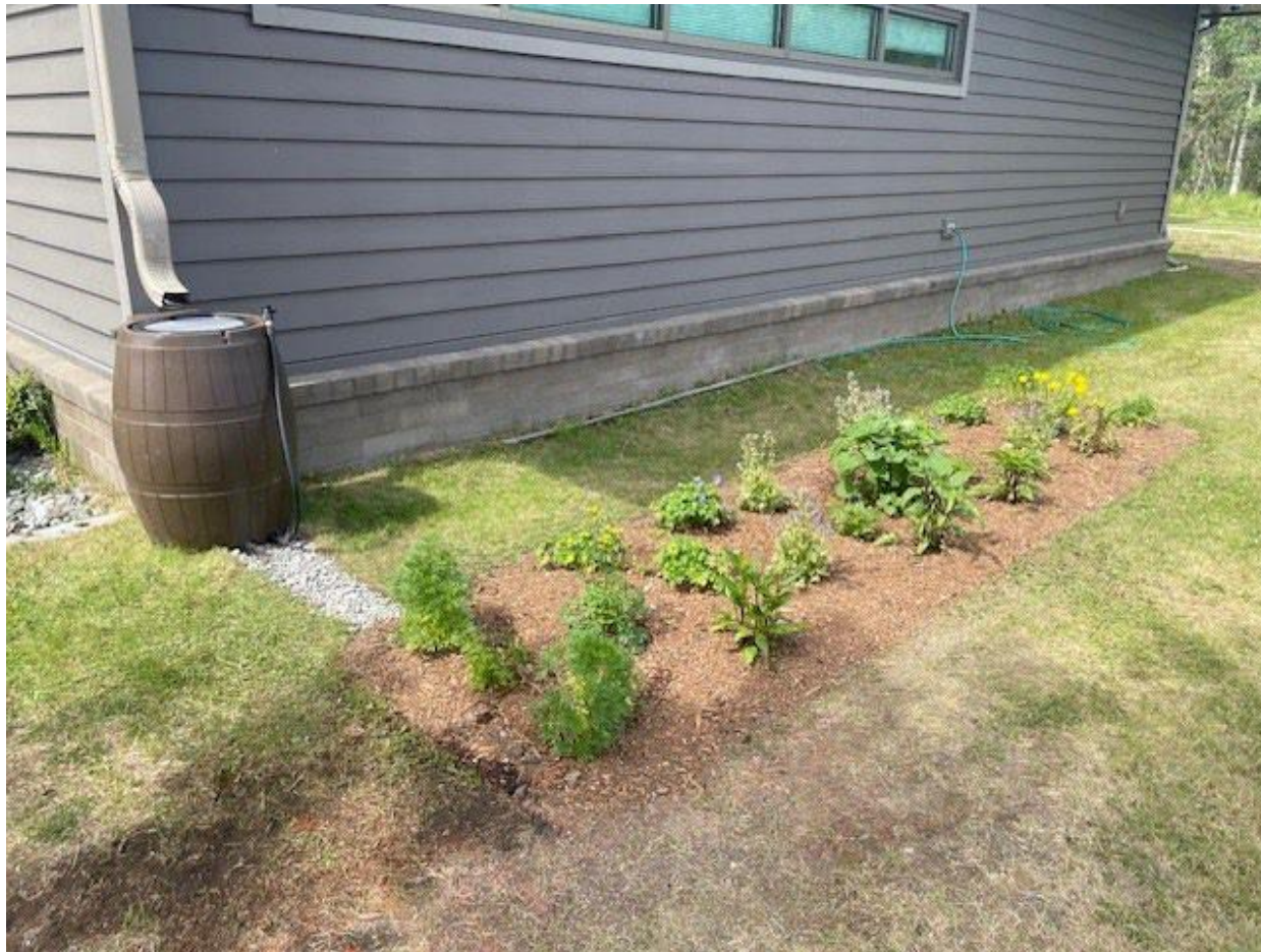
Rain Garden & Rain Barrel Installed
