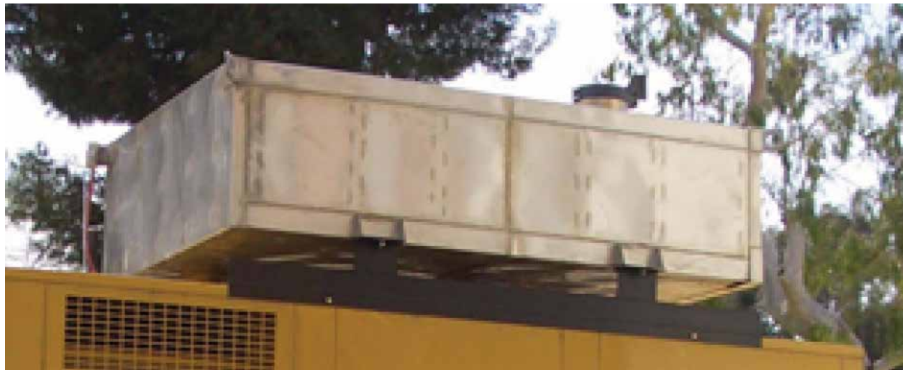
Figure 3.1 – Stationary Installation of a Cat DPF Reactor on a Generator Set
