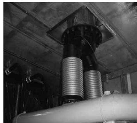
Figure 4.7 – Exhaust Bellows Connection
