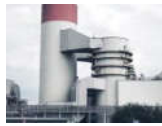
RYBNIK, POLAND Wet limestone FGD Customer: Elektroenergia Rybnik Capacity: 4 × 200 MWel, 2 × 1,320,000 m 3 /h [stp, wet] Fuel: Hard coal Start-up: 2008
