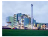
TA LAUTA, GERMANY Wet limestone FGD Customer: RWE Power Capacity: 2 × 1,100 MWel, 2 × 4,850,000 m 3 /h [stp, wet] Fuel: Lignite Start-up: 2011
