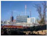
LINZ 04-05, AUSTRIA SCR DeNOx Customer: VA STAHL Capacity: 2 × 150,000 m 3 /h [stp, wet] Fuel: Blast furnace gas, coke oven gas Start-up: 2004-2005
