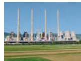
TURCENI, ROMANIA Wet limestone FGD Customer: S.C. Complexul Energetic Turceni S.A. Capacity: 4 × 330 MWel, 4 × 1,723,000 m 3 /h [stp, wet] Fuel: Lignite Start-up: 2011
