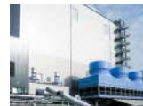
GLÜCKSTADT, GERMANY Dry FGC (TurboSorp) Customer: HKWG Glückstadt Capacity: 160,000 m 3 /h [stp, wet] Fuel: RDF, sludge, coal Start-up: 2009
