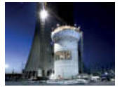
LÜNEN, GERMANY Wet limestone FGD Customer: Trianel Capacity: 1 × 800 MWel, 1,965,000 m 3 /h [stp, wet] Fuel: Hard coal Start-up: 2012
