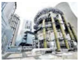
NEURATH F/G, GERMANY Wet limestone FGD Customer: RWE Power Capacity: 2 × 1,100 MWel, 2 × 4,850,000 m 3 /h [stp, wet] Fuel: Lignite Start-up: 2011
