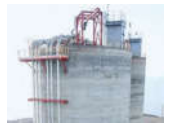
GUACOLDA, CHILE Turbo-CDS and SCR plant Customer: Empresa Electrica Guacolda Capacity: 3 × 140 MW, 3 × 560,000 m 3 /h [std, wet] Fuel: Coal Start-up: 2015-2016
