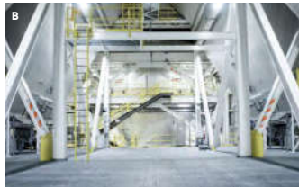
A Cleco, USA B Hoppers for the pulse jet fabric filter – Big Stone – Otter Tail
