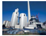
KARLSRUHE, GERMANY Wet limestone FGD Customer: EnBW Capacity: 910 MWel, 2,500,000 m 3 /h [stp, wet] Fuel: Hard coal Start-up: 2011
