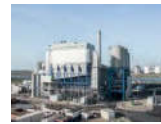
MOERDIJK, NETHERLANDS TurboSorp PJFF, ESP and SCR/DeNOx Customer: BMC Moerdijk Capacity: 250,000 m 3 /h [stp, wet] Fuel: Poultry litter Start-up: 2008
