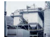
LUKE, MD, USA Pulse Jet Fabric Filter (PJFF) Customer: New Page Capacity: 1 × 179900 and 1 × 349,800 m 3 /h [stp, wet] Fuel: Eastern bituminous coal Start-up: 2007
