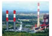
MELLACH, AUSTRIA SCR DeNOx Customer: Siemens, Verbund ATP Capacity: 2 × 400 MWel, 2 × 2,100,000 m 3 /h [stp, wet] Fuel: Natural gas Start-up: 2011
