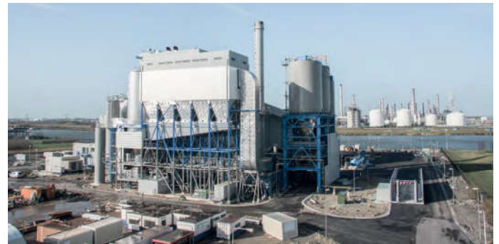
TurboSorp, Fabric Filter, SCR, Moerdijk, Netherlands
