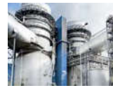
TUSIMICE II, CZECH REPUBLIC Wet limestone FGD Customer: CEZ Capacity: 4 × 200 MWel, 2 × 1,780,000 m 3 /h [stp, wet] Fuel: Lignite Start-up: 2009/2010
