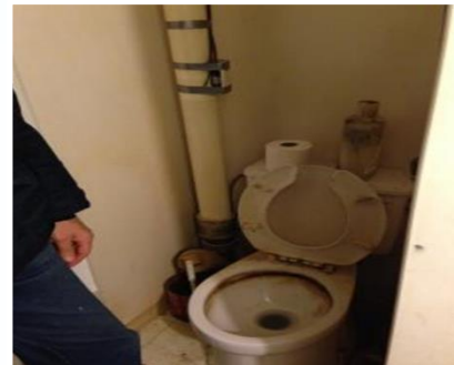
Toilet flushing with used sink water
