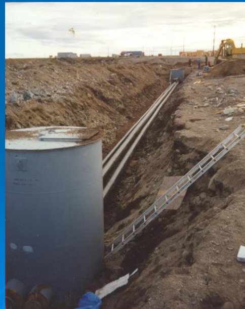
Buried water and sewer system in Iqaluit
